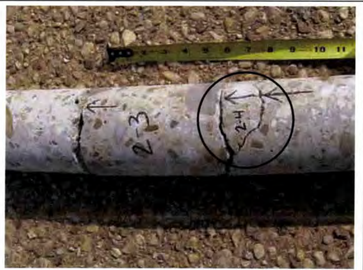
Photo 7: Core 2, Segments 3 and 4 - Chip in Segment 4.
