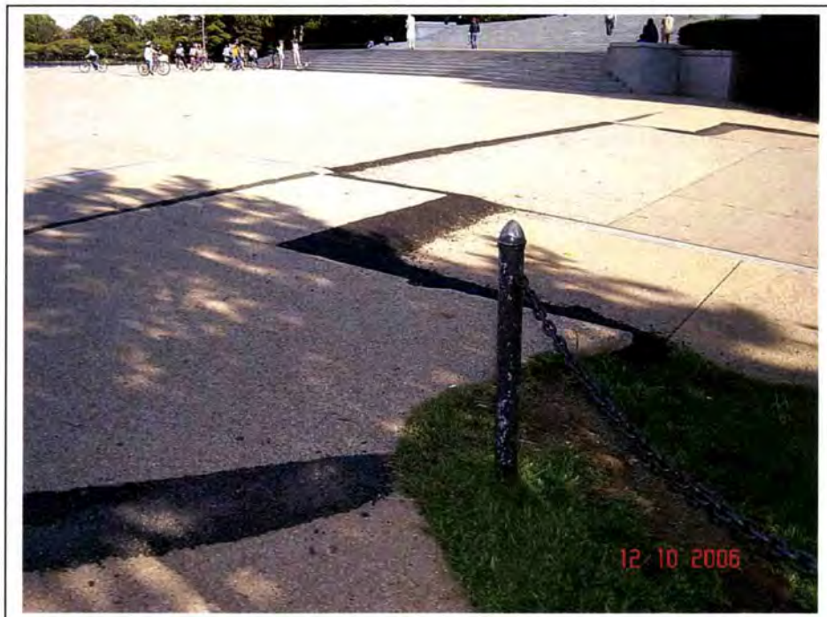
Figure 5. Asphalt Patches on North Plaza and Circular Roadway Interface (10-12-06). Note "bulge" in grassy area suggesting the presence of a grade beam on piles.
