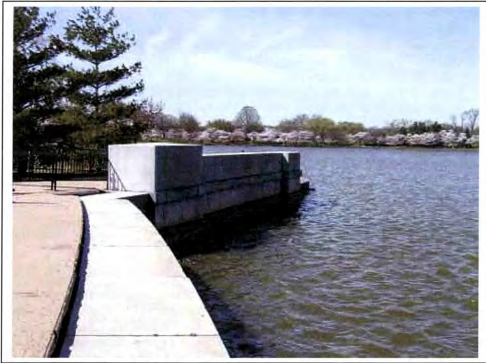
Figure 1. View Standing on the Ashlar Seawall Looking West (3-29-07)
