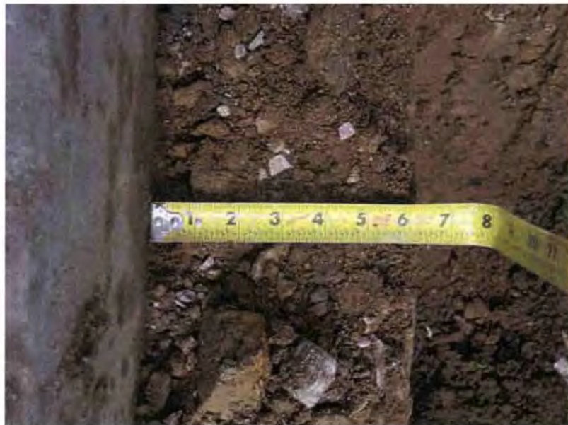
PHOTO 19 – Grade beam beyond slab joint
