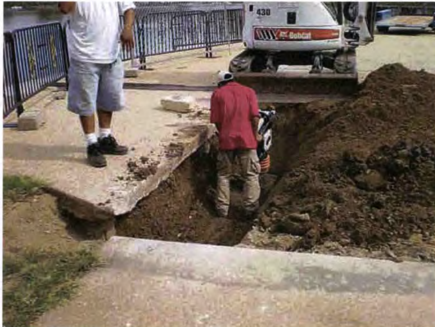
PHOTO 13 – Backfilling and compaction
