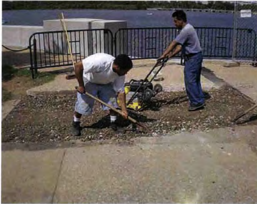
PHOTO 14 – Backfilling and compaction of #57 stone
