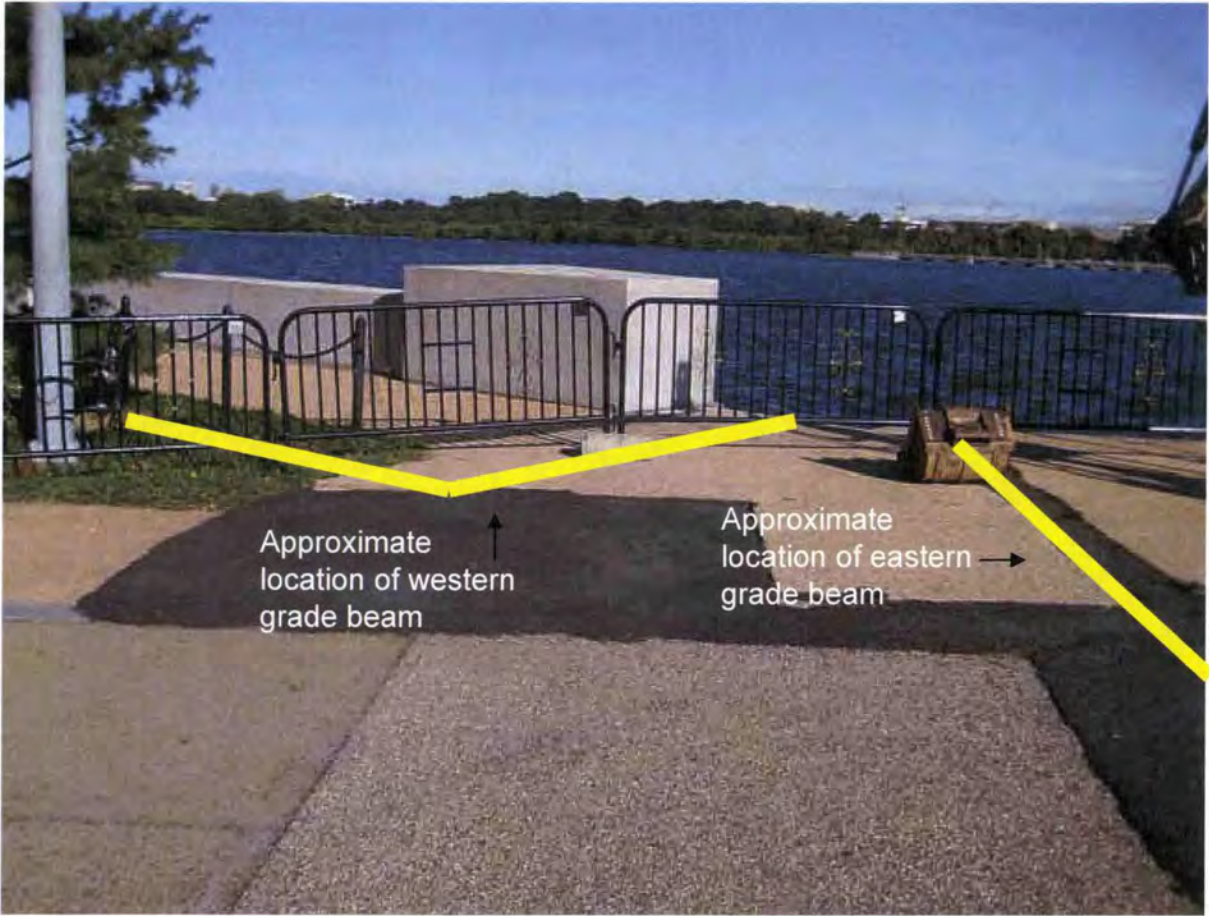
PHOTO 1 – Approximate locations of grade beams
