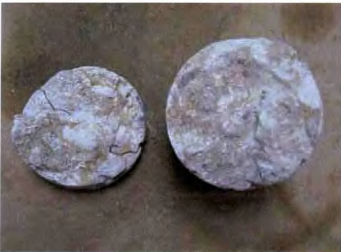
Photo 18: Core 4, Segment 1 - Cracking within Segment 1 shows evidence of efflorescence (white staining).
