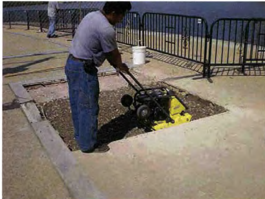
PHOTO 21 – Backfilling and compaction of #57 stone
