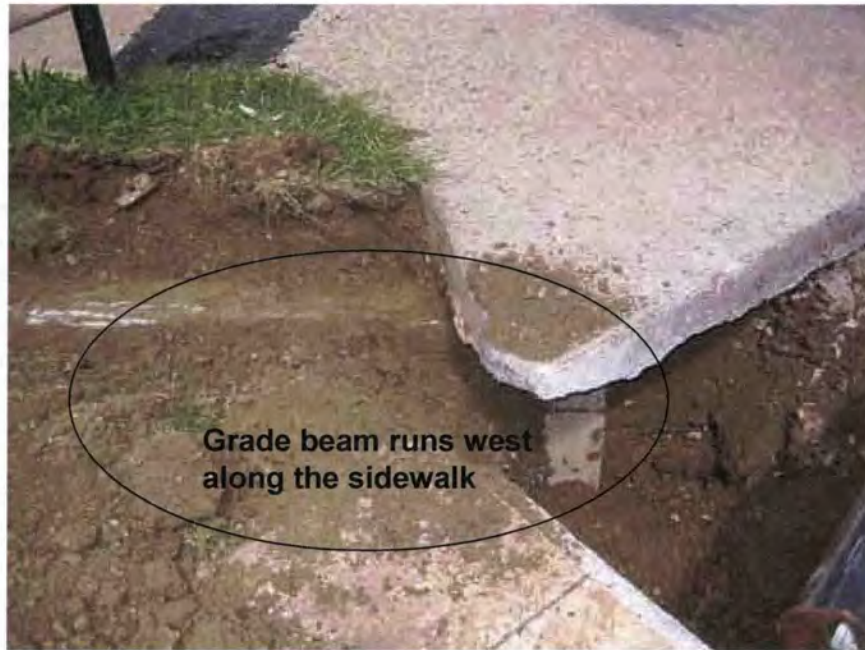
PHOTO 11 – Location of western grade beam
