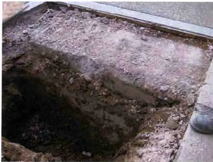
PHOTO 16 – Test Pit #2 grade beam
