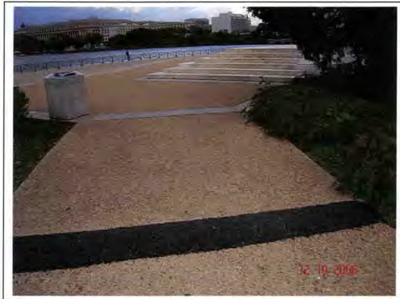
Figure 8. West Terrace Walkway Looking Toward Main Stairs (10-12-06)
