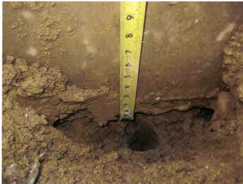
PHOTO 3 – Void below eastern grade beam
