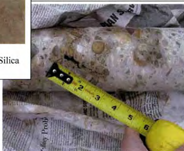
Photo 6: Core 1, Segment 11 - Entrapped air in concrete.
