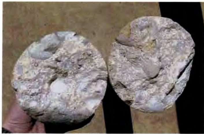
Photo 8: Core 2, Segments 3 and 4 - Evidence of efflorescence (white staining).
