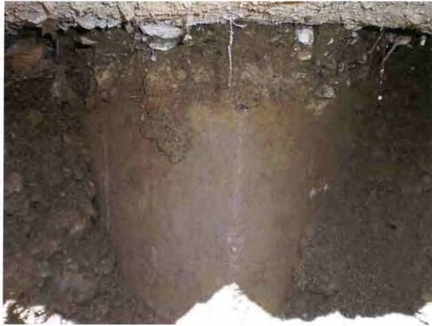
PHOTO 12 – Corner of western grade beam
