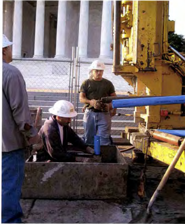
PHOTO 5: Installation of inclinometer casing
