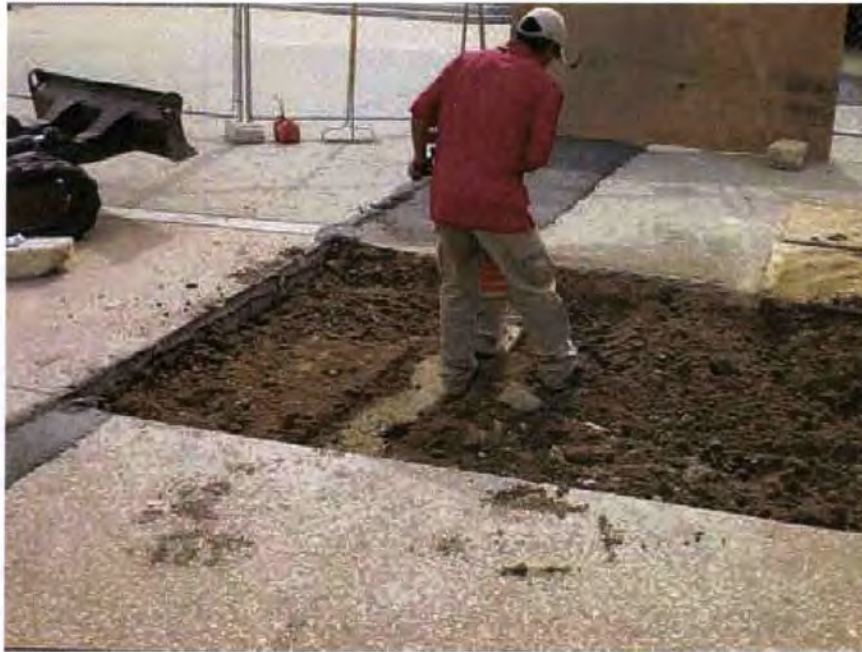
PHOTO 20 – Backfilling and compaction
