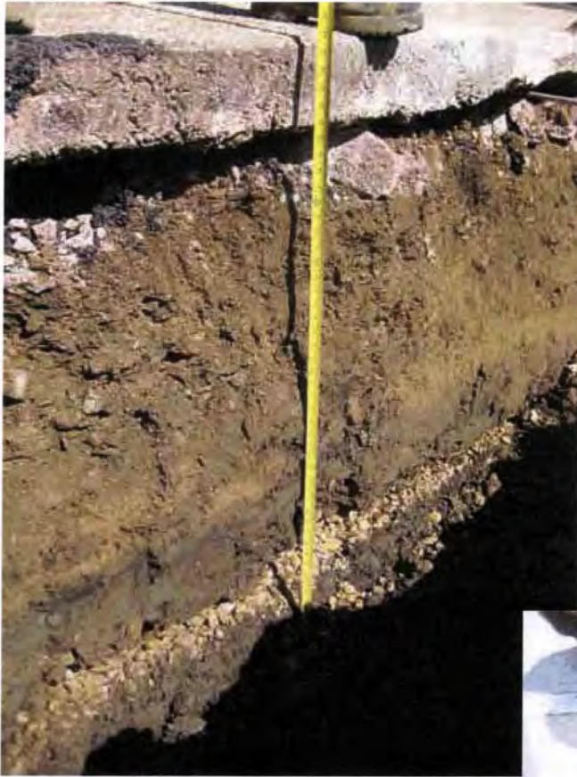
PHOTO 4 – Subgrade material. Note the 6" layer of rounded cobble
