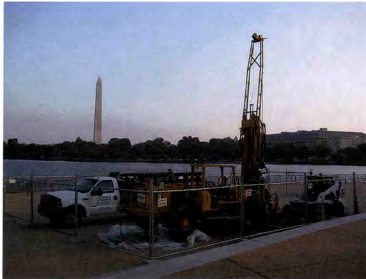
PHOTO 3: Connelly drill rig set up
