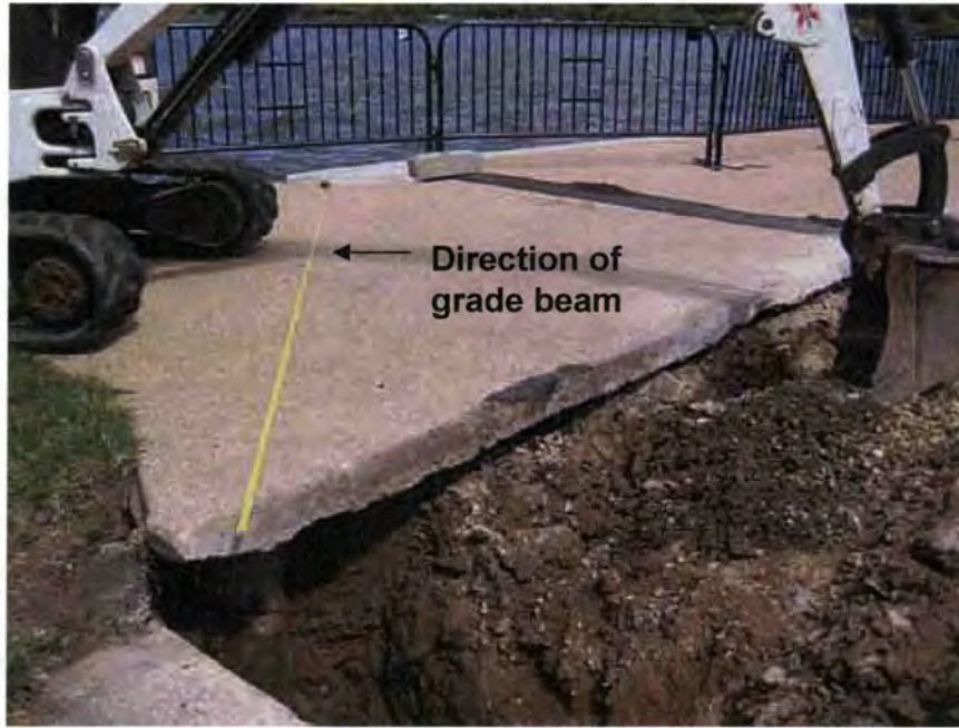
PHOTO 10 – Location of western grade beam
