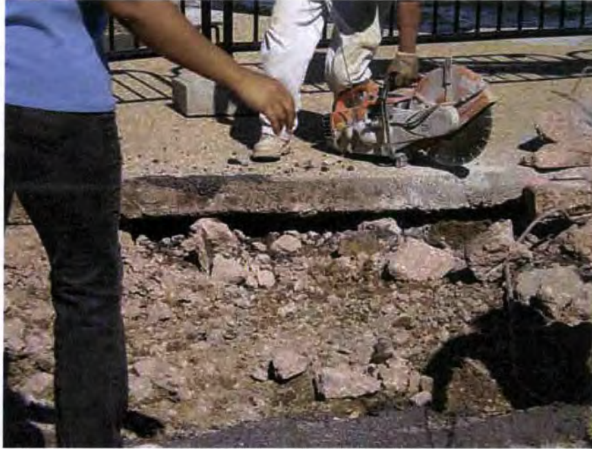
PHOTO 8 – 3 to 5" void below northern slab
