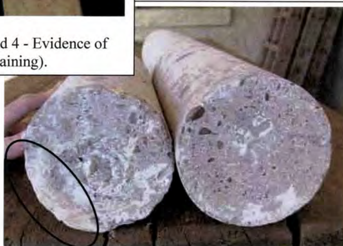
Photo 9: Core 2, Segments 4 and 5 - Smooth finish shows evidence of a joint. Silica gel forming in concrete.
