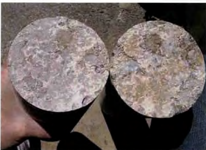
Photo 27: Core 5, Segments 6 and 7 - Cross section of joint shows evidence of efflorescence.
