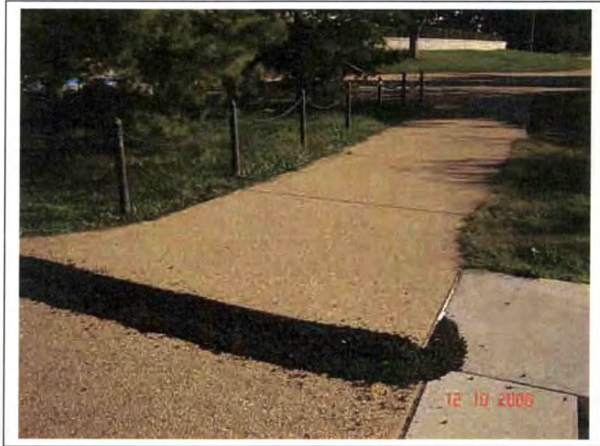
Figure 5. Asphalt Patch at Northwest Stairs (10-12-06)
