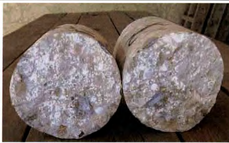
Photo 13: Core 3, Segments 1 and 2 - Cross section of break showing evidence of efflorescence (white staining).
