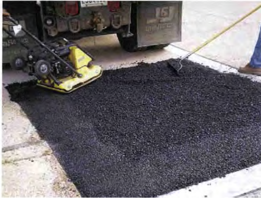
PHOTO 22 – Final asphalt layer
