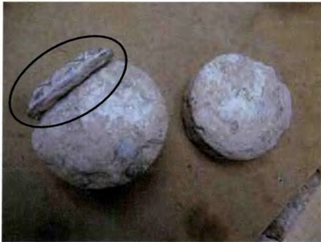
Photo 1: Core 1, Segments 3 and 4 - Cross section of break, showing reinforcing steel (not intact) and evidence of efflorescence (white staining).
