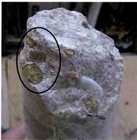
Photo 14: Core 3, Segment 3 - Dark rings around the aggregate show a potential for ASR.
