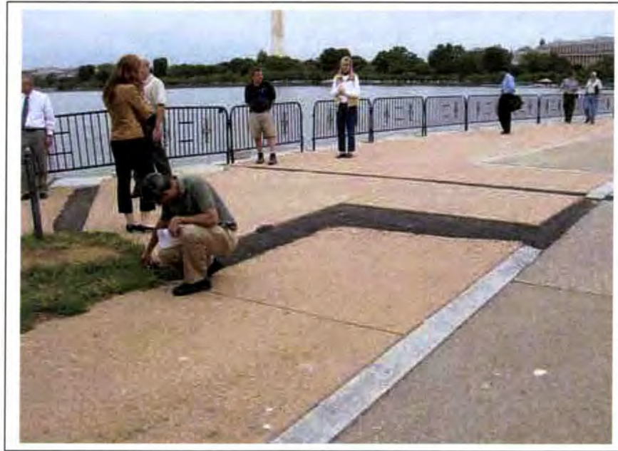
Figure 3. Asphalt Patches on North Plaza and Circular Roadway Interface (9-12-06)
