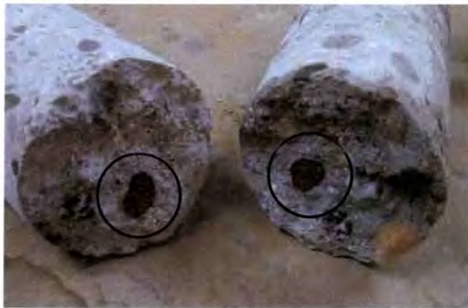
Photo 26: Core 5, Segments 1 and 2 - Cross section of break. Note that the aggregate fractured and that a ring appears around aggregate indicating potential ASR.
