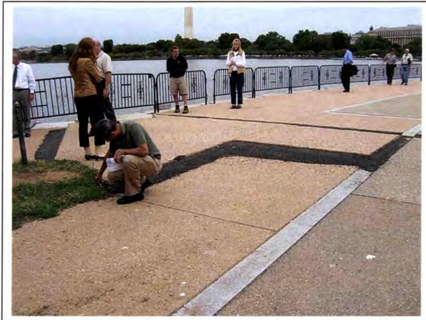
Figure 4. Asphalt Patches on North Plaza and Circular Roadway Interface (9-12-06)
