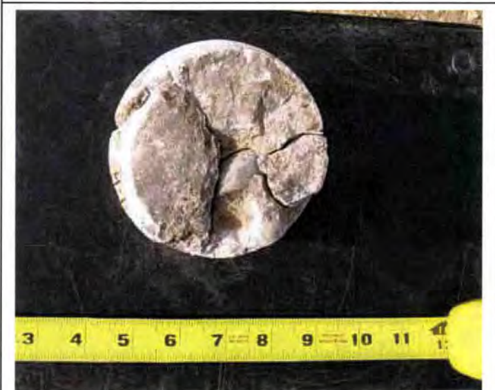
Photo 17: Core 4, Segment 1 - Top of core shows significant cracking.
