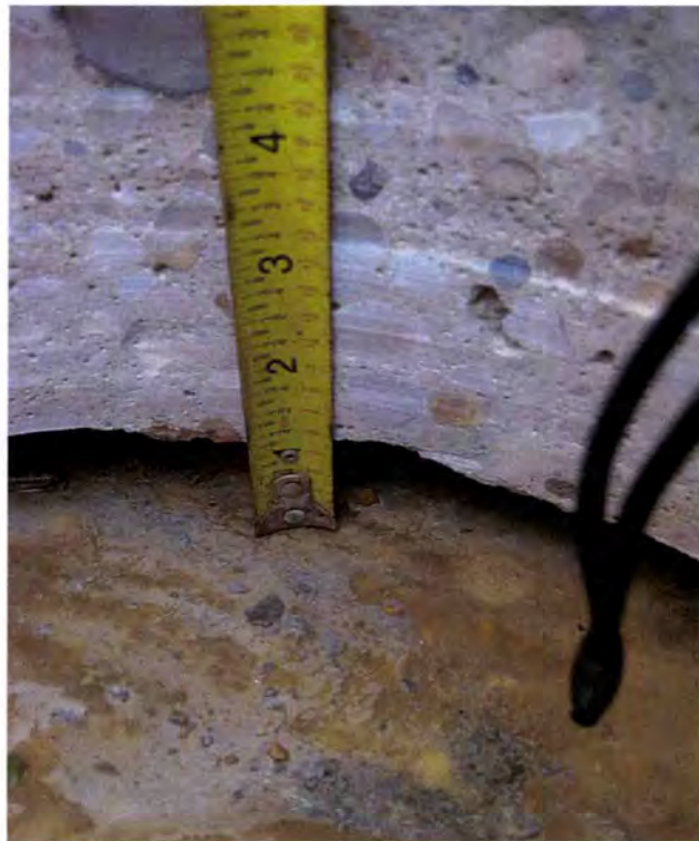
PHOTO 2: One-inch gap below plaza slab
