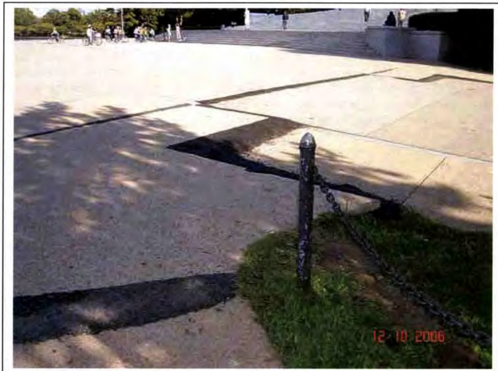
Figure 4. Asphalt Patches on North Plaza and Circular Roadway Interface (10-12-06). Note "bulge" in grassy area suggesting the presence of a grade beam on piles.
