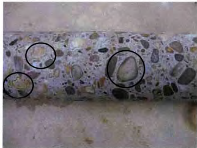
Photo 4: Core 1, Segment 10 - Dark rings around aggregate show a potential for ASR.
