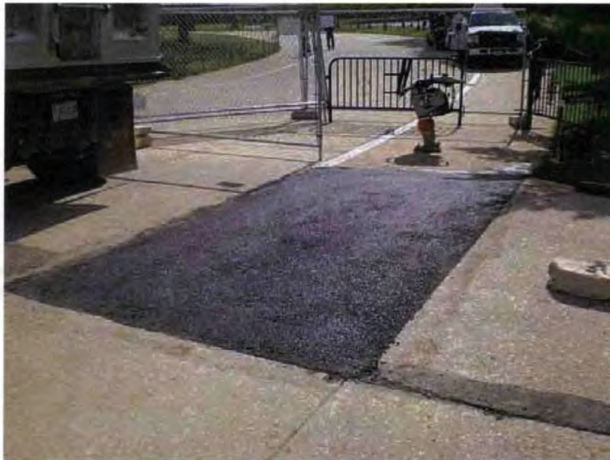
PHOTO 15 – Final asphalt layer
