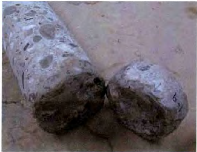
Photo 2: Core 1, Segments 8 and 9 - Cross section of joint.
