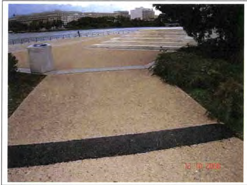
Figure 7. West Terrace Walkway Looking Toward Main Stairs (10-12-06)
