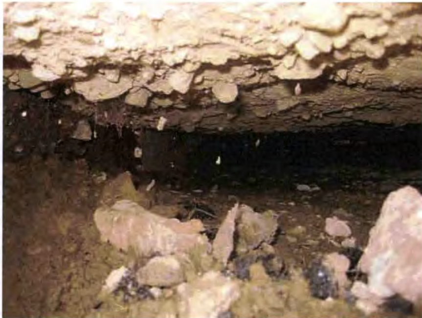
PHOTO 9 – 3 to 5" void below northern slab
