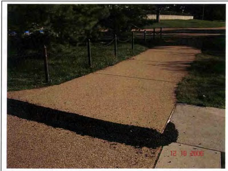
Figure 6. Asphalt Patch at Northwest Stairs (10-12-06)
