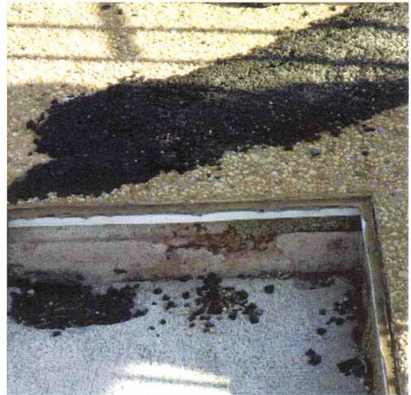
Photograph 3: Soil movement has caused the seawall to separate from the north plaza. The separation has created a tripping hazard.
