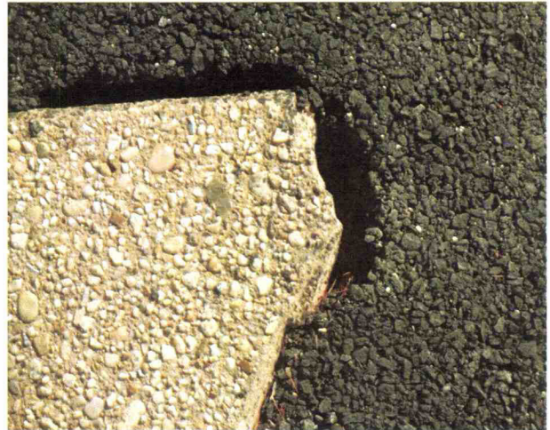
Photograph 1: Continued soil movement has resulted in additional separation at previously repaired areas.
