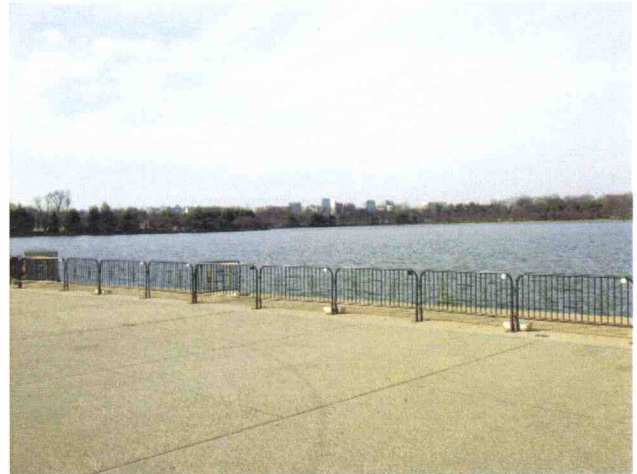
Photograph 6: Separation between the north plaza and the seawall has created a tripping hazard. To protect visitors from this hazard, the NPS has erected a temporary metal fence along the length of the seawall.
