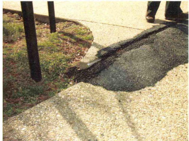
Photograph 7: The asphalt patching used to cover separation of pavement in the transition areas (shown above) is not consistent with the concrete aggregate that is used in the walkways and the plaza.
