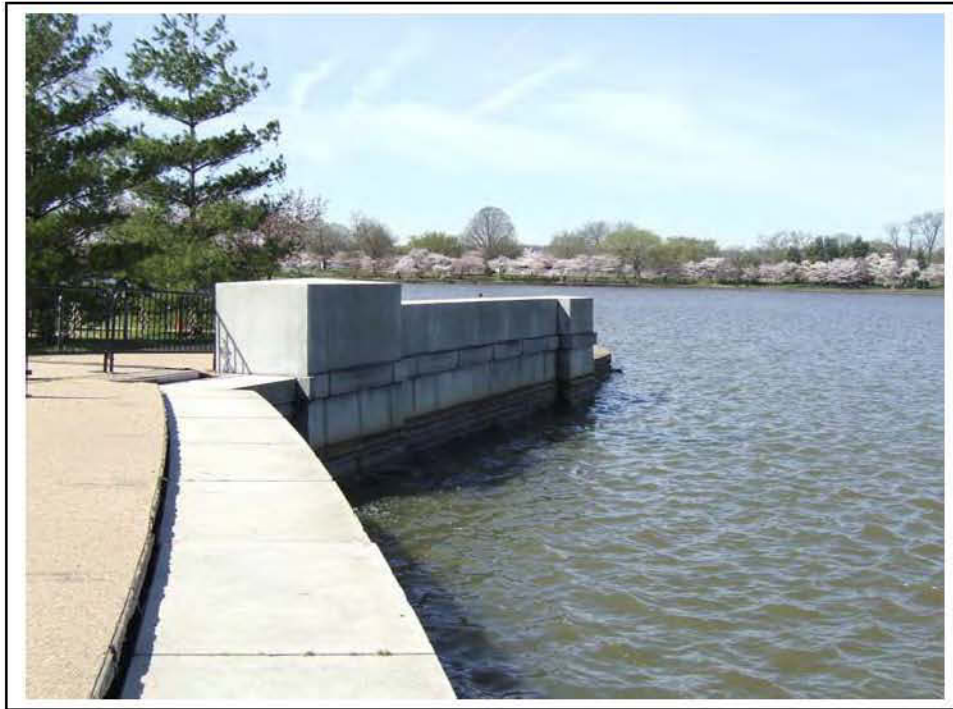
Figure 2. View Standing on the Ashlar Seawall Looking West (3-29-07)
