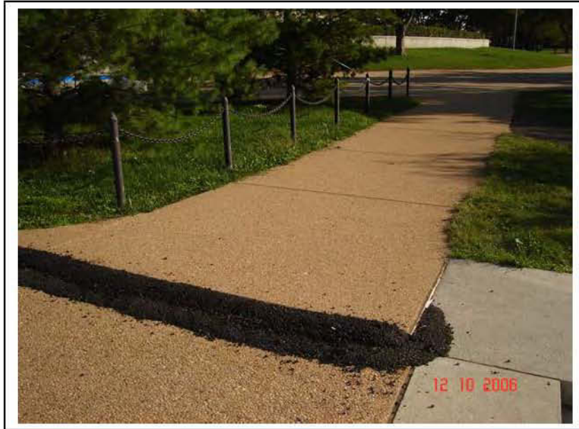
Figure 6. Asphalt Patch at Northwest Stairs (10-12-06)
