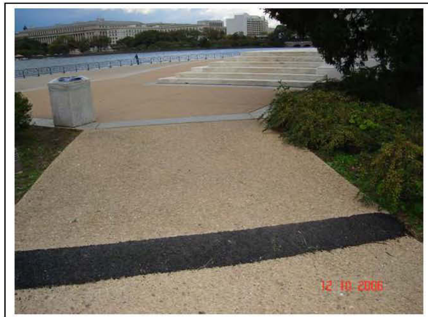
Figure 8. West Terrace Walkway Looking Toward Main Stairs (10-12-06)
