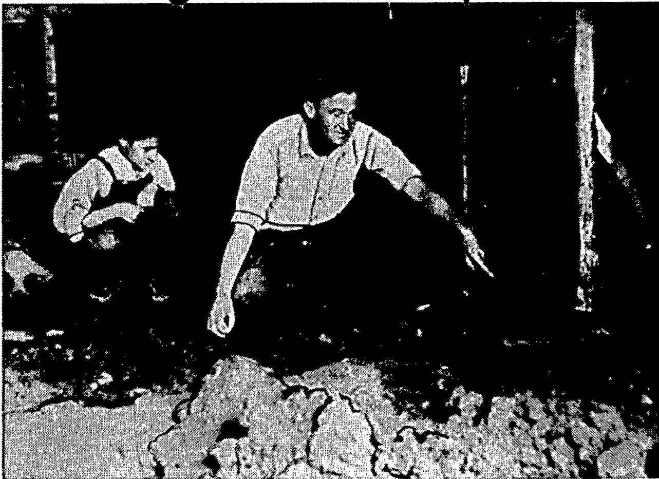
INTERIOR OF THE HAUPTMANN GARAGE. HERE THE KIDNAPER HAD BURIED $13,760.00 OF THE RANSOM MONEY.
