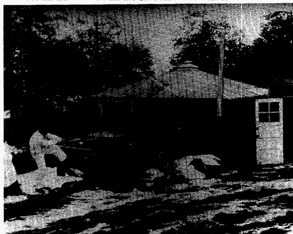
Figure 45. Early method of handling radioactive sources at Los Alamos.
