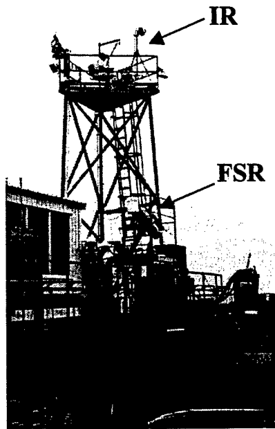
Figure 3. Bridge Showing FSR on Scaffold and IR on Tower
