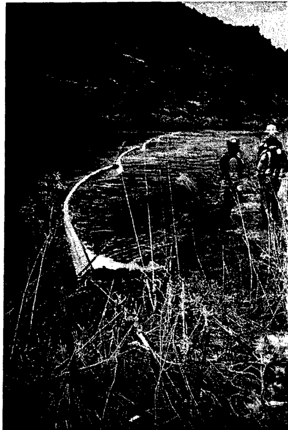
Figure 12. Cascade Booming of a Narrow River
