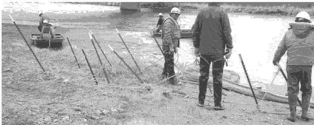
Figure 8-9. Multiple booms being anchored (DOWCAR, 1997).
