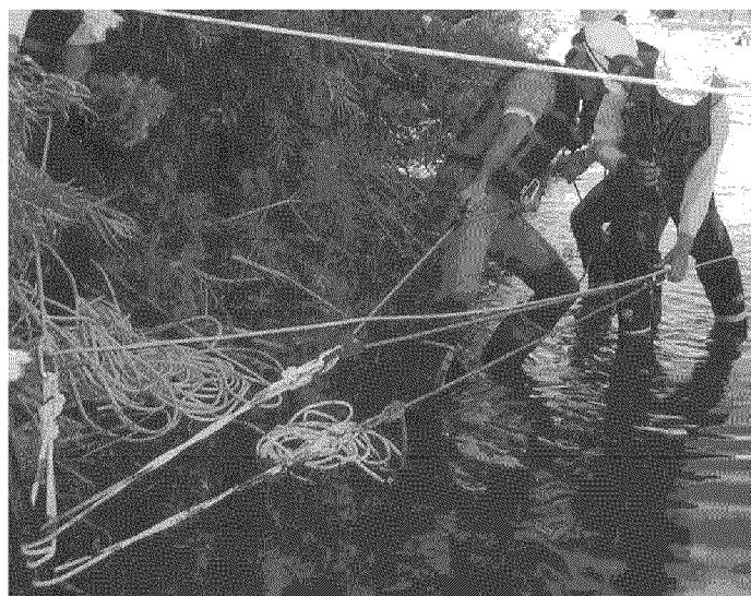
Figure 9-2. Ascenders in use for tightening lines (DOWCAR, 1997).
