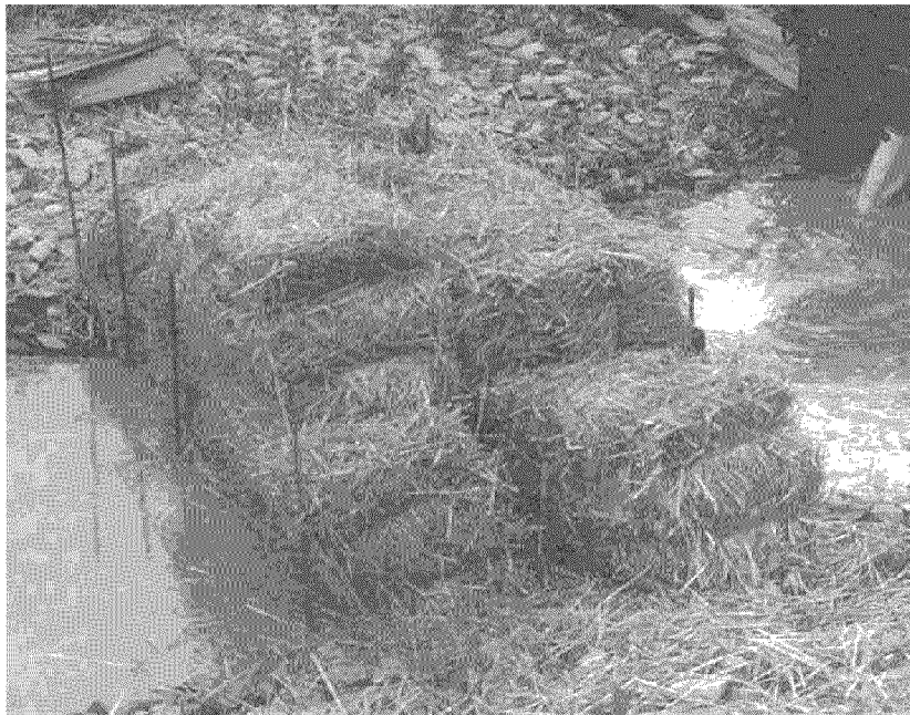
Figure 4-29. Hay filter barrier.
