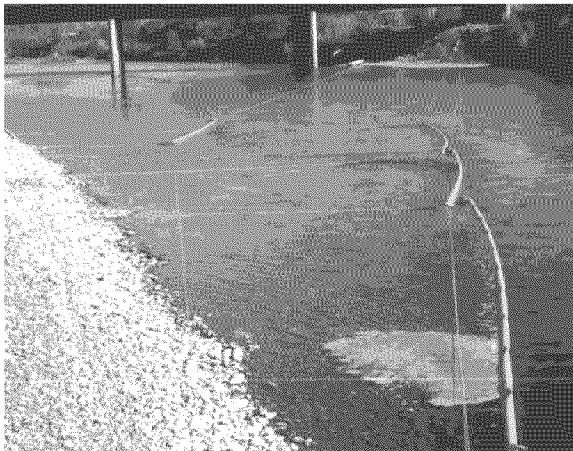
Fourth boom is deployed.
