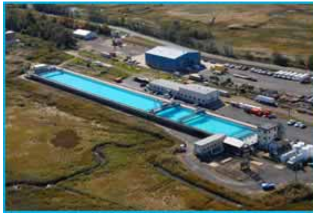
Figure 1. OHMSETT test facility.
