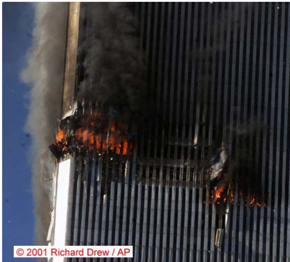
Figure 7–74. Impact damage to the northeast corner of the exterior wall of WTC 2.
