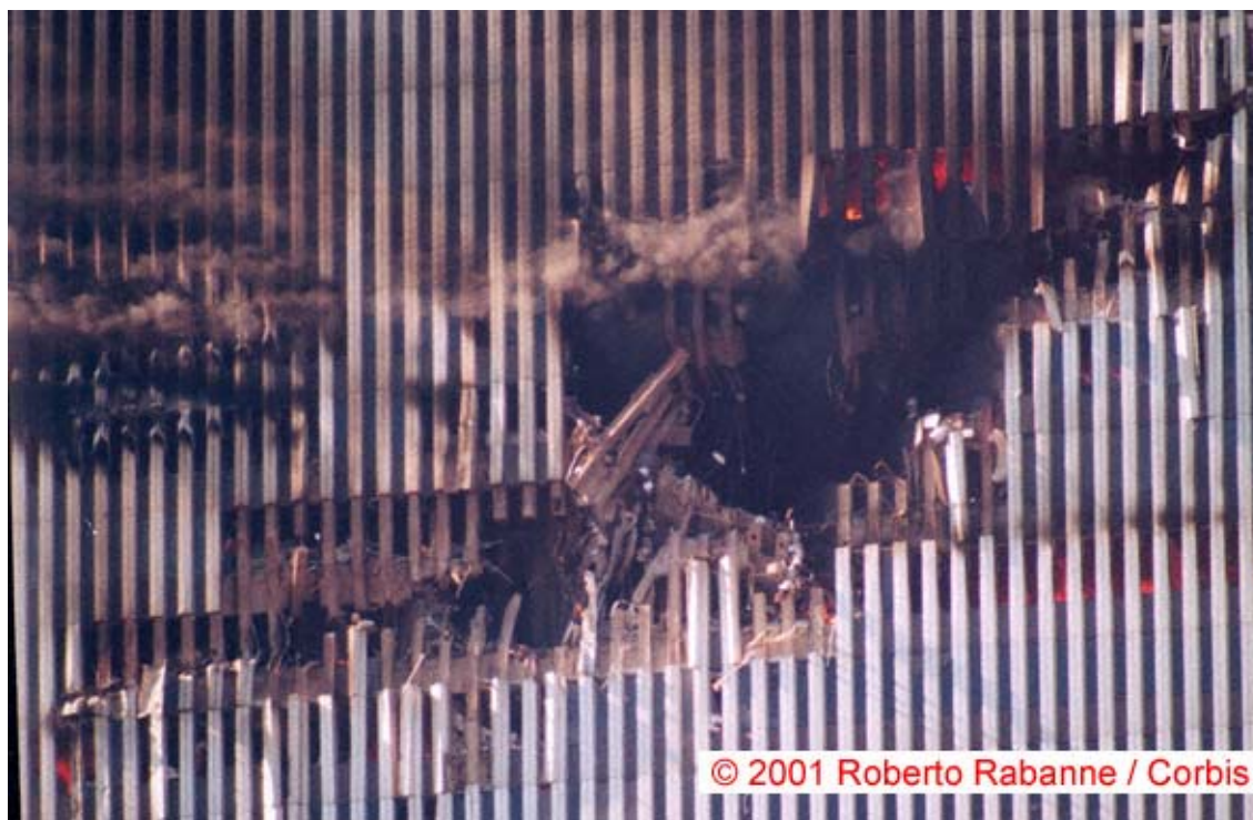
(a) Observed Damage
