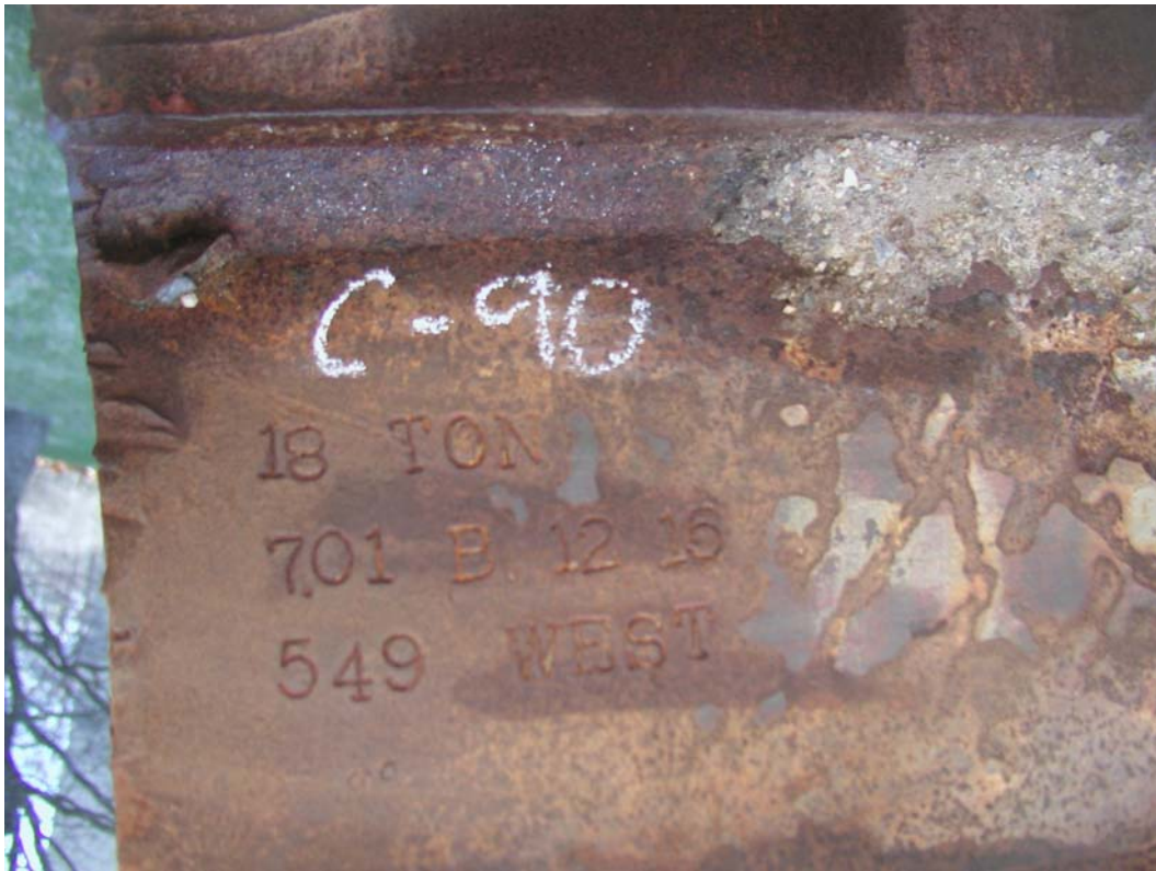
Figure 3–4. Example of stampings placed on one end of a core column.
