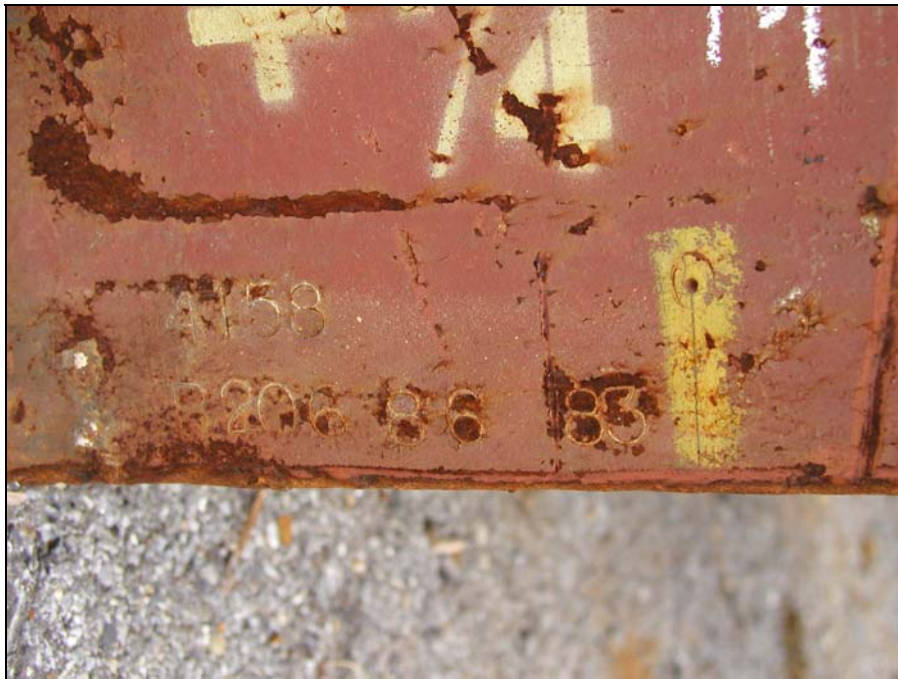
Figure 3–3. Example of stampings on the interior base of the middle column for each panel.
