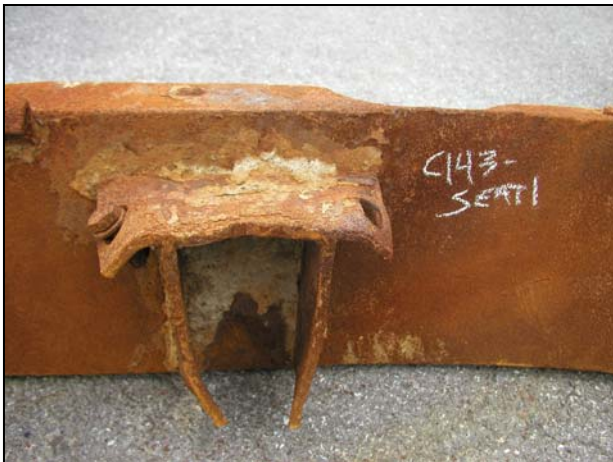
Seat 1: Both holes intact, one has bolt remaining, seat was bent
