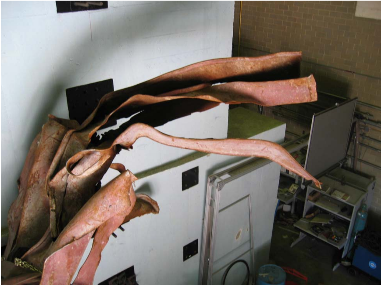
Figure 14. Column elements on Piece M-27 that have decomposed from closed box sections into ribbon-like slender plate elements as a result of the aircraft impact
