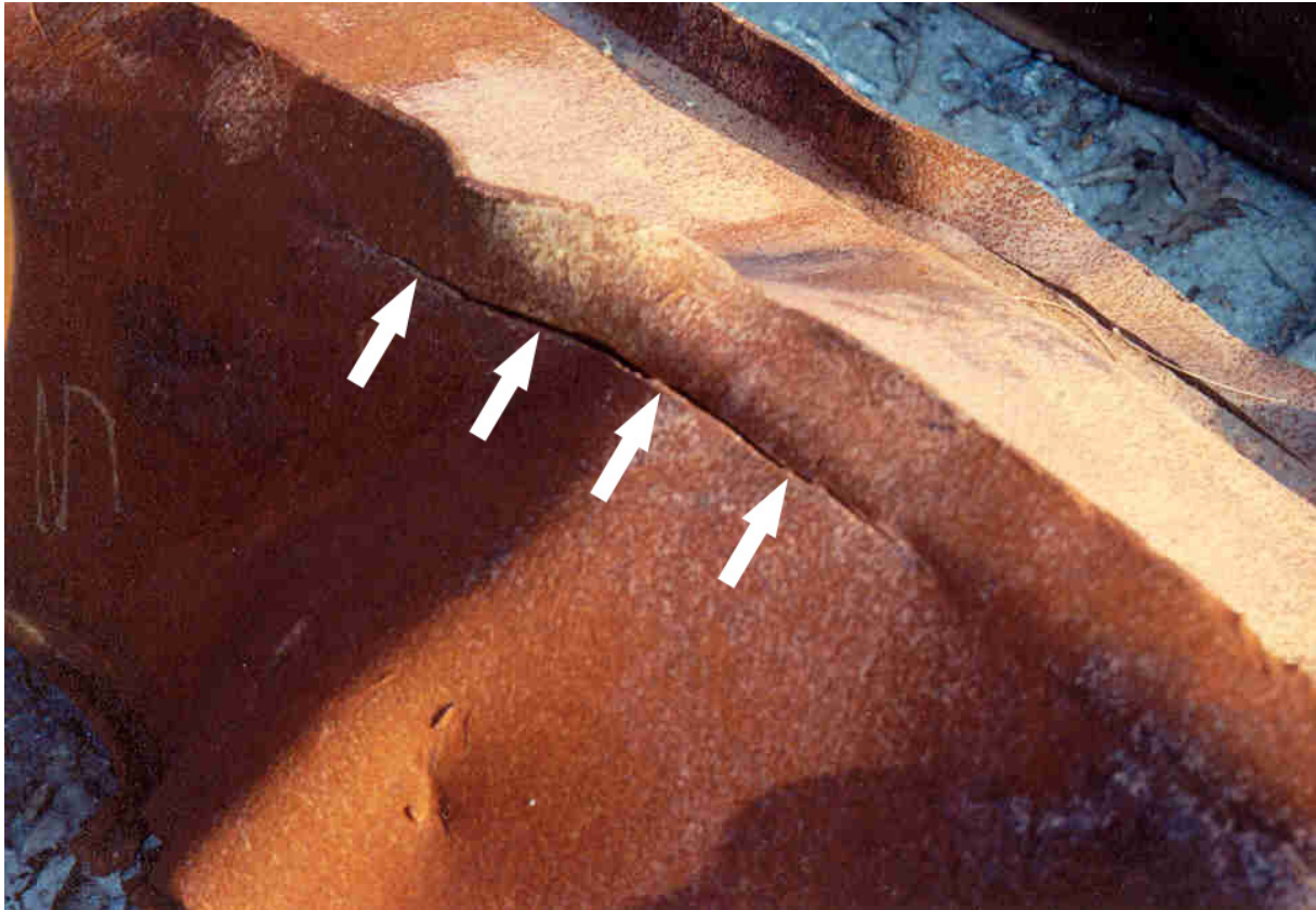
Figure 7. Transverse rupture through the thickness of the parent material, initiating in HAZ at toe of fillet welds
