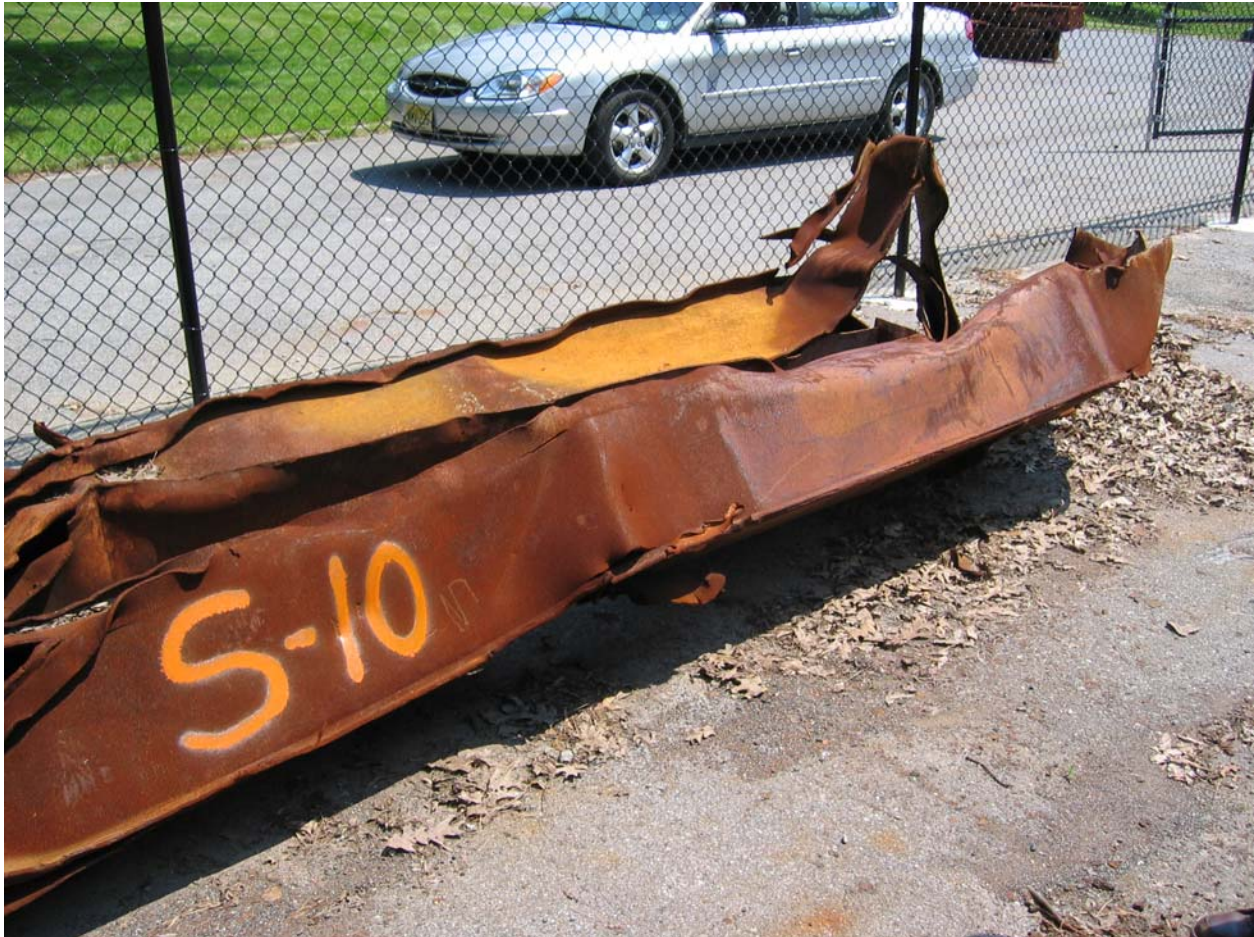
Figure 15. Pattern of possible fire effects (absence of paint at left; presence of paint at right) observable on the side face of Column 224 of Piece S-10
