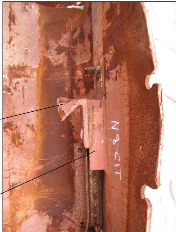
Figure A1b: Type A floor truss connector
