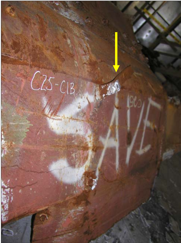
Figure A4a: Type D floor truss connector
