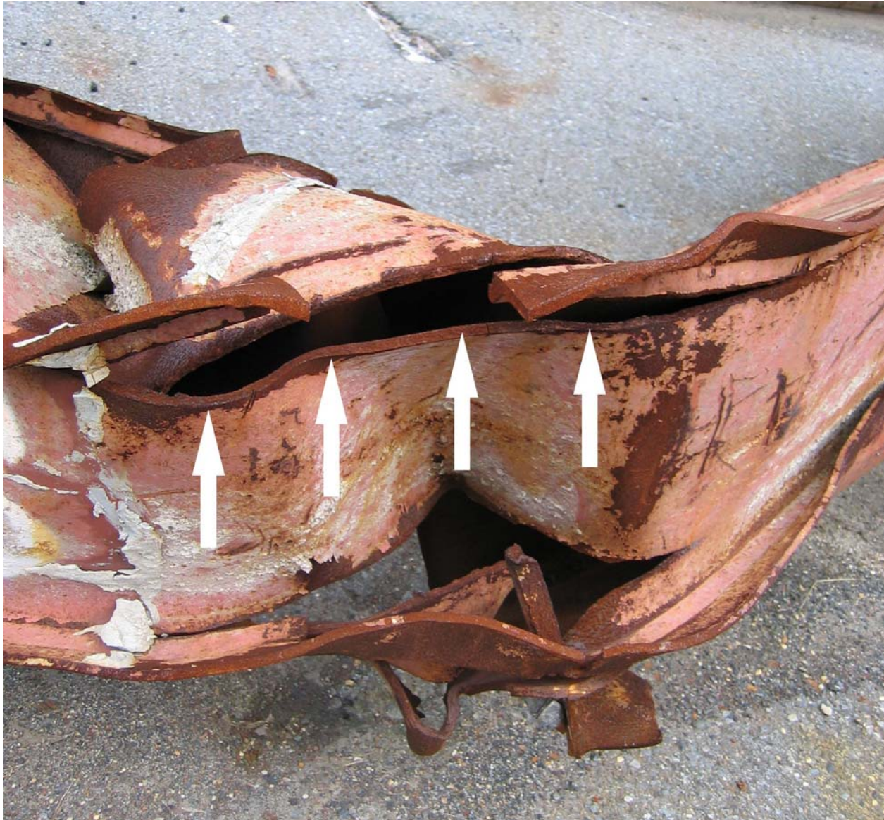
Figure 10. Ruptures of fillet welds through parent material HAZ (at arrows) on probable mechanically pinched zone on Piece C-40 (ruptures through parent material away from welds are also observable in the photo)
