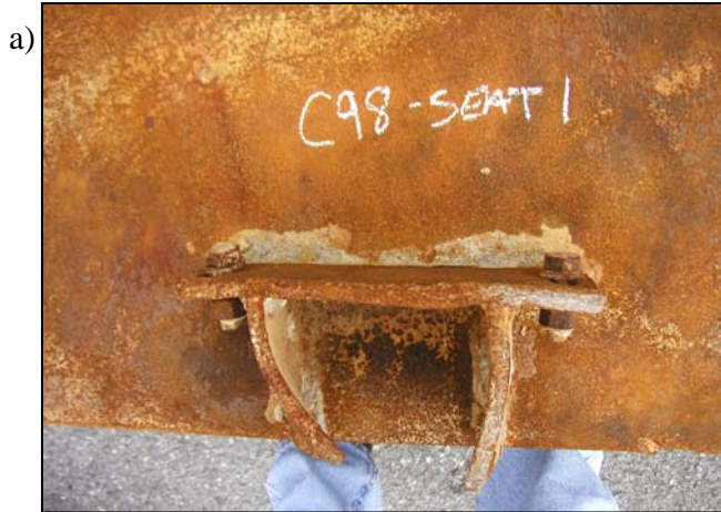
Seat 1: Both holes intact, both have bolts remaining, seat was bent
