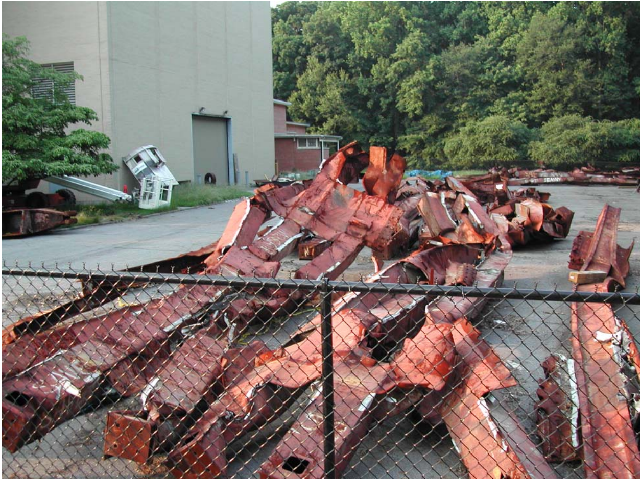
Figure 1. Debris field adjacent to Building 202
