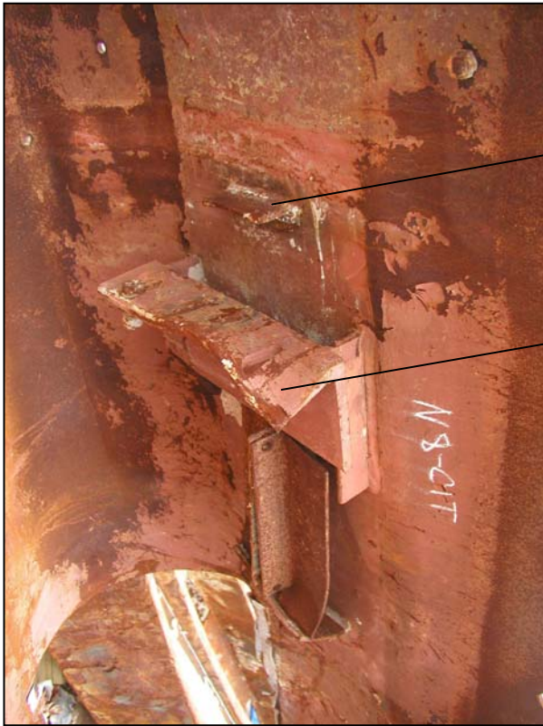
Figure A1a: Type A floor truss connector
