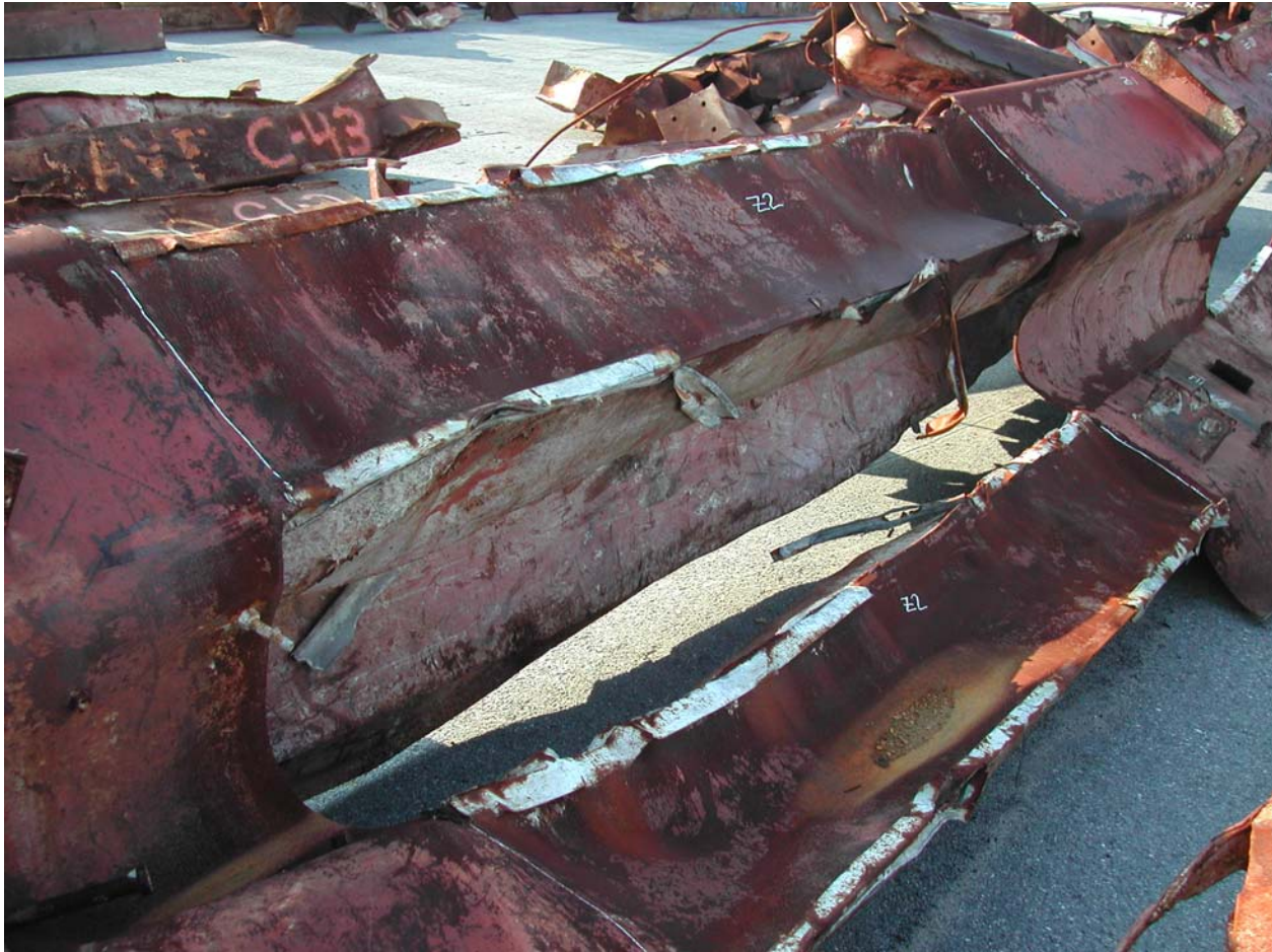
Figure 16. Pattern of presence and absence of possible fire effects on column elements of Piece M-4. Zones marked Z2 at middle are possible fire-effected areas at window openings. Spandrel plates above and below window openings appear unaffected by fire.
