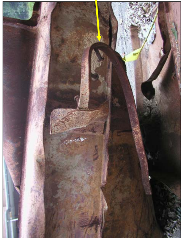
Figure A3d: Type C floor truss connector
