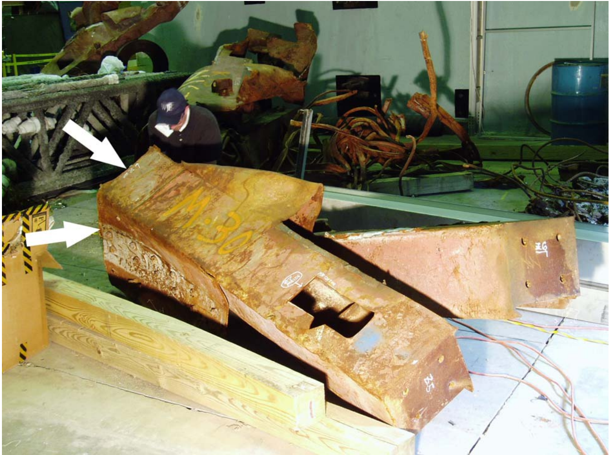
Figure 13. Severed column (at arrows) as observed on Piece M-30.
