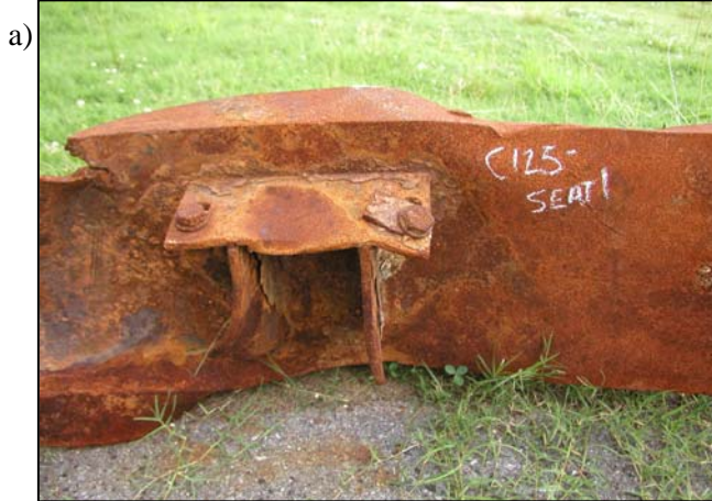
Seat 1: Both holes intact with bolts remaining, one has piece of angle attached, seat was bent
