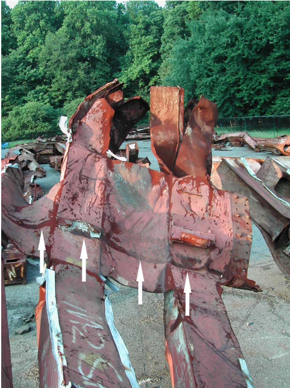
Figure 11. View of Piece M-2, showing inward bend of bottom of piece (at top of photo) about edge of the 97th floor slab(darkened line running left-to-right across spandrel plate, indicated by arrows)
