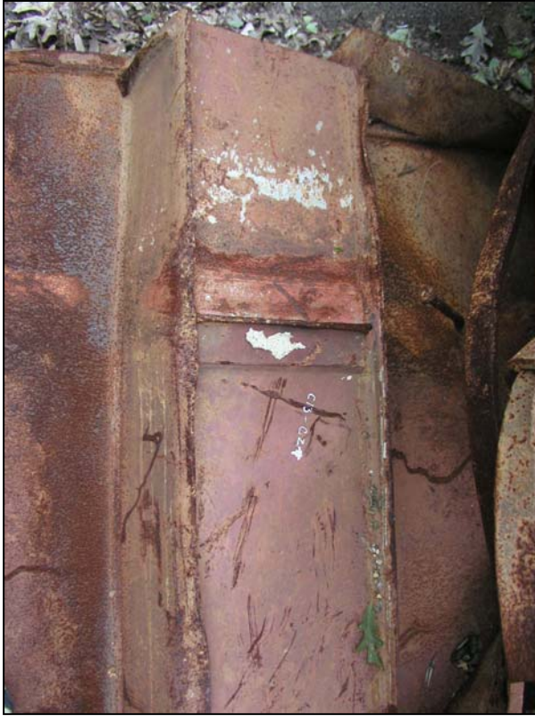
Figure A3c: Type C floor truss connector
