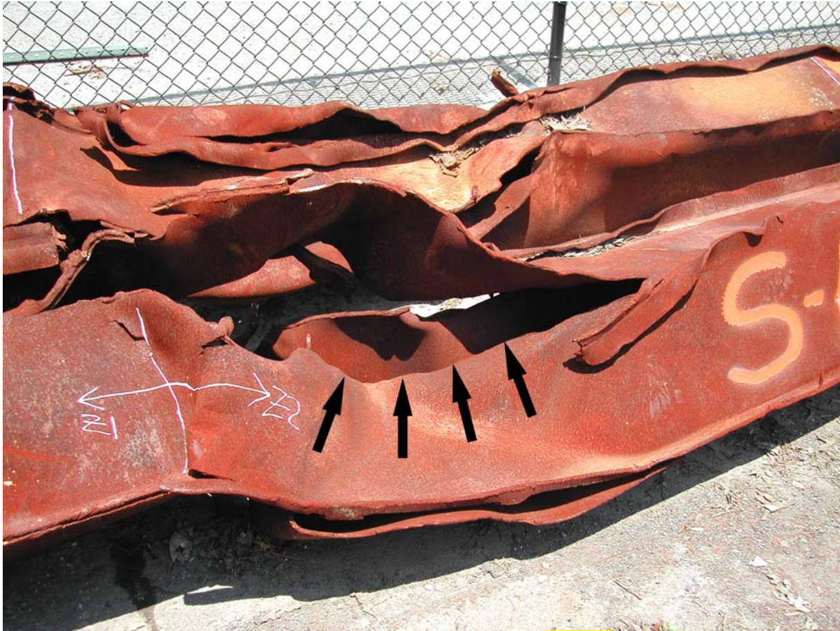
Figure 9. Ruptures of fillet welds through parent material HAZ on possible fire-affected region of Piece S-10
