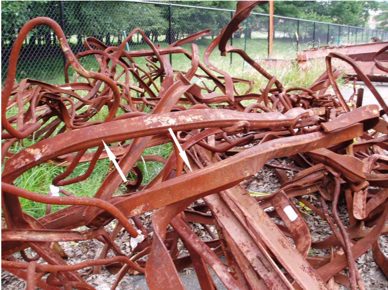
Figure 19. Close view of some recovered floor truss material. Arrows point to truss chords that exhibit longitudinal rib typical of floor trusses manufactured by Laclede Steel
