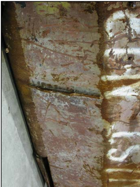
Figure B-34. Floor truss connectors found on recovered panel N-13 (A130: 99-102) from WTC 1. Shown are connectors found on column 130 at different floor levels (cont.).
