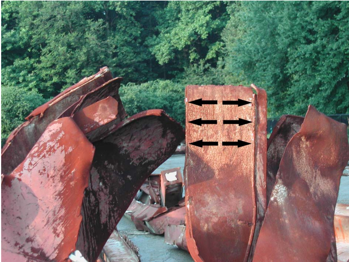
Figure 8. Ruptures of fillet welds through parent material HAZ on impact-affected region of Piece M-2
