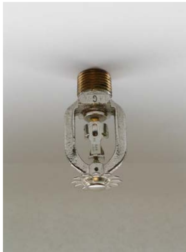
Figure 5–11. Typical standard spray pendent sprinkler.
