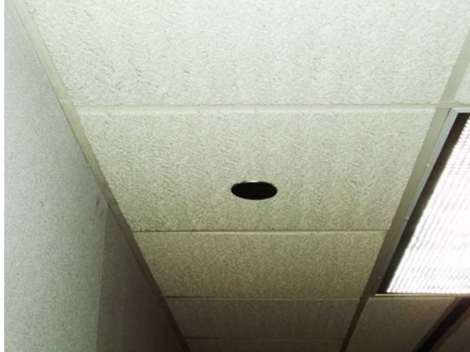
Figure 5–10. Typical concealed pendent sprinkler.
