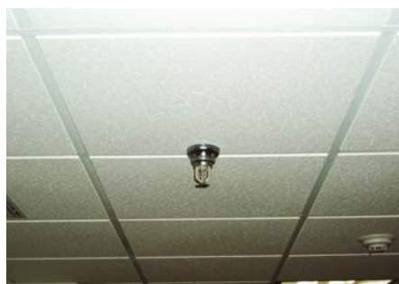
Figure 3–1. Typical sprinkler installed in ceiling.
