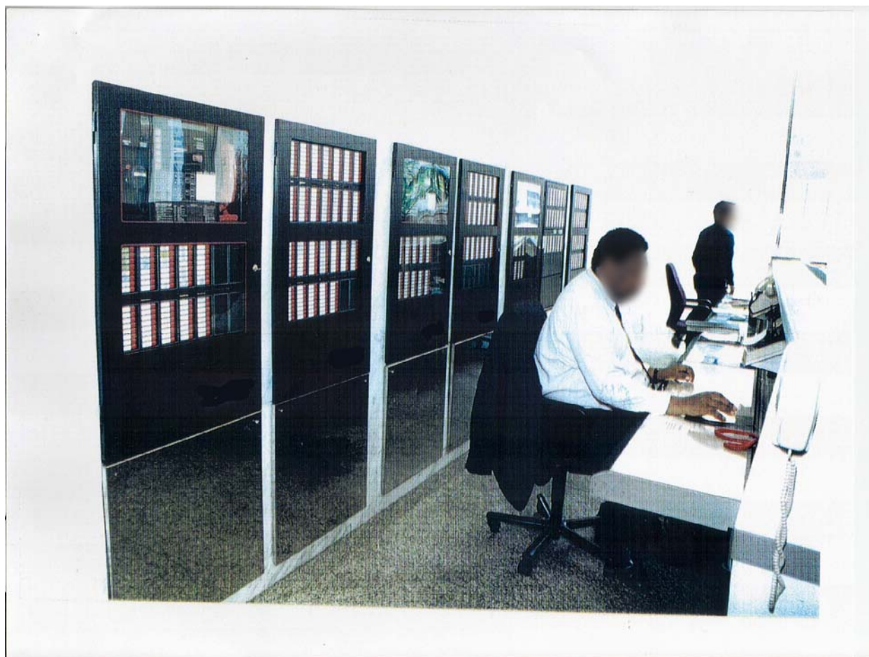
Figure 5–17. WTC 2 fire command station.
