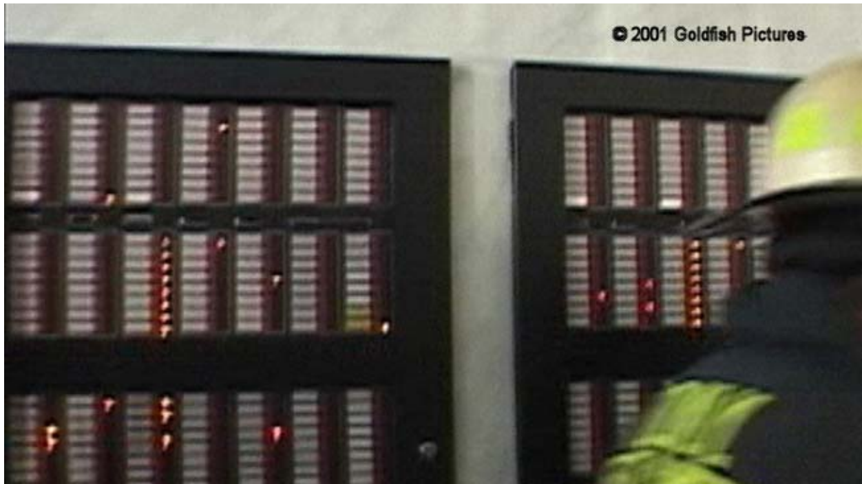
Figure 6–1. WTC 2 speaker and telephone circuit faults.
