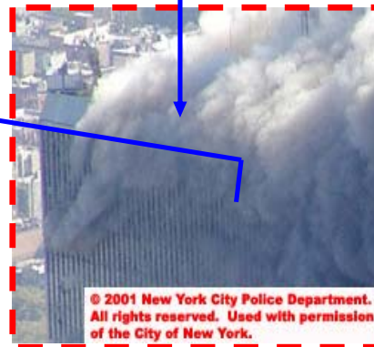
Figure 7–3. Impact damage to north and west faces of WTC 1.
