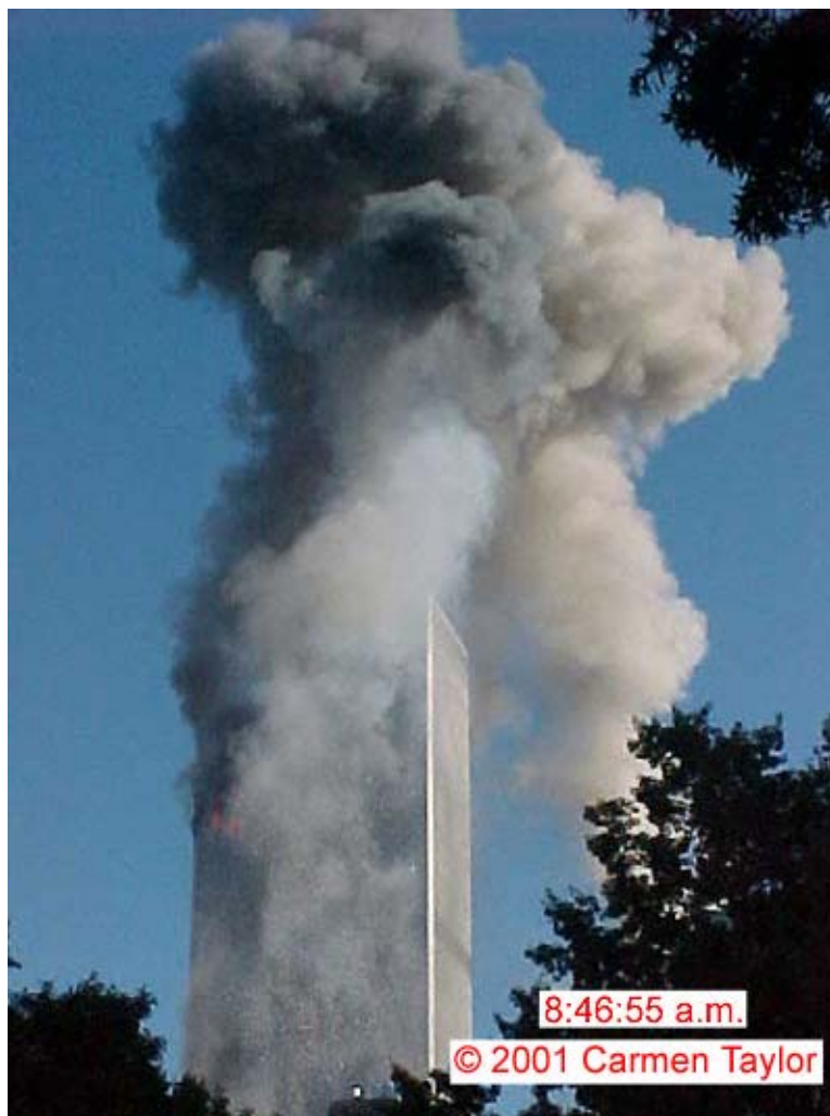
Figure 6-2. View of the WTC towers shot at 8:46:55 a.m. from the southeast shortly after American Airlines Flight 11 struck WTC 1. A dust-filled vortex is visible on the right side. A second area of falling debris can be seen passing on the south side of WTC 2. Significant fires are present on the west side of the south face of WTC 1, which can be seen to the left and behind WTC 2.
