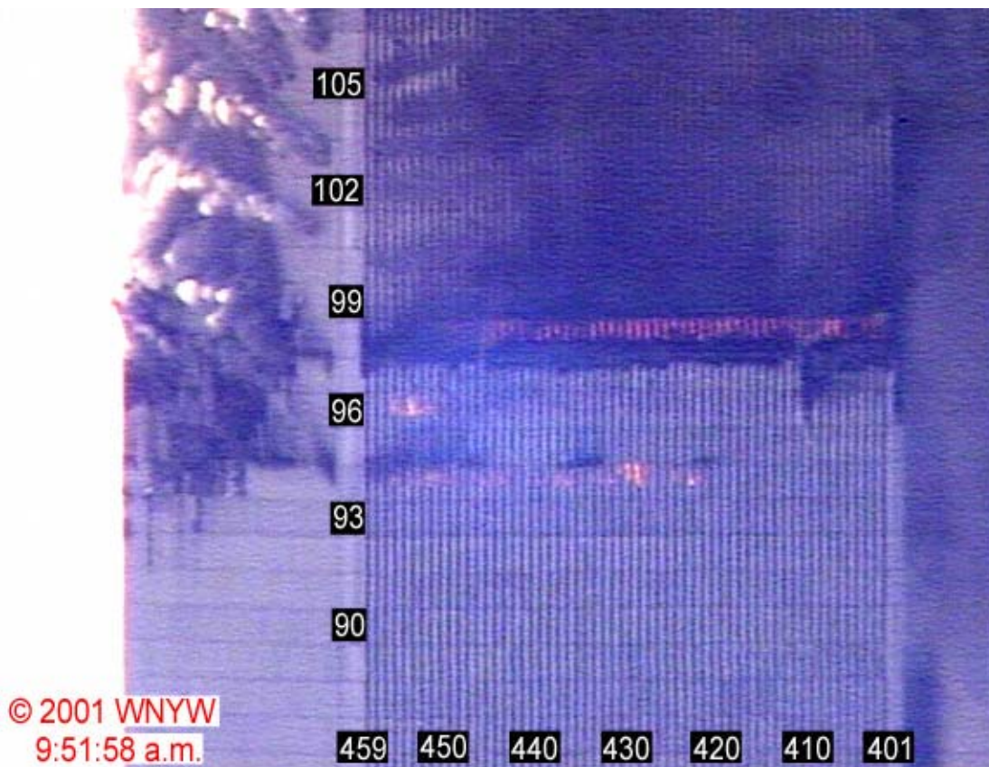
Figure 8-73. This image of the north and west faces of WTC 1 is a frame captured from a video recorded by a news helicopter at 9:51:58 a.m. The image has been enhanced by adjusting the intensity range, and areas to the left of the tower are saturated. Column and floor numbers have been added.
