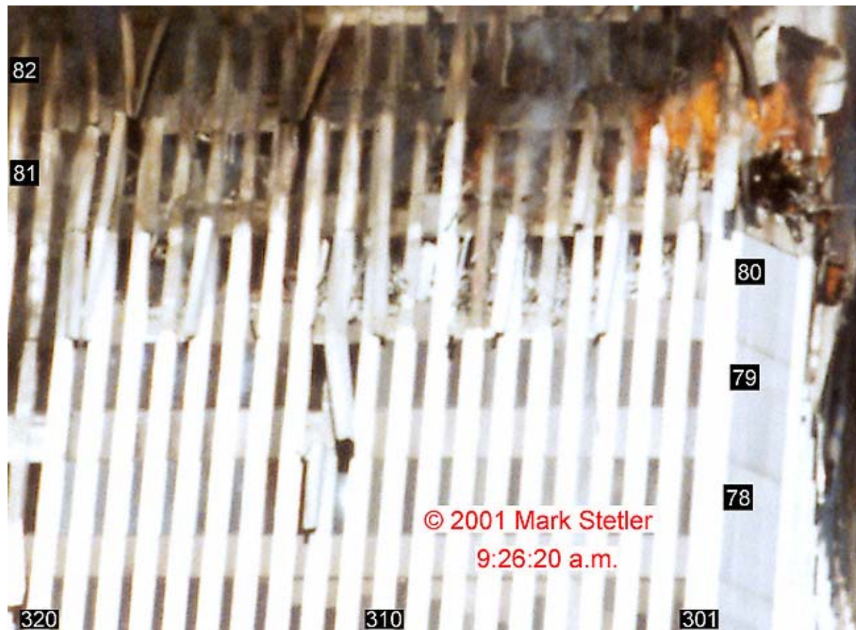
Figure 7-30. This photograph showing a portion of the east face of WTC 2 was cropped from the image shown in Figure 7–28. The image has been rotated, and column and floor numbers have been added. Note the large piles of debris on the 80th and 81st floors.
