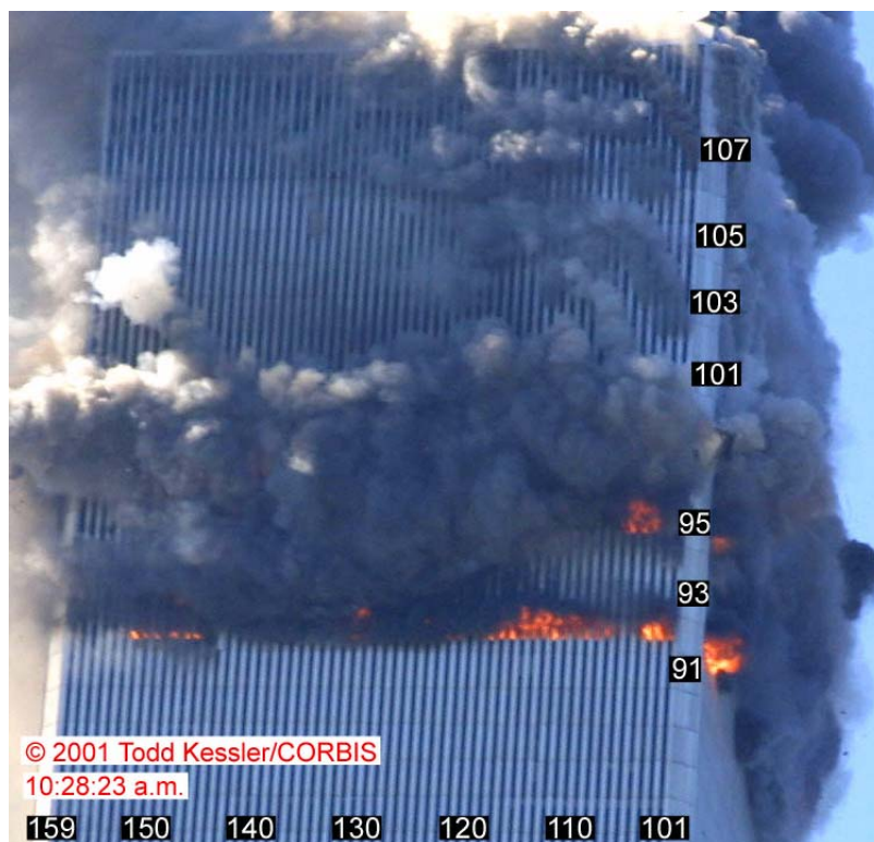
Figure 8-101. This cropped photograph shows the north face of WTC 1 at 10:28:23 a.m. The image has been enhanced by adjusting the intensity levels. Column and floor numbers have been added.
