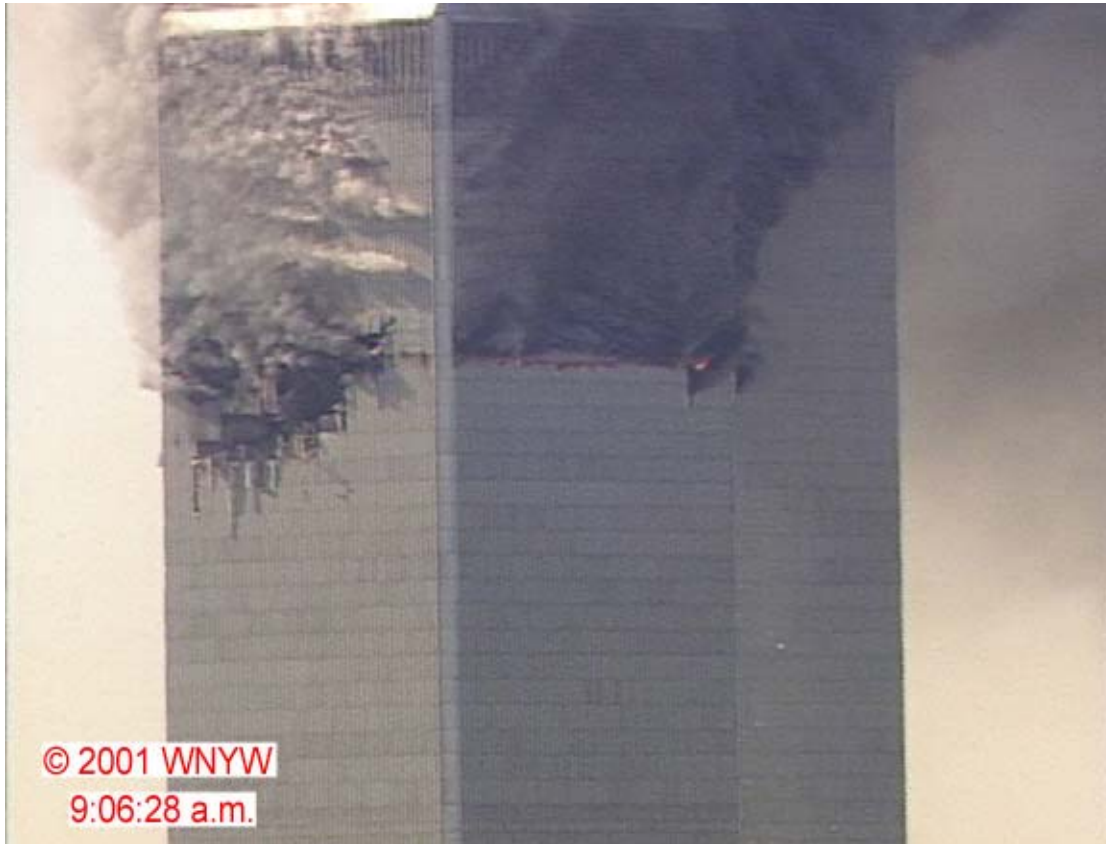
Figure 8-29. This image of the north and west faces of WTC 1 is a frame from a video recorded by a news helicopter at 9:06:28 a.m. WTC 2 can be seen behind WTC 1. Note the burst of flame from near window 97-408 at the southwest corner of WTC 1.
