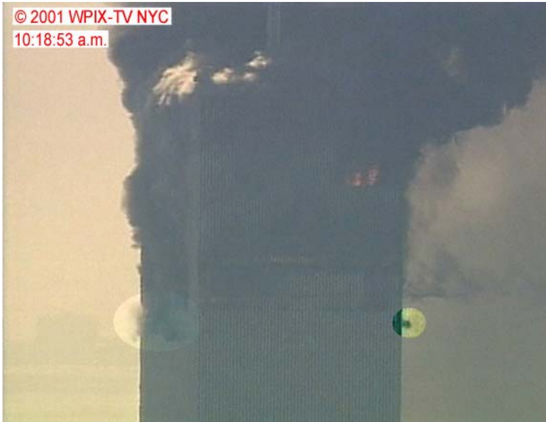
Figure 8-97. This image showing the west face and an oblique view of the north face was captured from a video shot from a news helicopter at 10:18:53 a.m. The highlighted areas with adjusted intensities indicate smoke and/or dust plumes that were pushed from the north and south faces by a pressure pulse that passed through the tower at 10:18:48 a.m.
