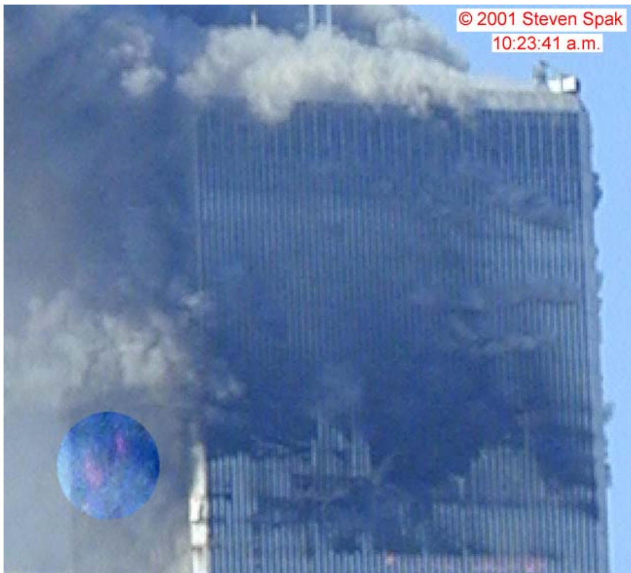
Figure 8-103. This cropped photograph shows the north face and an oblique view of the east face of WTC 1 at 10:23:41 a.m. The intensity levels in an area of the east face have been adjusted to highlight an area of extended flame.
