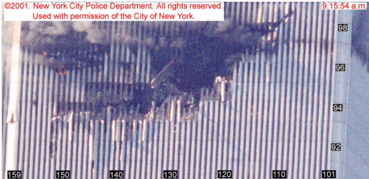
Figure 8-19. An image recorded at 9:15:54 a.m. shows the north face of WTC 1. The original has been cropped, rotated, and enhanced. Column and floor numbers have been added.
