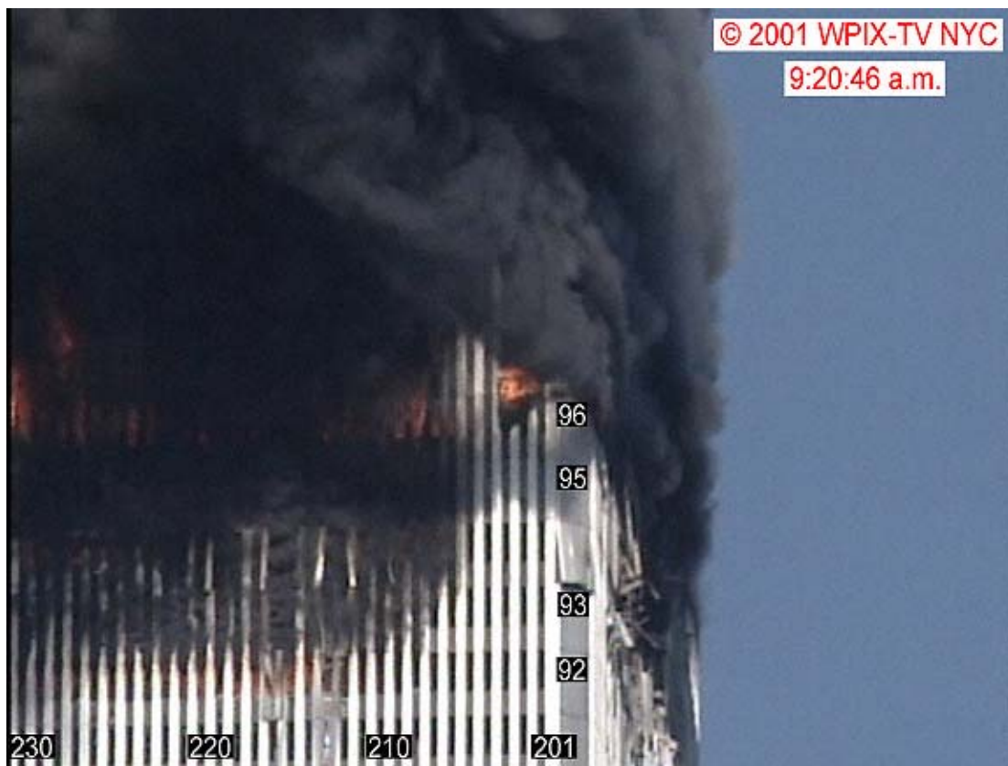
Figure 8-41. A frame taken from a video shows a portion of the east face of WTC 1 at 9:20:46 a.m. The image has been enhanced. Column and floor numbers have been added.
