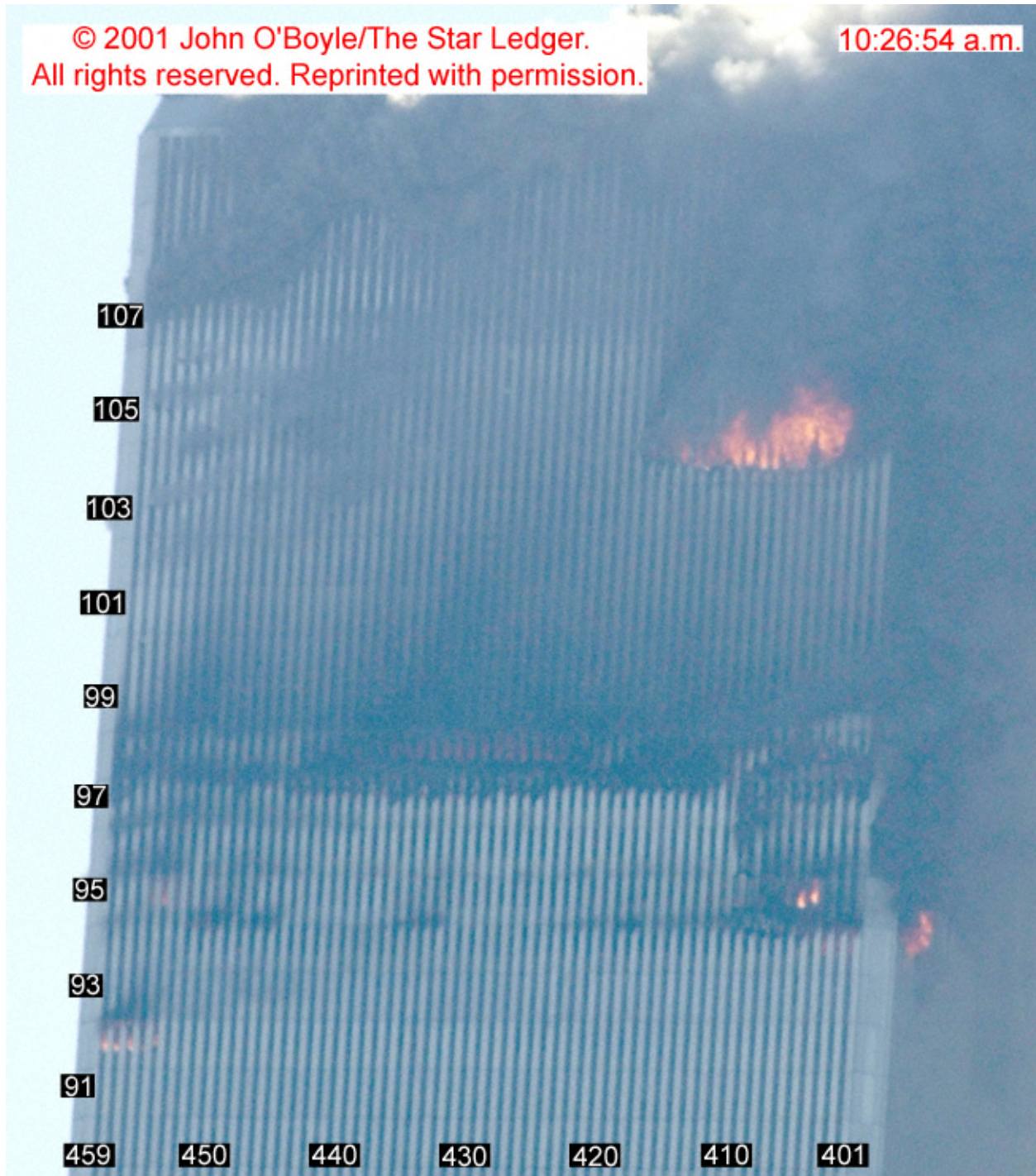
Figure 8-114. This cropped photograph showing the west face of WTC 1 was taken at 10:26:54 a.m. The image has been enhanced by adjusting the intensity levels, and column and floor numbers have been added.
