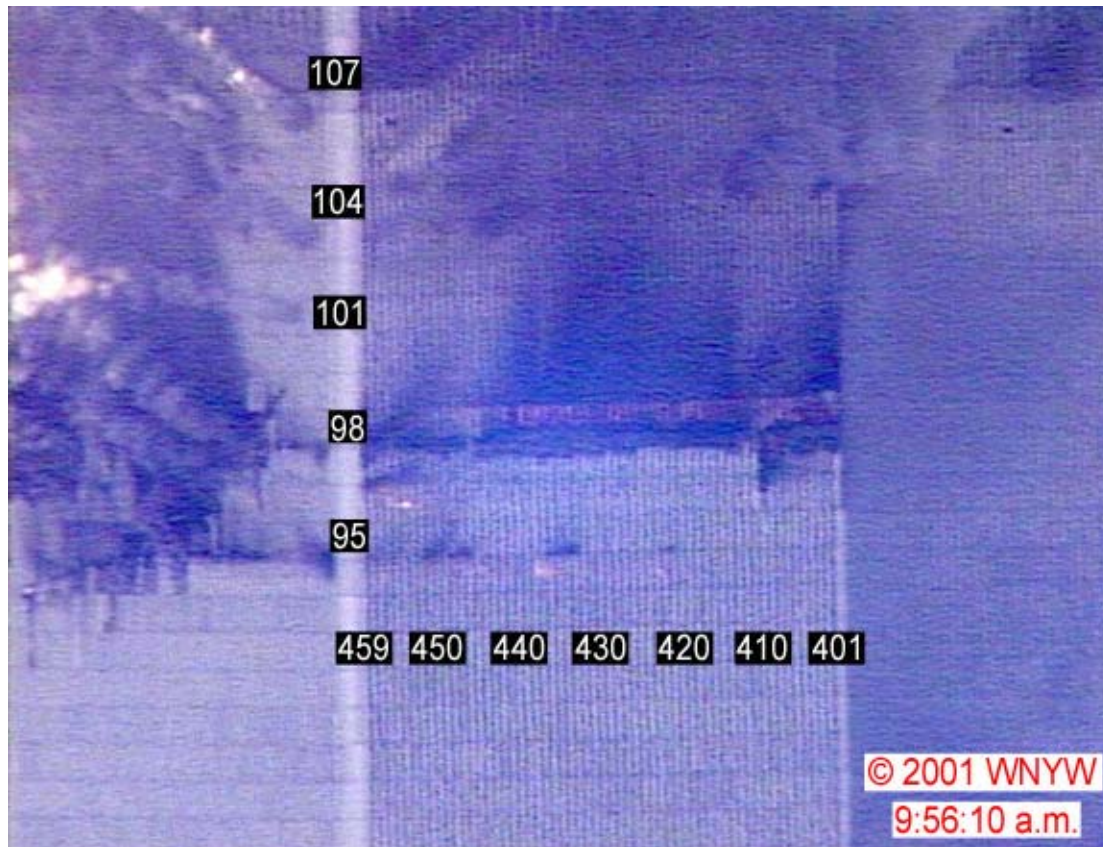
Figure 8-74. This image of the north and west faces of WTC 1 is a frame captured from a video recorded by a news helicopter at 9:56:10 a.m. The image has been enhanced by adjusting the intensity range. WTC 2 appears in the background to the right. Column and floor numbers have been added to WTC 1.
