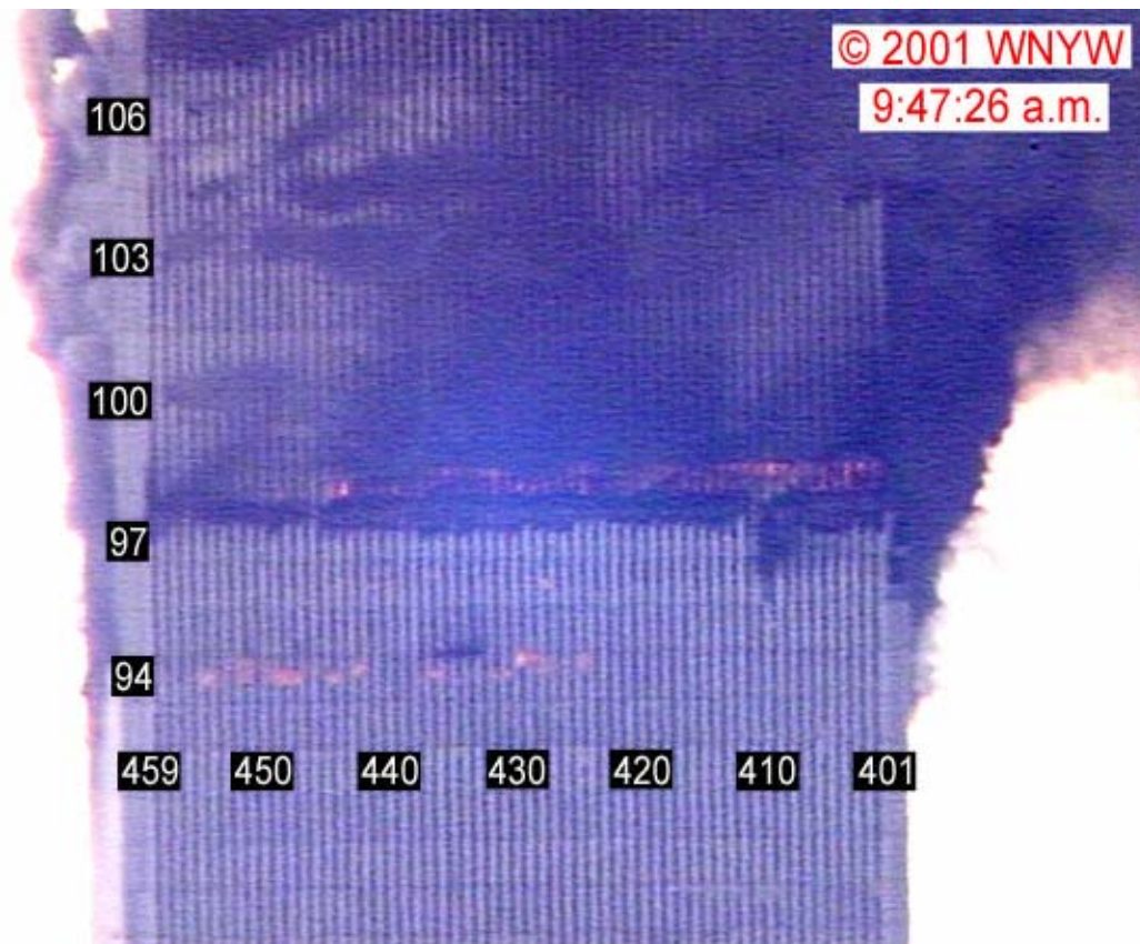
Figure 8-71. This image of the west face of WTC 1 is a frame captured from a video recorded by a news helicopter at 9:47:26 a.m. The image has been enhanced by adjusting the intensity range, and areas to the left and right of the tower are saturated. Column and floor numbers have been added.
