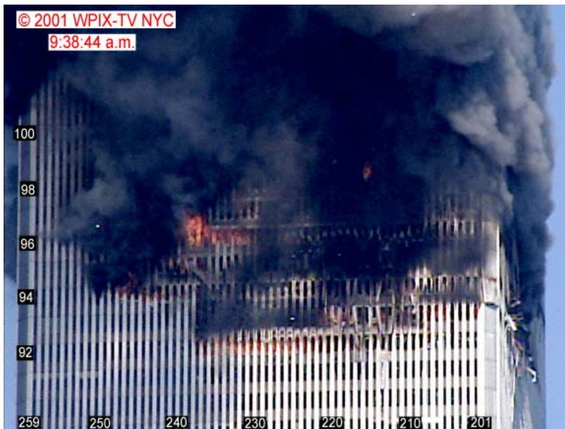
Figure 8-57. This image of the east face of WTC 1 was captured from a video recorded at 9:38:44 a.m. It has been enhanced by adjusting the intensity levels. Column and floor numbers have been added.
