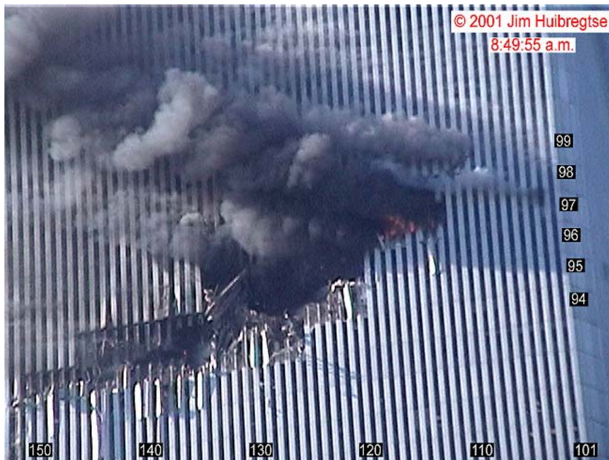
Figure 8-1. This image is extracted from a video recording that shows the north face of WTC 1 at 8:49:55 a.m. Column and floor numbers have been added.
