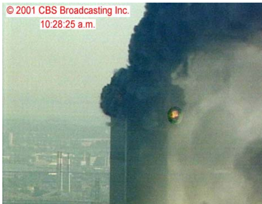
Figure 8-111. This image showing the south face of WTC 1 was taken from a video shot from a news helicopter at 10:28:25 a.m. The intensity levels of the image have been adjusted. An area showing a fireball generated by fire pushed from the tower by the collapse is highlighted.
