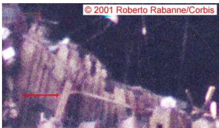
Figure 6-8. An enlarged and enhanced portion of Figure 6–5 shows a portion of one of WTC 1’s floor slabs that has collapsed into the opening created by the aircraft impact. The corrugated steel on the bottom of the floor slab and a portion of one of the support trusses (indicated by an arrow) can be seen.
