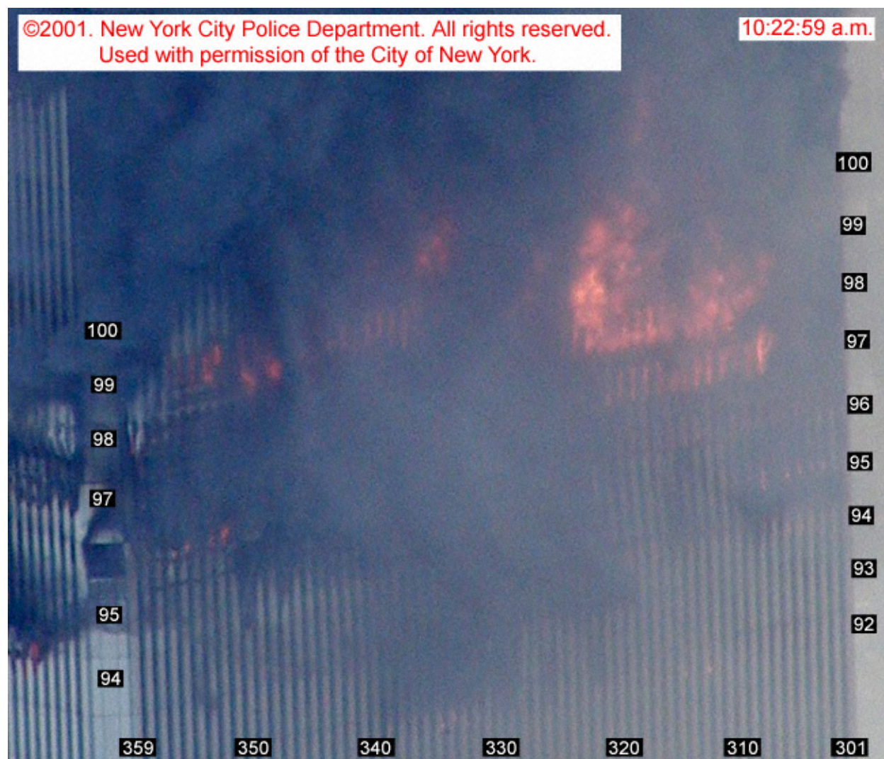
Figure E–9. This photograph showing the south face of WTC 1 is a cropped version of a photograph shot from a helicopter at 10:22:59 a.m. It has been enhanced by adjusting the intensity levels, and column and floor numbers have been added.
