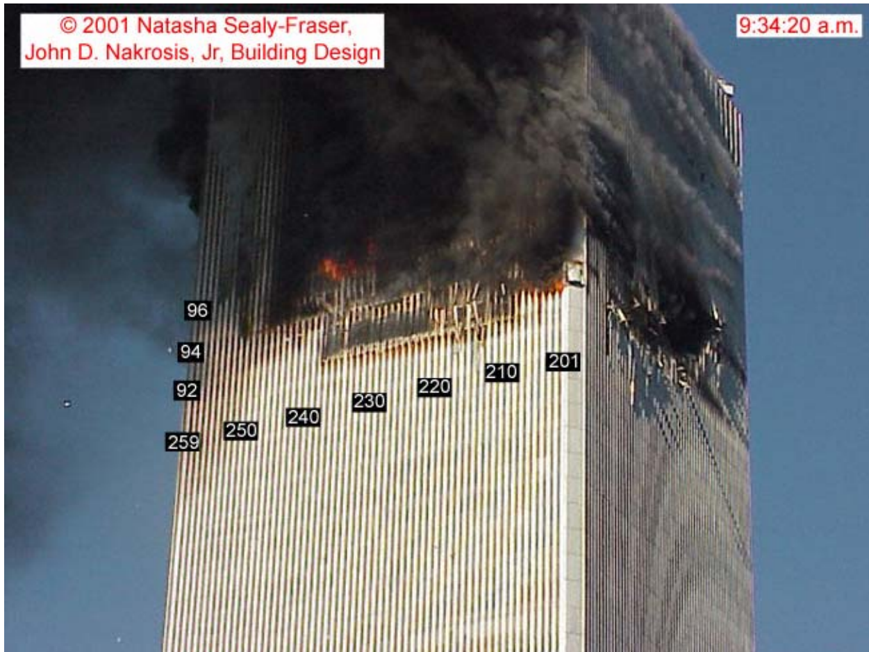
Figure 8-43. Photograph of the east face of WTC 1 recorded at 9:34:20 a.m. Column and floor numbers have been added.
