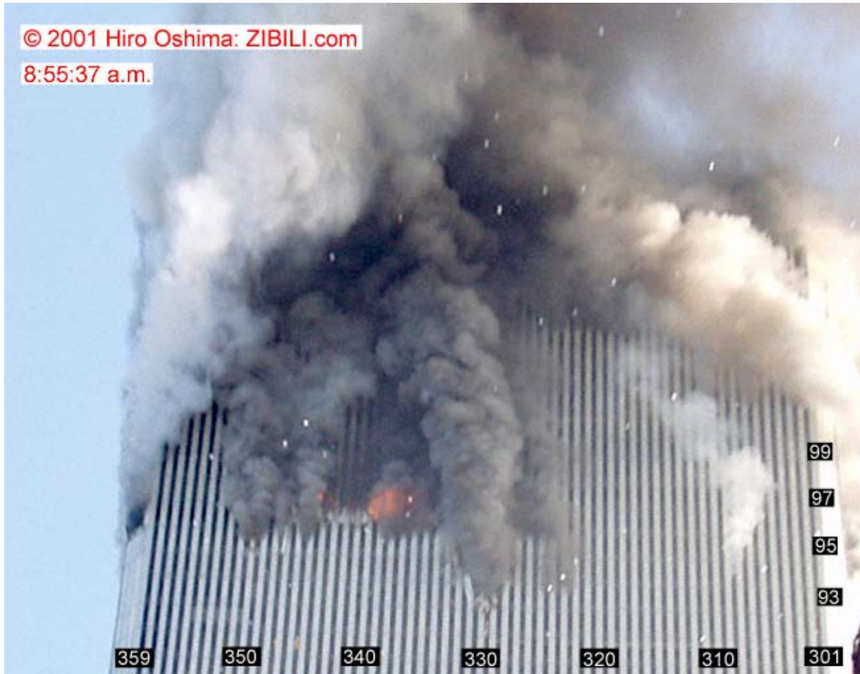
Figure 6-13. This enhanced and cropped photograph shows the south face of WTC 1 at 8:55:37 a.m. Column and floor numbers have been added.
