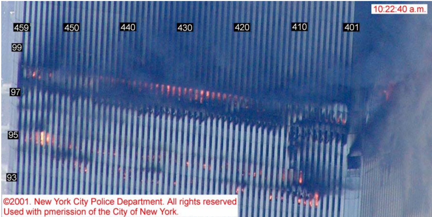
Figure 8-112. This cropped photograph was shot from a helicopter at 10:22:40 a.m. and shows the west face of WTC 1 from above. The image has been enhanced by adjusting the intensity levels, and column and floor numbers have been added.
