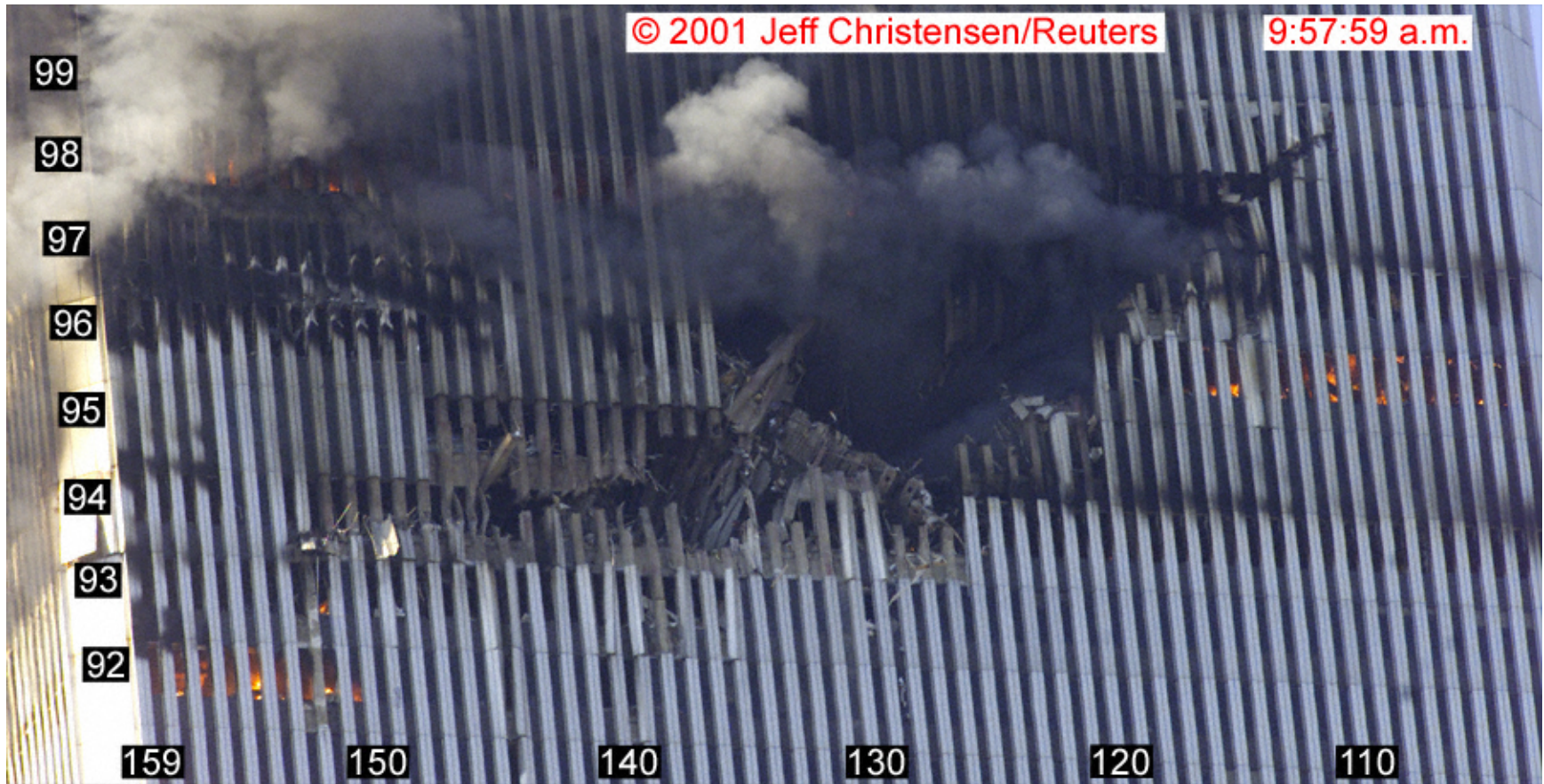
Figure 8-55. This image shows the north face of WTC 1 at 9:57:59 a.m. The original has been rotated, cropped, and enhanced. Column and floor numbers have been added.
