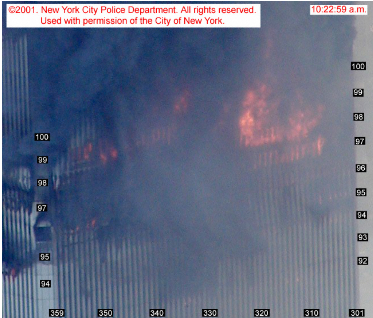
Figure 8-108. This photograph showing the south face of WTC 1 is a blowup of a portion of Figure 8-107. It was shot from a helicopter at 10:22:59 a.m. It has been enhanced by adjusting the intensity levels, and column and floor numbers have been added.
