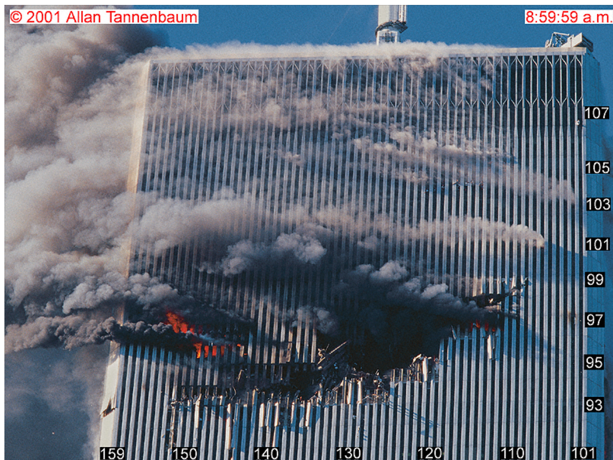
Figure 8-8. This photograph of the north face of WTC 1 was recorded at 8:59:59 a.m. The image has been cropped and floor and column numbers have been added.
