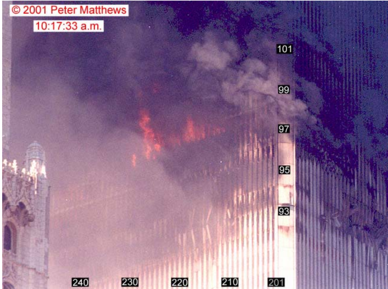
Figure 8-86. This photograph shows the north and east faces of WTC 1 at 10:17:33 a.m. The original has been cropped and enhanced by adjusting the intensities. Column and floor numbers have been added.
