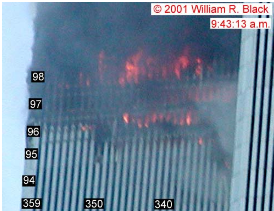
Figure 8-62. This cropped photograph of the south face of WTC 1 was recorded at 9:43:13 a.m. The image has been rotated and enhanced. WTC 2 appears at the right. Column and floor numbers have been added.
