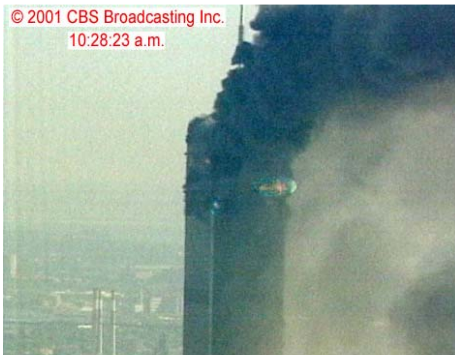
Figure 8-110. This image showing the south face of WTC 1 was taken from a video shot from a news helicopter at 10:28:23 a.m. The intensity levels of the image have been adjusted. Two areas showing flames that were pushed out of the tower as it started to collapse are highlighted.
