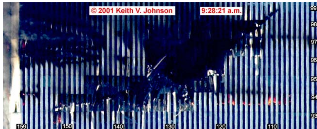
Figure 8-37. This cropped photograph shows the north face of WTC 1 at 9:28:21 a.m. The image has been rotated and enhanced. Column and floor numbers have been added.
