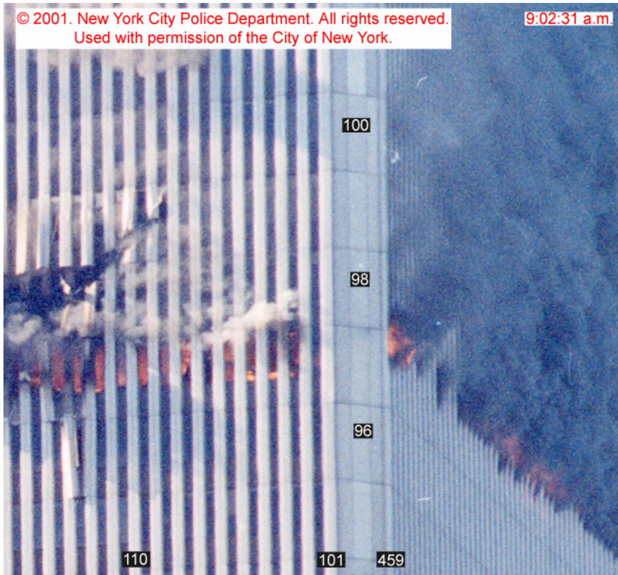
Figure 8-12. This photograph was shot from the northwest and shows the north and west faces of WTC 1 at 9:02 31 a.m. The image has been cropped and the intensity levels have been adjusted. Column and floor numbers have been added.
