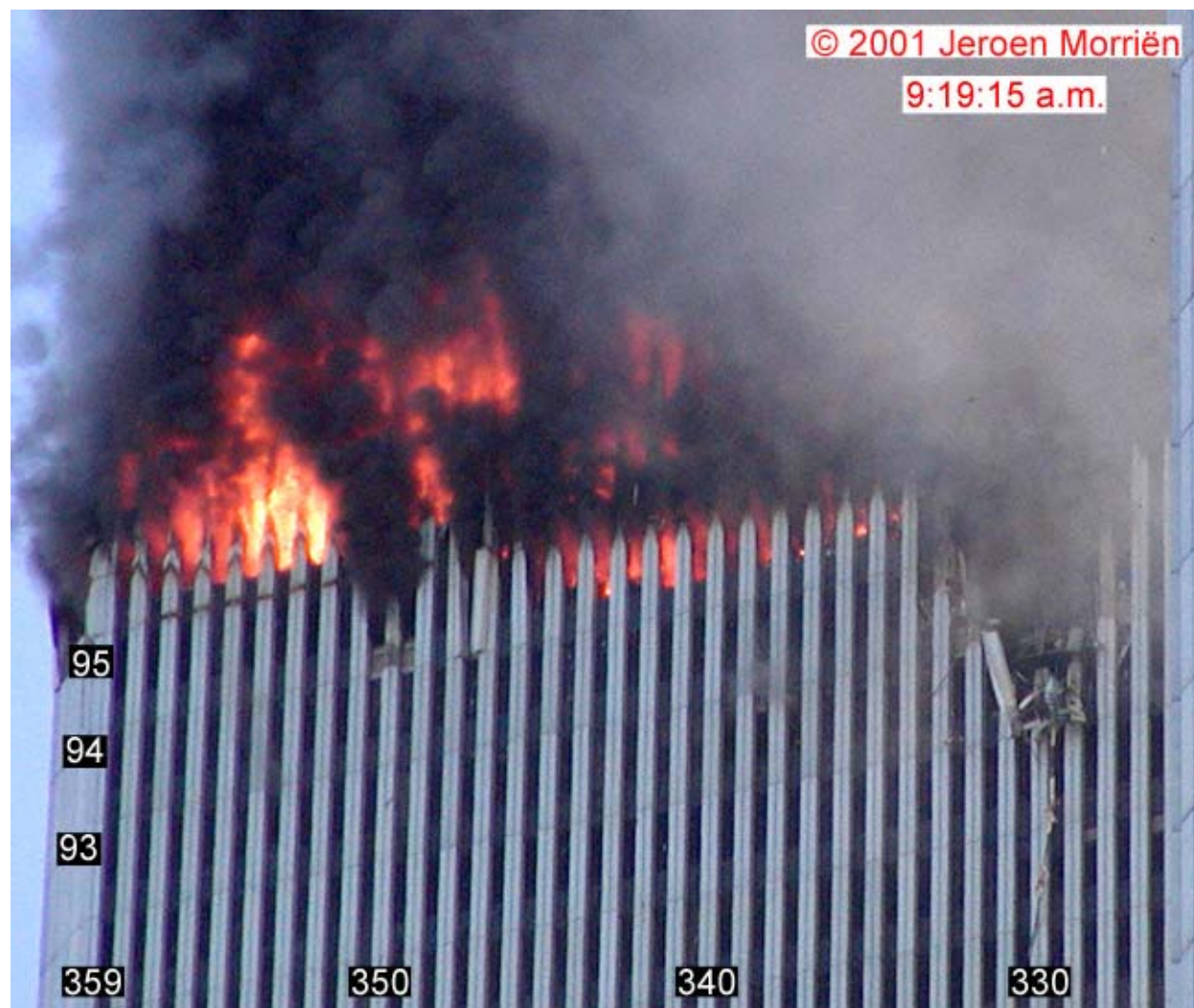
Figure 8-44. This cropped image shows a portion of the south face of WTC 1 at 9:19:15 a.m. The photograph has been enhanced and column and floor numbers have been added. The corner of WTC 2 is visible at the far right side of the image.
