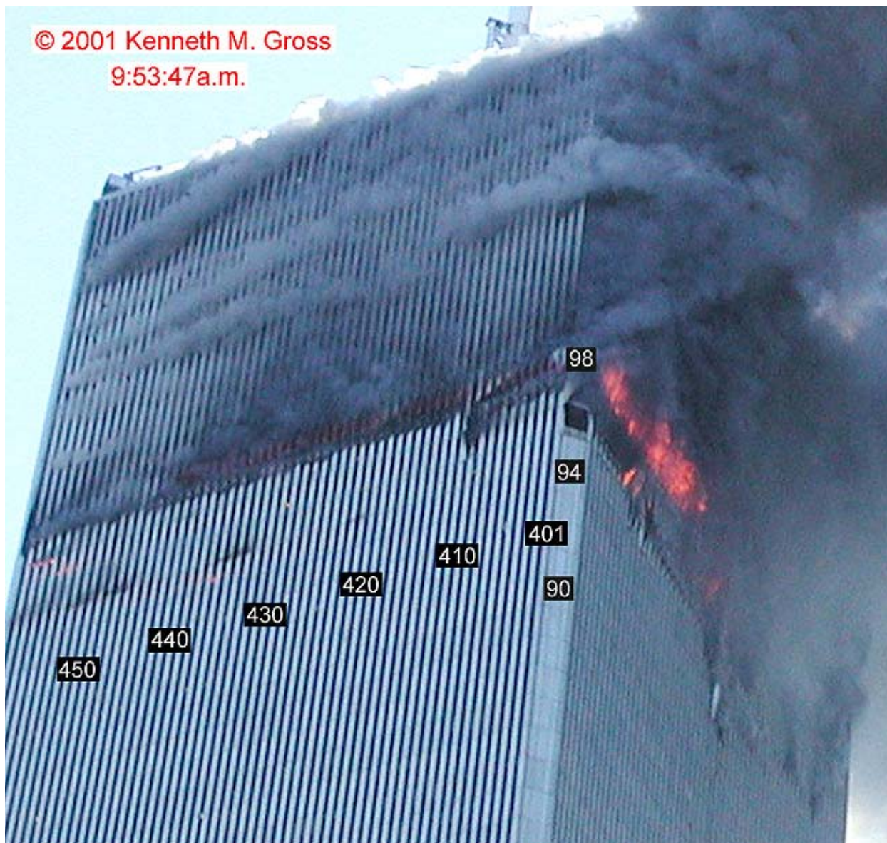
Figure 8-65. A photograph shot from the southwest shows the west and south faces of WTC 1 at 9:53:47 a.m. The original image has been cropped and enhanced. Column numbers for the west face and floor numbers have been added.
