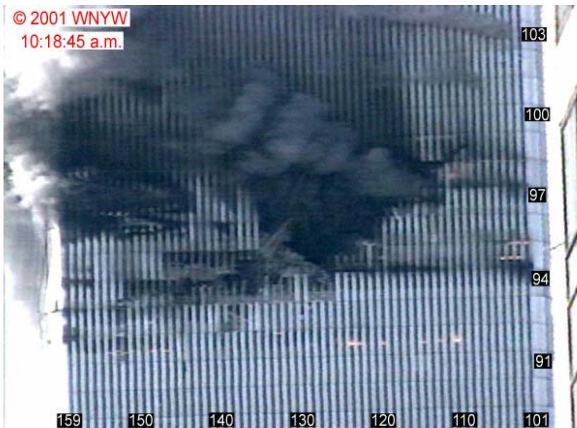
Figure 8-94. This image of the north face of WTC 1 was captured from a video shot at 10:18:45 a.m. It has been enhanced by adjusting the intensity range. Some portions of the image to the left of the tower are saturated. Column and floor numbers have been added.
