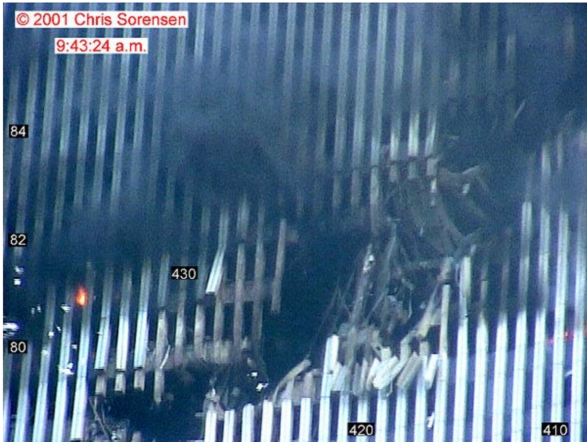
Figure 7-23. A frame captured from a video recording of the aircraft impact location on the south face of WTC 2 is shown. The image has been enhanced by adjusting the intensity levels. Column numbers and floor numbers have been added.
