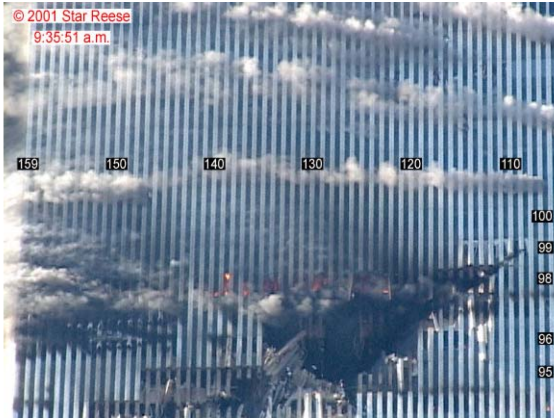
Figure 8-38. A frame taken from a video shows the north face of WTC 1 at 9:35:51 a.m. The image has been enhanced. Column and floor number have been added.
