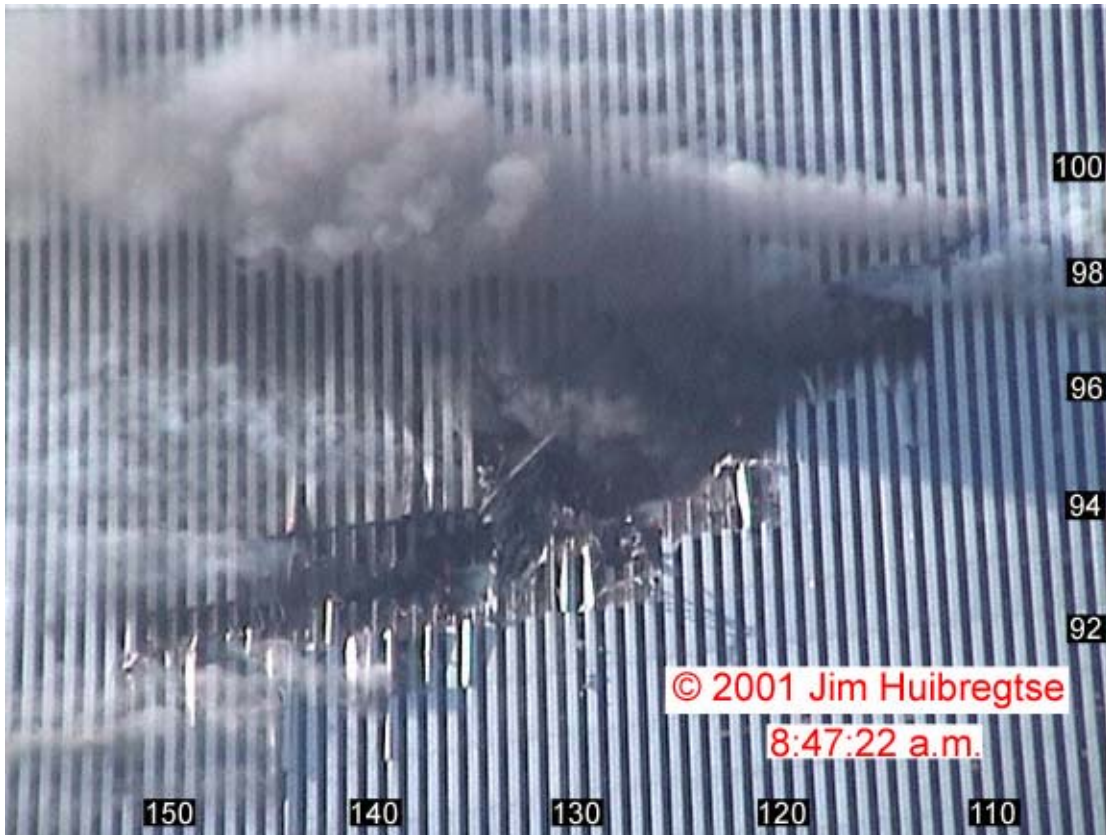
Figure 6-4. This image of the north face of WTC 2 is a frame taken from a video recorded at 8:47:22 a.m. Column and floor numbers have been added.
