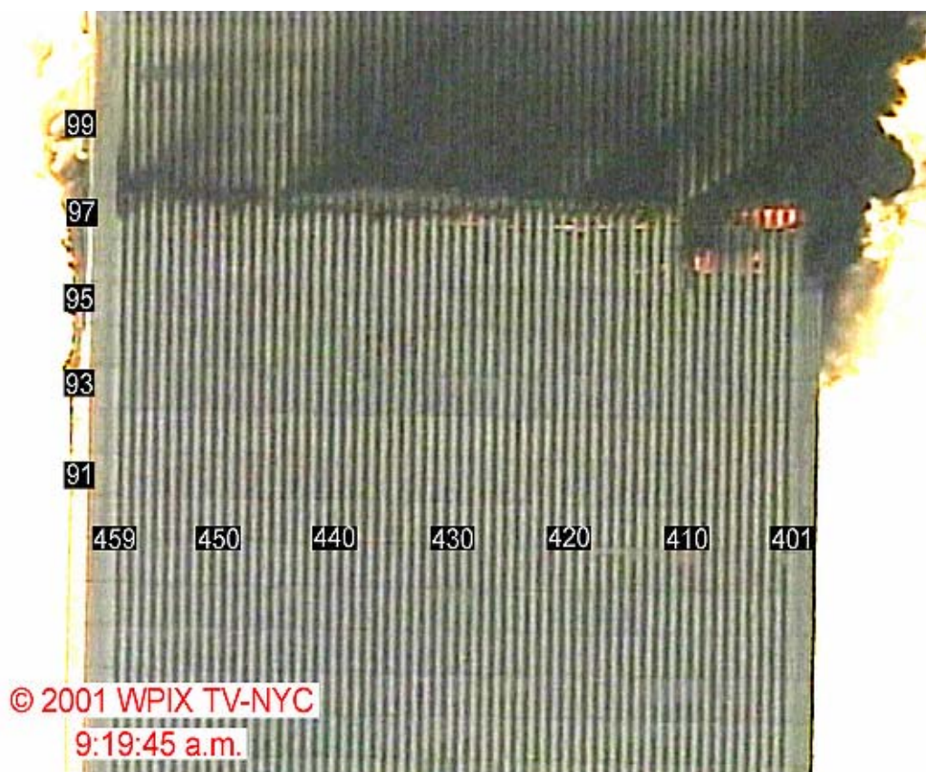
Figure 8-47. This image of the west face of WTC 1 is a frame captured from a video recorded by a news helicopter at 9:19:45 a.m. The image has been enhanced by adjusting the intensity range, and areas to the left and right of the tower are saturated. Column and floor numbers have been added.
