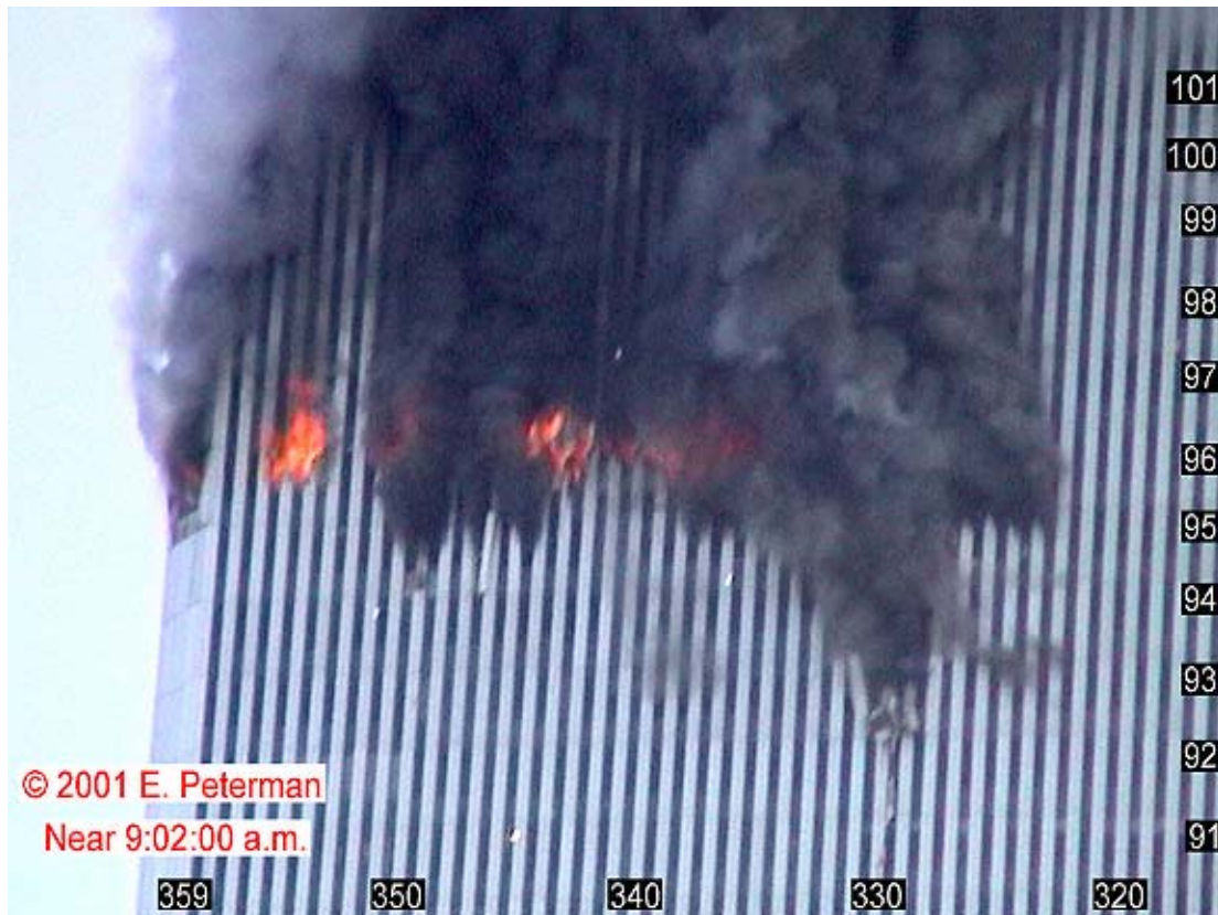
Figure 8-10. This image showing the south face was captured from a video. It was not possible to time this image exactly, but it was recorded within a minute of 9:02 a.m. Column and floor numbers have been added.
