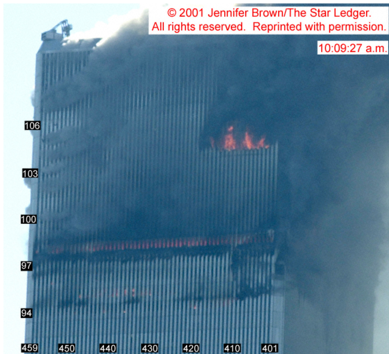
Figure 8-91. This photograph, showing the west face of WTC 1 and an oblique view of the south face, was recorded at 10:09:27 a.m. The image has been cropped and enhanced by adjusting intensity levels. Column and floor numbers have been added.
