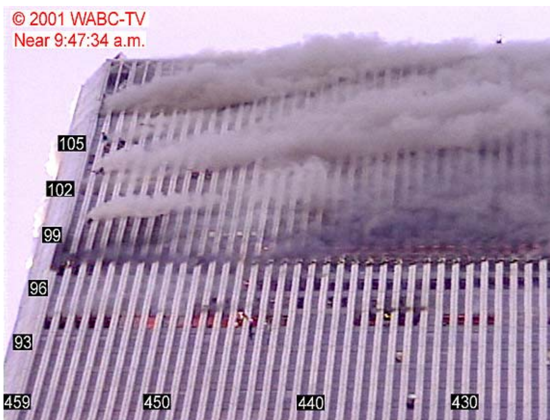
Figure 8-72. This view of the west face of WTC 1 was captured from a video recorded at 9:47:34 a.m. There is a 30 s uncertainty in the assigned time. The image has been enhanced by adjusting the intensity levels, and some locations above the building are saturated. Column and floors numbers have been added.
