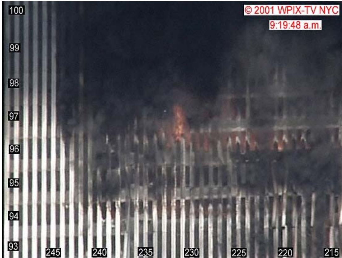
Figure 8-40. A frame taken from a video shows a portion of the east face of WTC 1 at 9:19:48 a.m. The image has been enhanced, column and floor numbers added.
