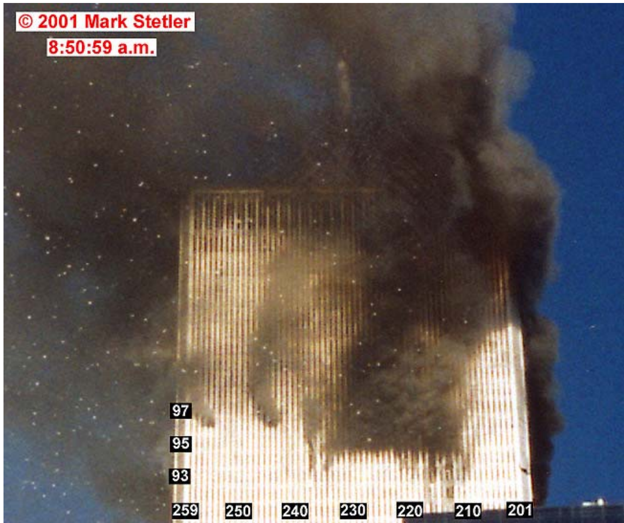
Figure 6-10. Photograph showing the east face of WTC 1 recorded at 8:50:59 a.m. Column and floor numbers have been added.
