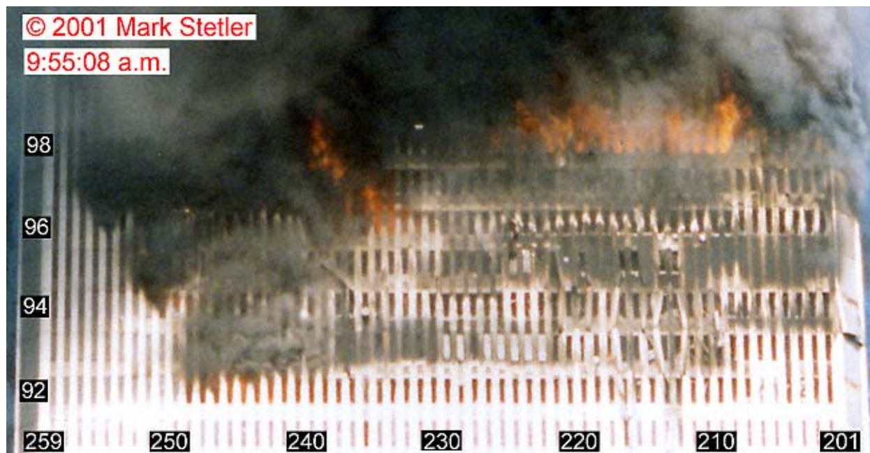
Figure 8-59. This photograph shows the east face of WTC 1 at 9:55:08 a.m. The original has been rotated, cropped, and enhanced. Column and floor number have been added.
