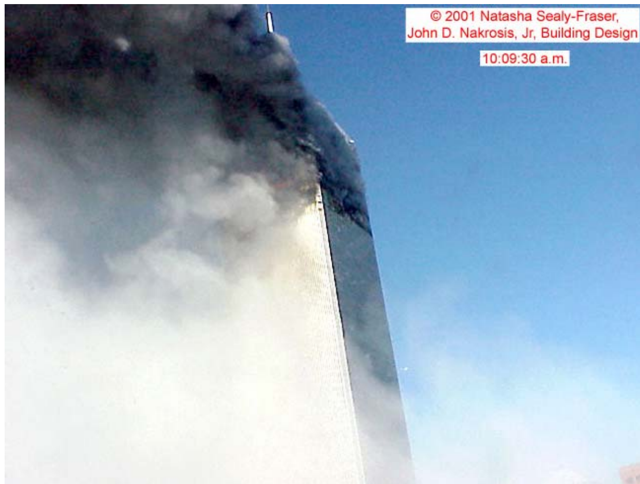
Figure 8-85. This photograph shows the east and north faces of WTC 1 at 10:09:30 a.m. The intensity levels have been adjusted.
