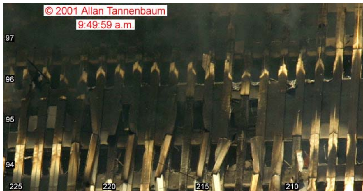
Figure 5-10. This cropped photograph shows a portion of the east face of WTC 1 at 9:49:59 a.m. The image has been rotated and enhanced by adjusting the intensity levels. A number of carets are visible near the tops of windows on the 96th floor. These carets were created during periods of external flaming from adjacent open windows. Column and floor numbers have been added.
