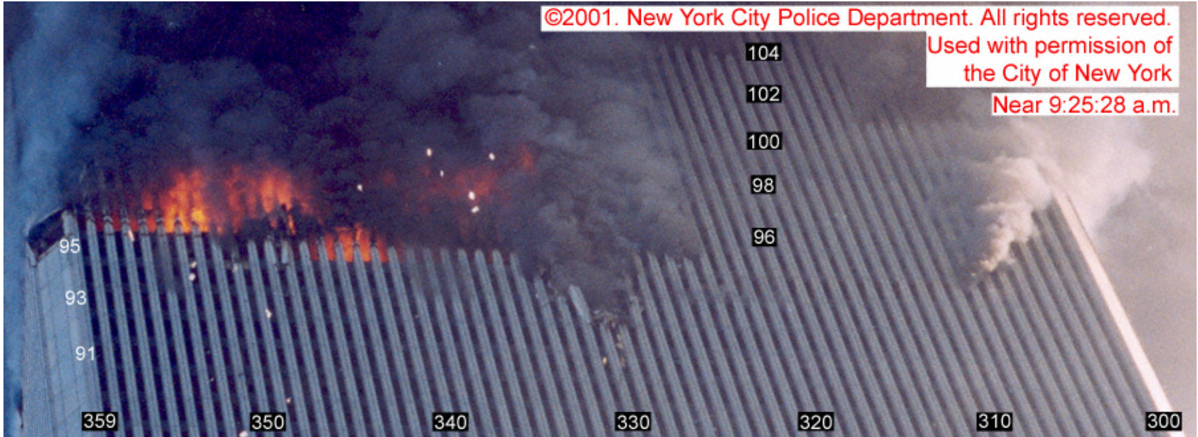
Figure 8-45. This cropped photograph shows the south face of WTC 1. It was taken around 9:25:28 a.m. with an assigned time uncertainty of 15 seconds. The original image has been enhanced and rotated. Column and floor number have been added. A number of pages of paper are present in the photograph.
