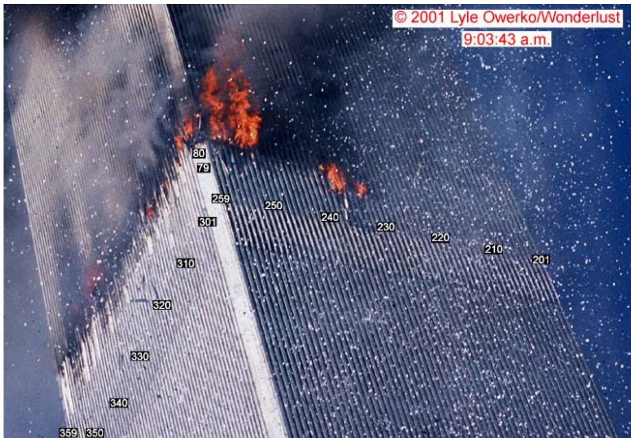
Figure 7-37. This cropped photograph showing WTC 2 from the northeast was taken from the corner of Vesey Street and Church Street at 9:03:43 a.m., i.e., 44 s after the aircraft impact. The intensity levels have been adjusted, and column and floor numbers have been added.
