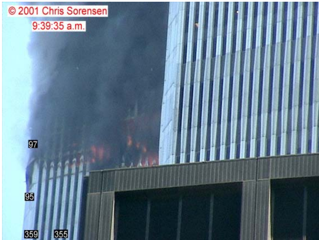
Figure 8-60. This image of the south face of WTC 1 was captured from a video recorded at 9:39:35 a.m. It has been enhanced by adjusting the intensity levels. WTC 1 is on the left behind WTC 2. Another building appears in the foreground. Column and floor numbers have been added.
