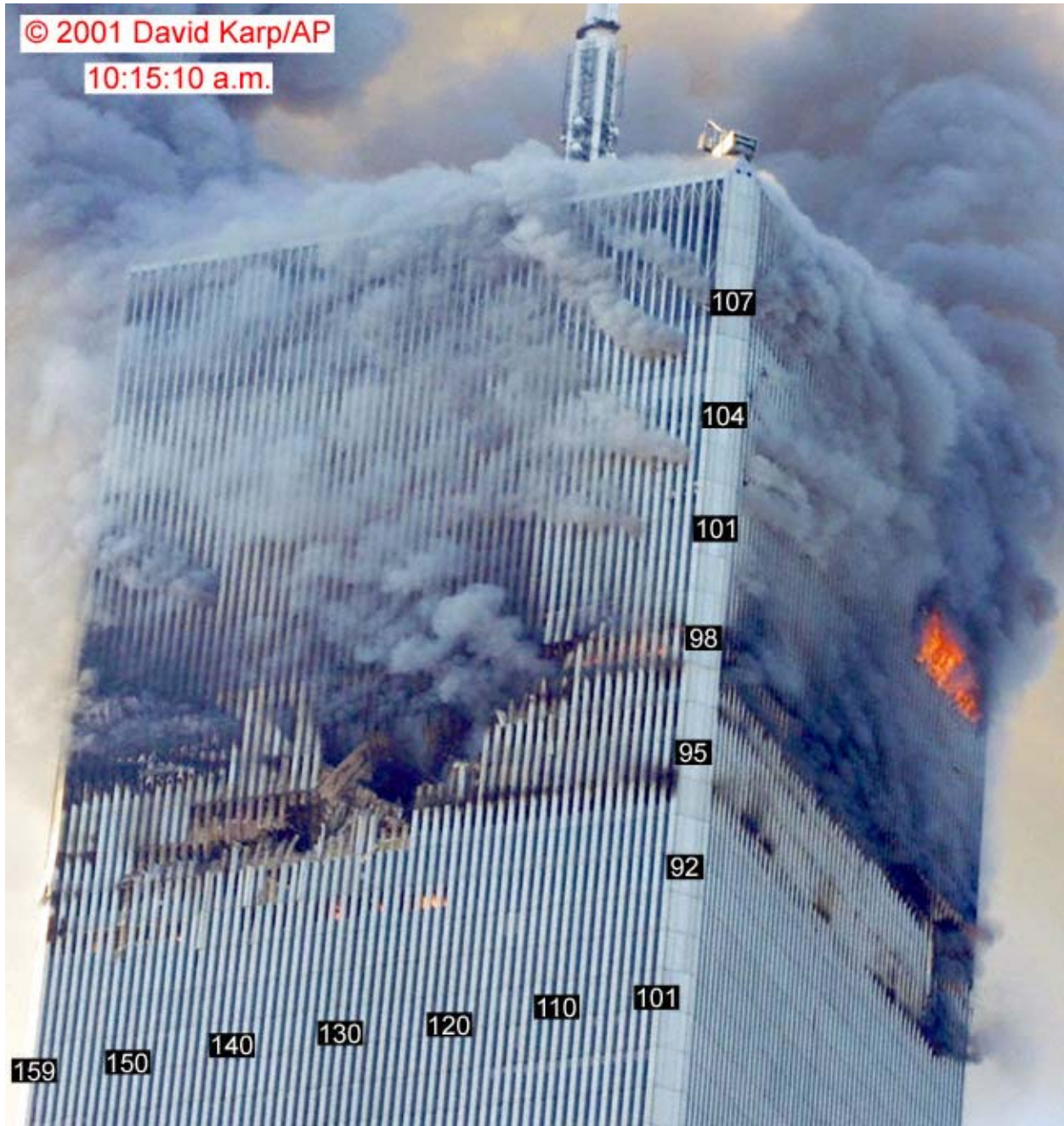
Figure 8-84. This photograph of WTC 1 shows the north and west faces of WTC 1 at 10:15:10 a.m. The image has been cropped and rotated, and the intensity levels have been adjusted. Column and floor numbers have been added.
