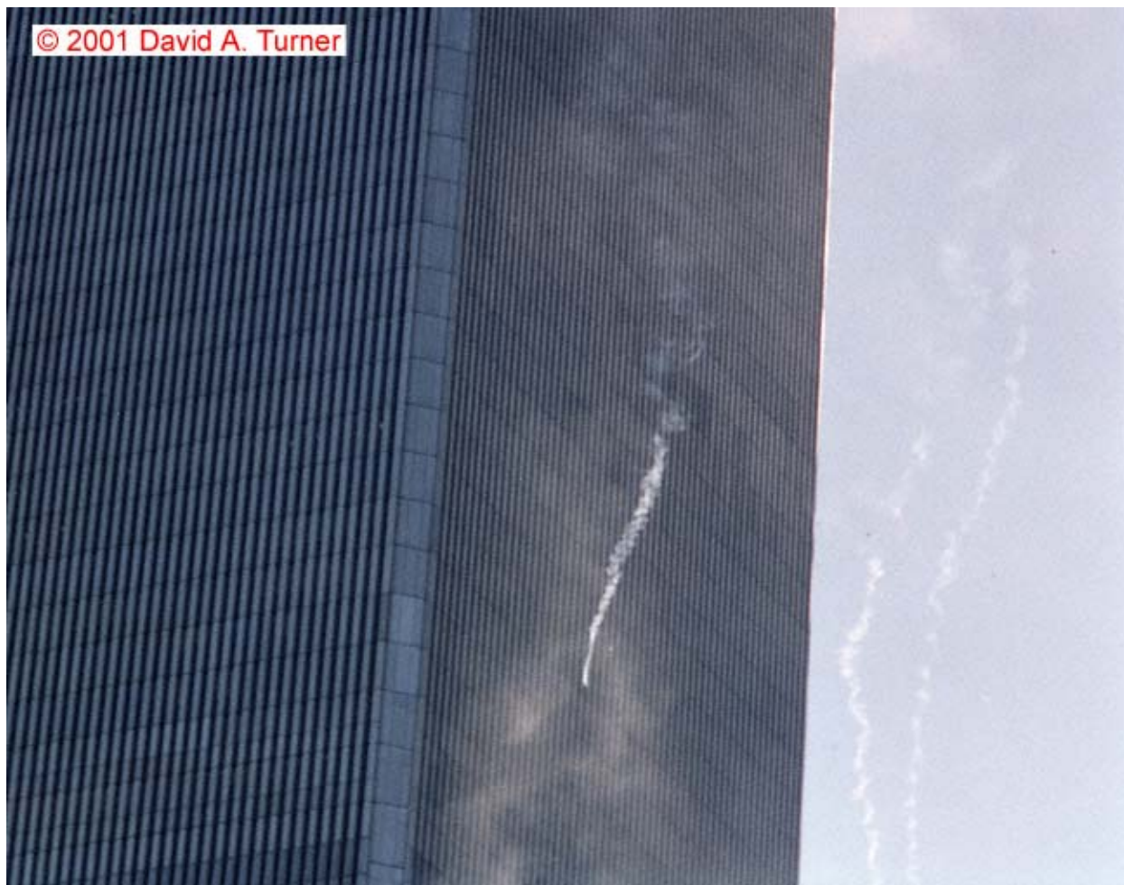
Figure 5-7. This cropped and enhanced photograph shows the west and south faces of WTC 1. An intense streamer is falling near the south face of the tower, and two additional streamers have already fallen through the image to the south. The exact time of this photograph is unknown.
