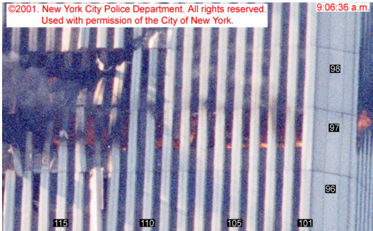
Figure 8-18. Two close-ups of the north face of WTC 1 taken from the photograph in Figure 8-17 show the east and west sides of the face around the 97th floor. The photos have been rotated, enhanced, and column and floor number have been added.
