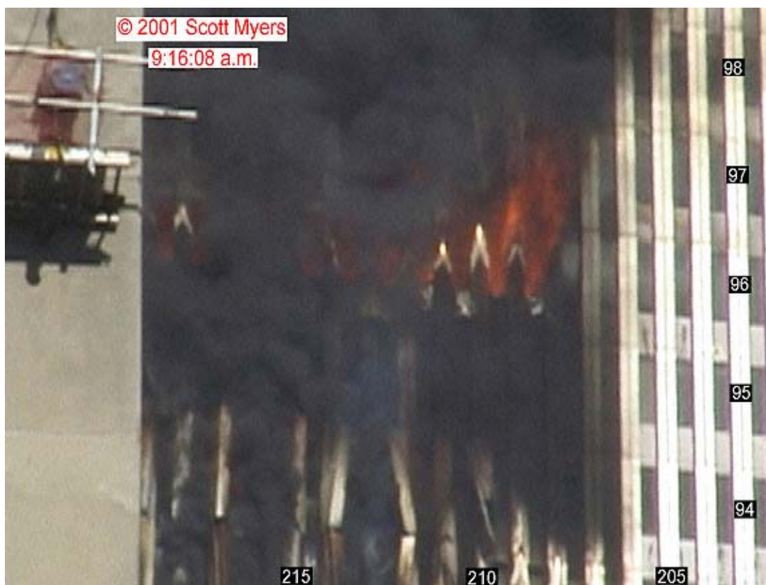
Figure 8-21. A close up of a portion of the east face of WTC 1 is shown. The image is a frame taken from a video recorded at 9:16:08 a.m. Column and floor numbers have been added. The area to the left with the scaffolding is another building in the foreground.
