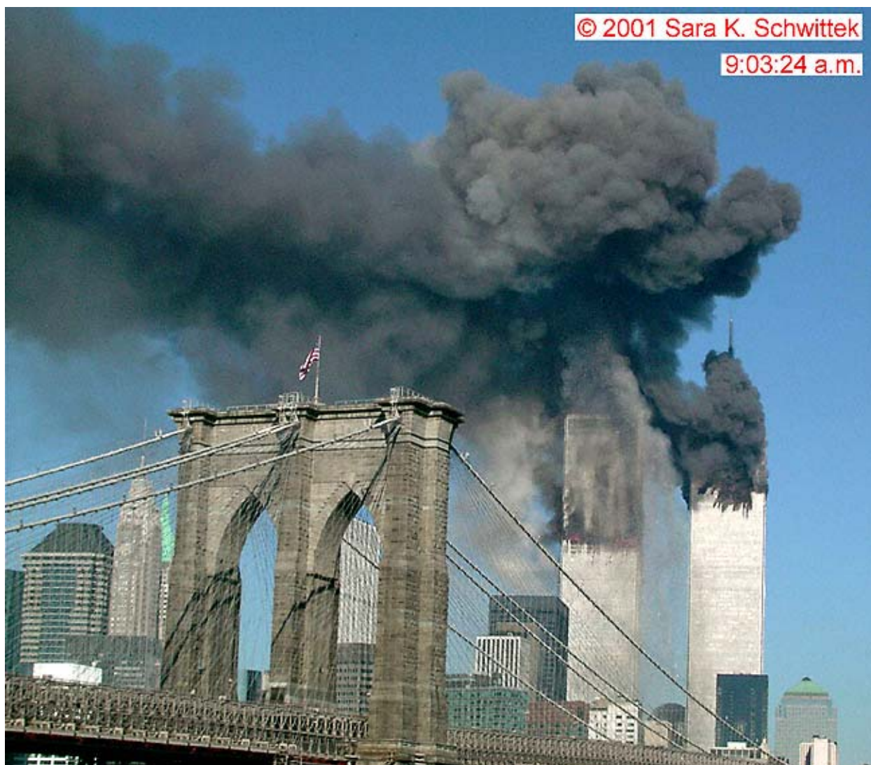
Figure 7-10. This cropped photograph recorded at 9:03:24 a.m., i.e., 25 s after the aircraft impact on WTC 2, shows the nascent thermal created by the fireballs on WTC 2. The intensity levels of the image have been adjusted.
