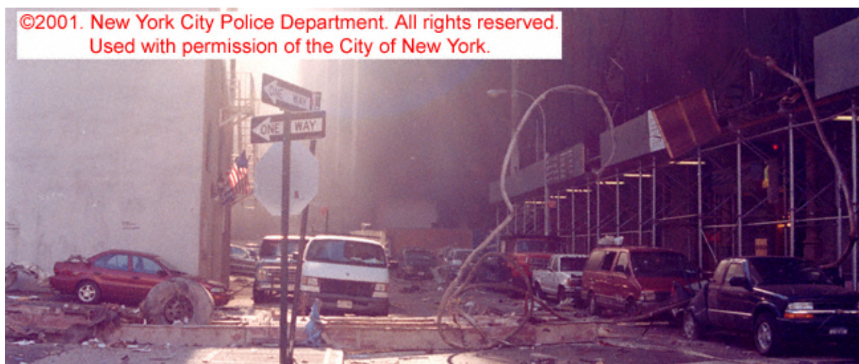
Figure 6-17. This cropped and enhanced photograph shows another view of the three-story steel panel section included in Figure 6–16. A long pipe section attached to the steel rises above both the panel section and the pickup truck to the right. The building on the left is Saint Nicholas Greek Orthodox Church, and the building on the right is 90 West Street.
