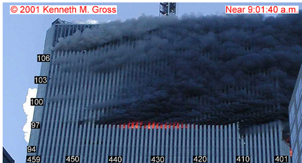
Figure 8-11. Image of the west face of WTC 1 recorded between 9:01:09 a.m. and 9:02:17 a.m. The image has been cropped and rotated, and column and floor numbers have been added.
