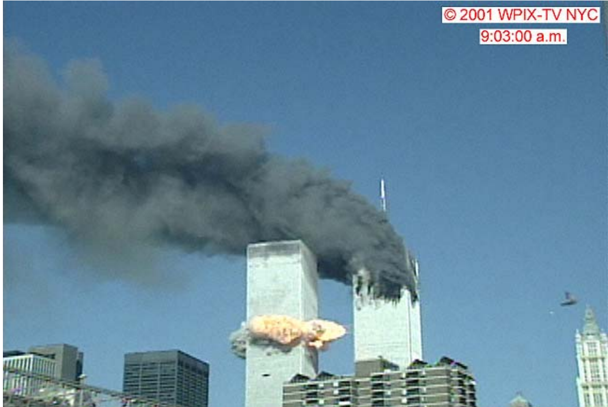
Figure 7-1. The nascent fireballs and dust clouds formed on WTC 2 1.2 s after the aircraft impact on the tower are shown. The image is a frame from a video.
