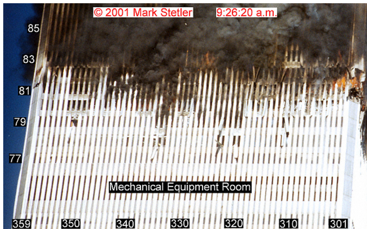
Figure 7-28. A cropped photograph shows the east face of WTC 2 at 9:26:20 a.m. The image has been rotated, and column and floor numbers have been added.
