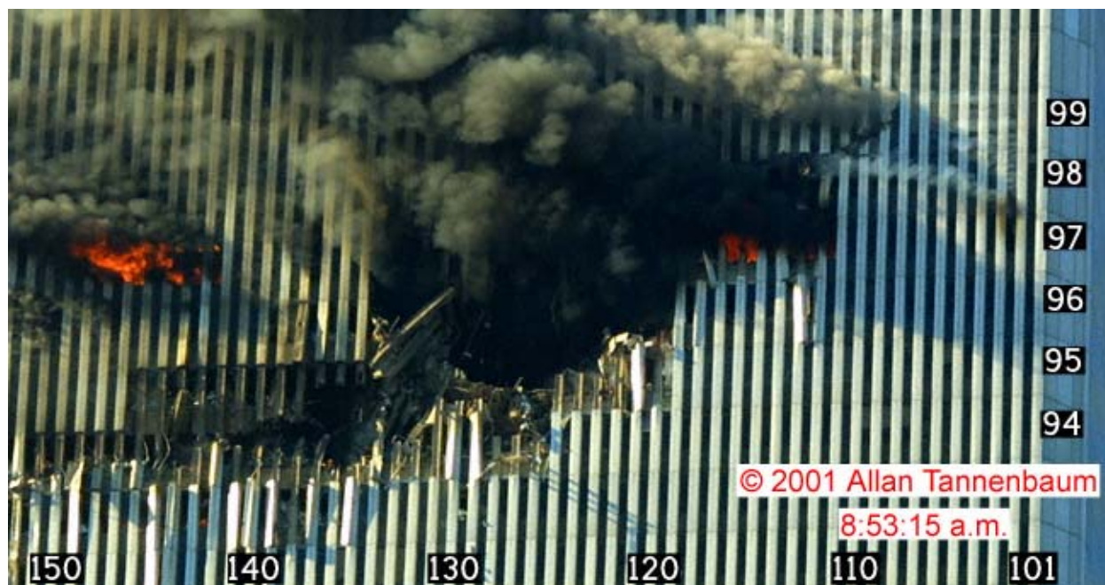
Figure 8-3. An enlargement of a portion of the photograph reproduced in Figure 8-2 showing the north face of WTC 1 at 8:53:15 a.m. is shown. Labels showing floor and column numbers have been added.
