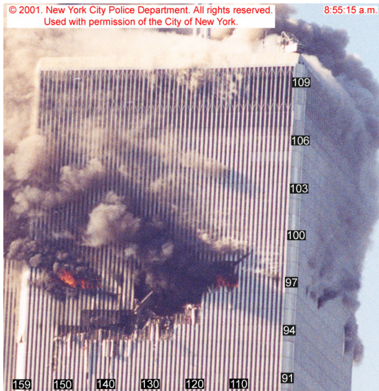
Figure 8-5. A photograph of WTC 1 recorded at 8:55:15 a.m. shows the north and west faces. The original image has been rotated and cropped. Numbers indicating column numbers for the north face and floors have been added.
