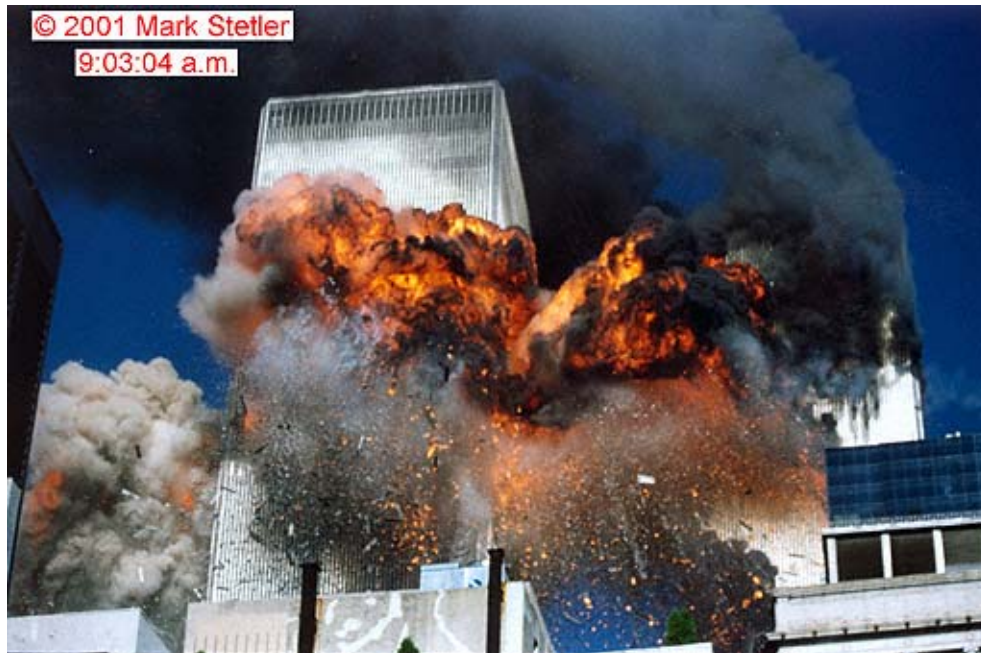
Figure 7-4. An image of the fireball on WTC 2 recorded from just north of due east is shown. The photograph was taken 4.6 s after the aircraft impact on the tower.
