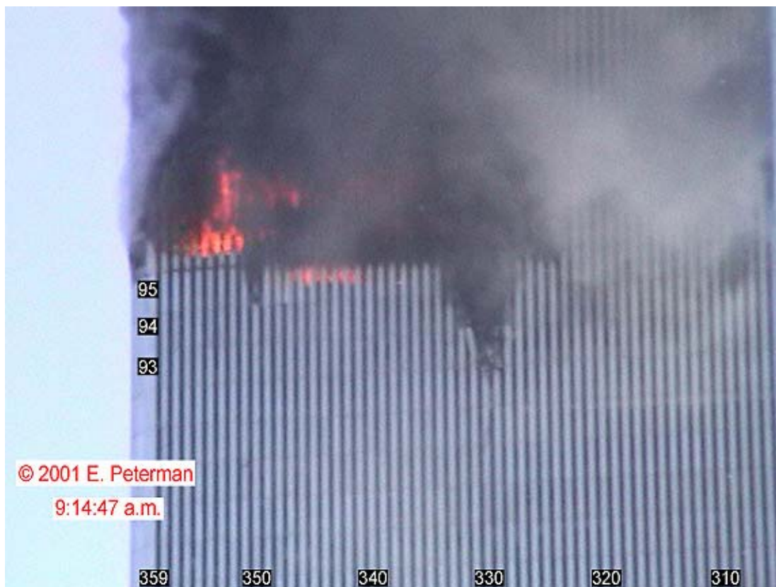
Figure 8-26. This image showing the south face of WTC 1 at 9:14:47 a.m. is a frame taken from a video. Column and floor numbers have been added.
