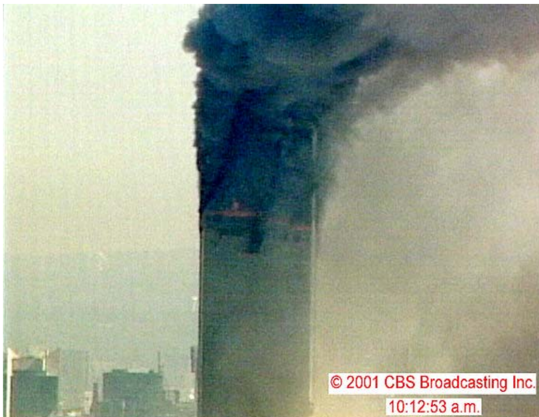
Figure 8-87. This view of the south face of WTC 1 was captured from a video recorded by a news helicopter at 10:12:53 a.m. The image has been enhanced by adjusting the intensity levels.
