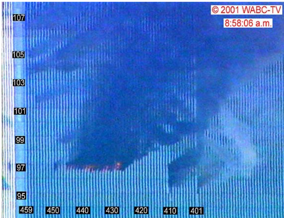
Figure 8-6. This image shows the west face of WTC 1 at 8:58:06 a.m. It is a frame taken from a video shot from a helicopter. Floor and column numbers have been added for WTC1. WTC 2 is in the background on the right side. Smoke is flowing from the damaged area on the corner of the 96th floor.
