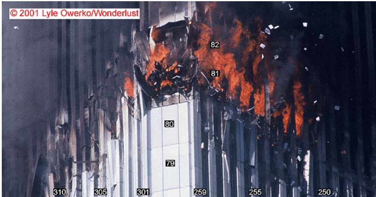
Figure 7-31. This cropped photograph shows the northeast corner of WTC 2. This image was recorded between 9:05 a.m. and 9:19 a.m. Column and floor numbers have been added. The corner aluminum panels on the 81st and 82nd floors have been pushed outward. A large pile of debris is evident in the opening on the 81st floor, and a vertical steel column, numbered 82-300, can be seen on the 82nd floor.
