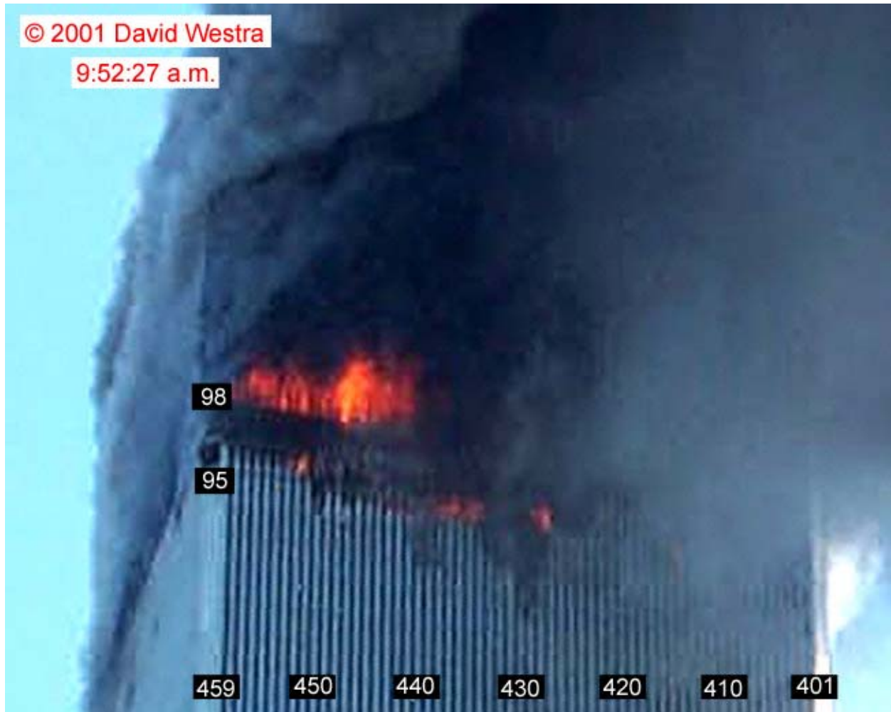
Figure 8-64. This cropped photograph shows the south face of WTC 1 at 9:52:27 a.m. The intensity levels have been adjusted and column and floor numbers have been added.
