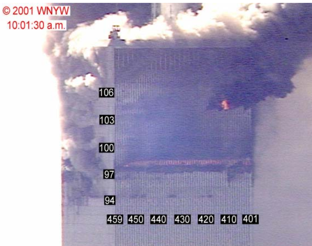
Figure 8-89. This image of the north and west faces of WTC 1 is a frame captured from a video recorded by a news helicopter at 10:01:30 a.m. The image has been enhanced by adjusting the intensity range, and some areas are saturated. Column and floor numbers have been added.
