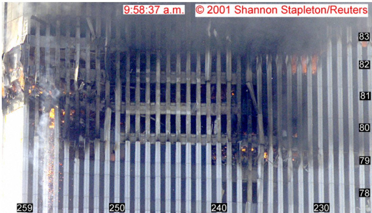
Figure 7-32. A cropped and enhanced photograph of WTC 2 taken at 9:58:37 a.m. shows the east side of the north face. Piles of debris are evident on the 80th and 81st floors at the northeast corner and on the 79th floor to the right of column 241. The “cold” spot extends over the 80th to 82nd floors from column 238 to 249.
