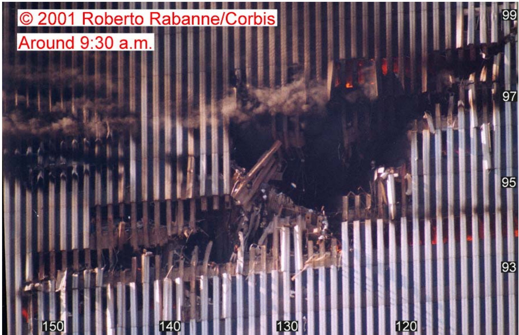
Figure 6-5. A close-up image of the north face of WTC 1 recorded around 9:30 a.m. shows the area of WTC 1 where the aircraft impacted. Column and floor numbers have been added.
