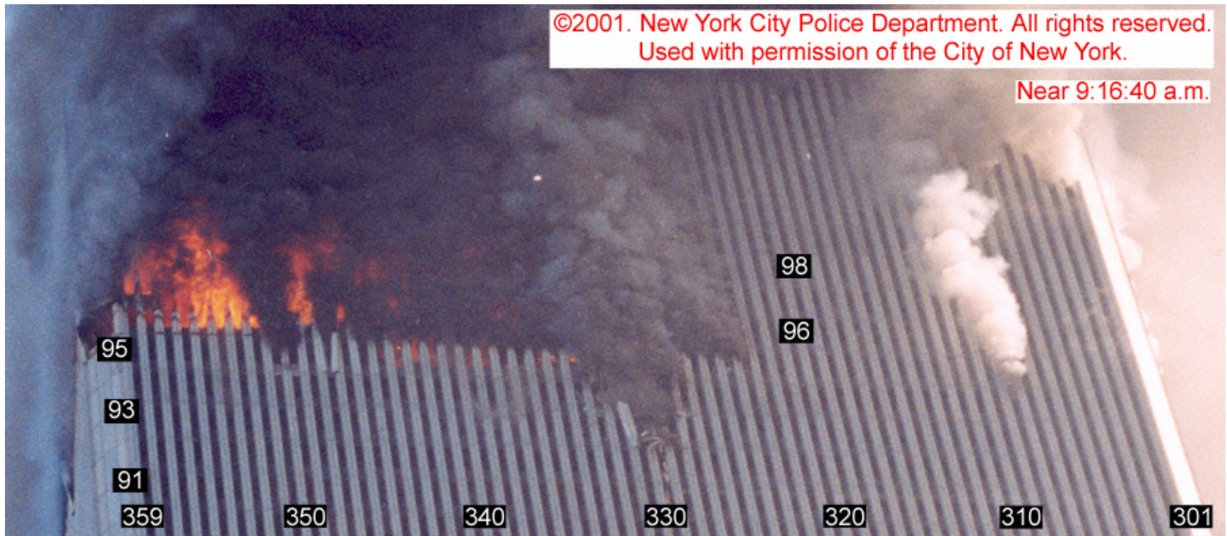
Figure 8-27. This image of the south face has been cropped from a high-resolution photograph. There is a 35 s uncertainty in the assigned time of 9:16:40 a.m. The image has been enhanced and rotated. Column and floor numbers have been added.
