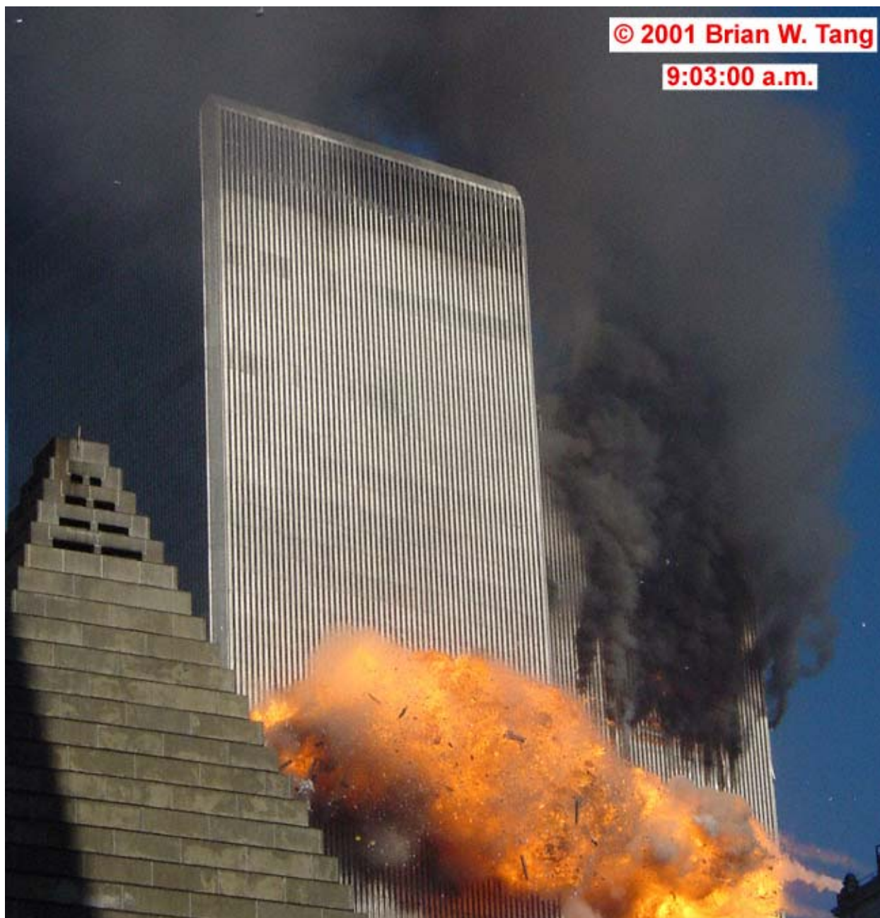
Figure 7-2. This cropped photograph shows the fireball formed on the east face of WTC 2 following the aircraft impact that took place 1.1 s earlier. The east face of WTC 1 is visible in the background
