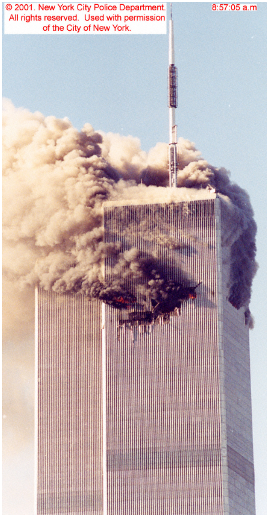
Figure 4-5. This cropped photograph shows a view of WTC 1 and WTC 2 taken from the north northwest at 8:57:05 a.m. The intensity levels have been adjusted.
