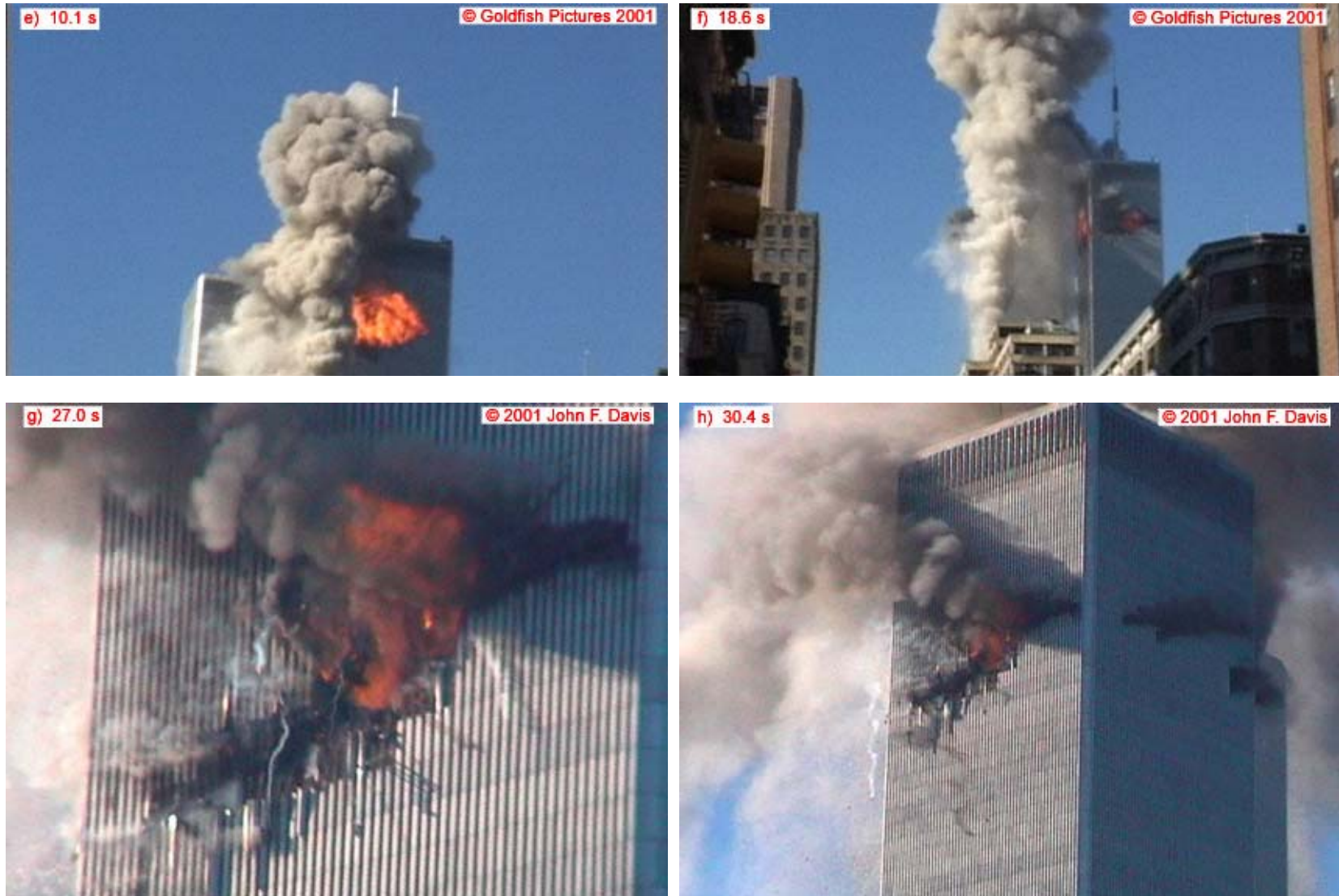
Figure 6–1. A series of frames from videos shows American Airlines Flight 11 striking WTC 1 and the immediate aftermath. Times relative to the aircraft impact time are shown in the upper left-hand corner (continued).
