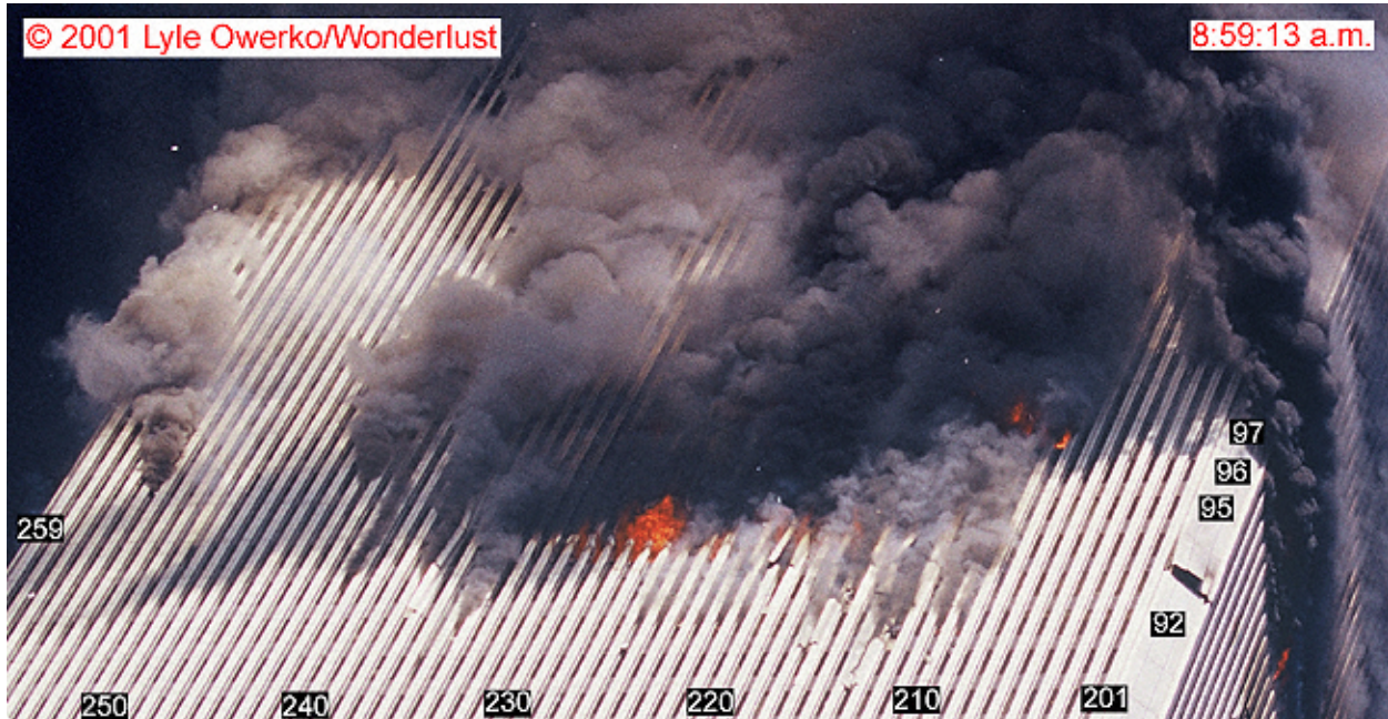
Figure 8-9. This view of the east face of WTC 1 was recorded at 8:59:13 a.m. The original image has been rotated and cropped. Column and floor numbers have been added.
