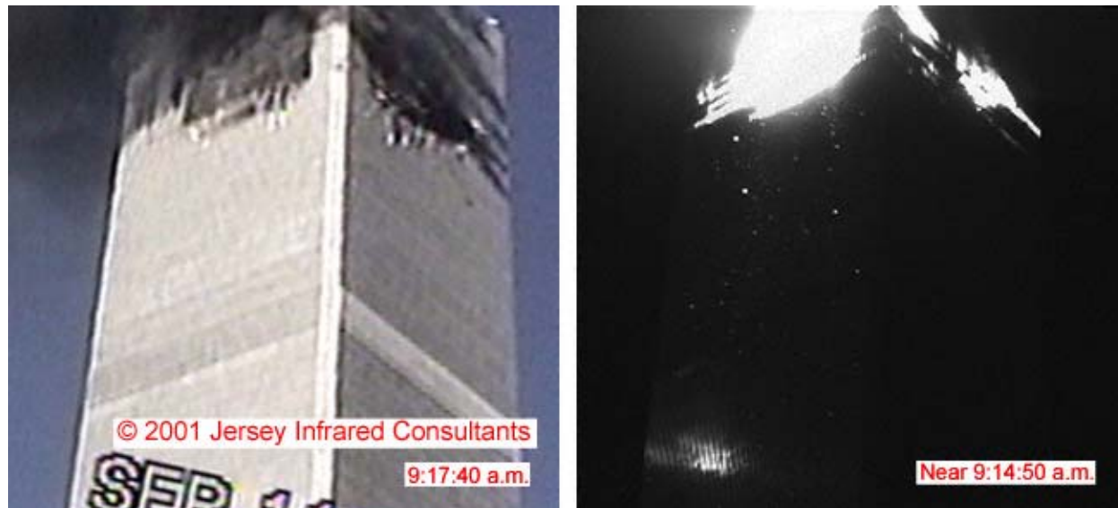
Figure 8-23. A frame from a standard video camera (left) and an image from an infrared camera (right) showing the north and east faces of WTC 1 are compared. The video frame was shot at 9:17:40 a.m., and the infrared image was taken around 9:14:50 a.m. (an uncertainty of 15 s has been assigned). The infrared image intensity levels were adjusted. The video frame has been rotated and sized to match the infrared image.
