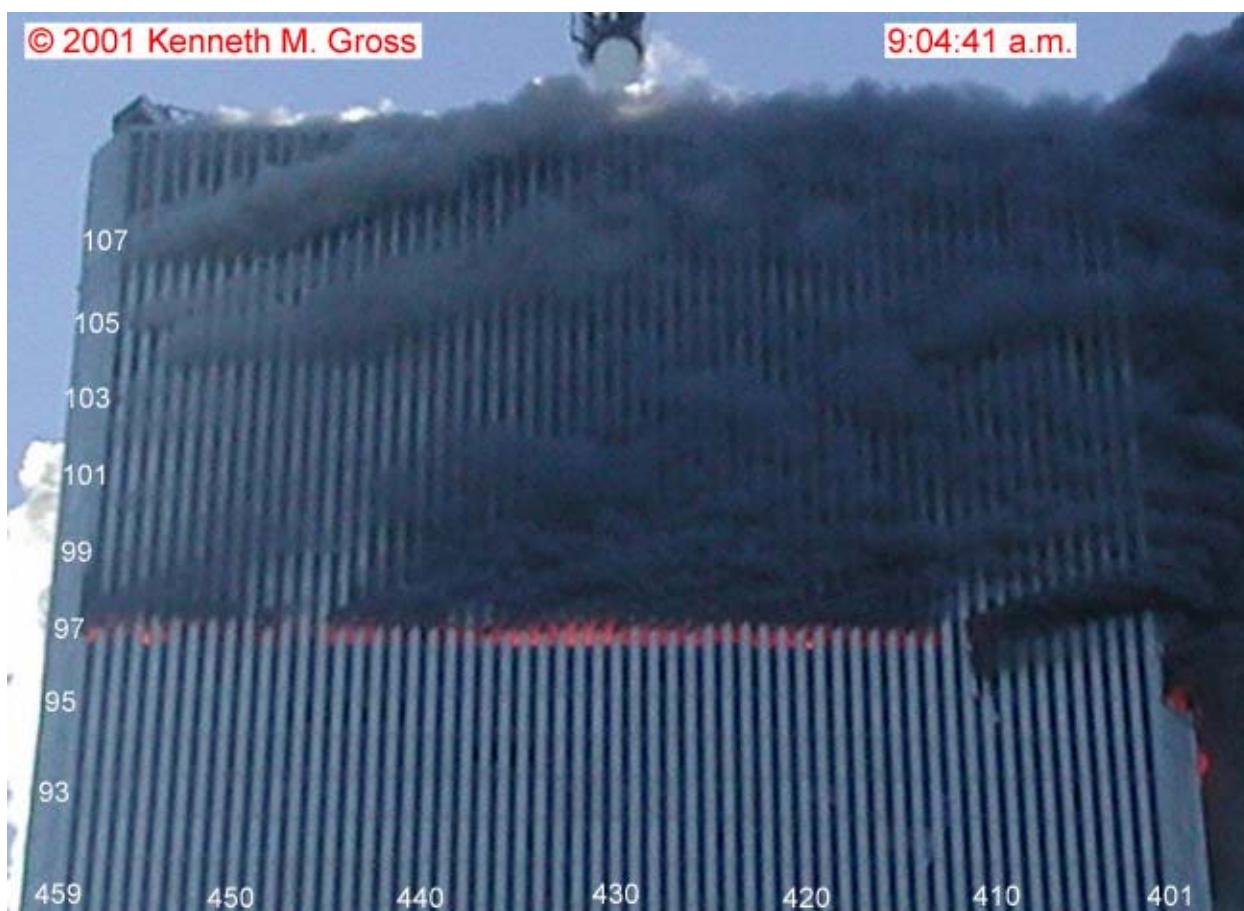
Figure 8-28. A cropped photograph of the west face of WTC 1 taken at 9:04:41 a.m. is shown. The image has been enhanced and rotated. Window and floor numbers have been added. A streamer can be seen falling near the bottom of the image at column 414.
