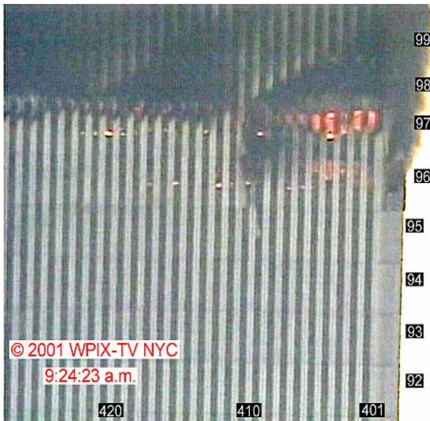
Figure 8-48. This image of a portion of the west face of WTC 1 is a frame captured from a video recorded by a news helicopter at 9:24:23 a.m. The image has been enhanced by adjusting the intensity range, and the area to the right of the tower is saturated. Column and floor numbers have been added.
