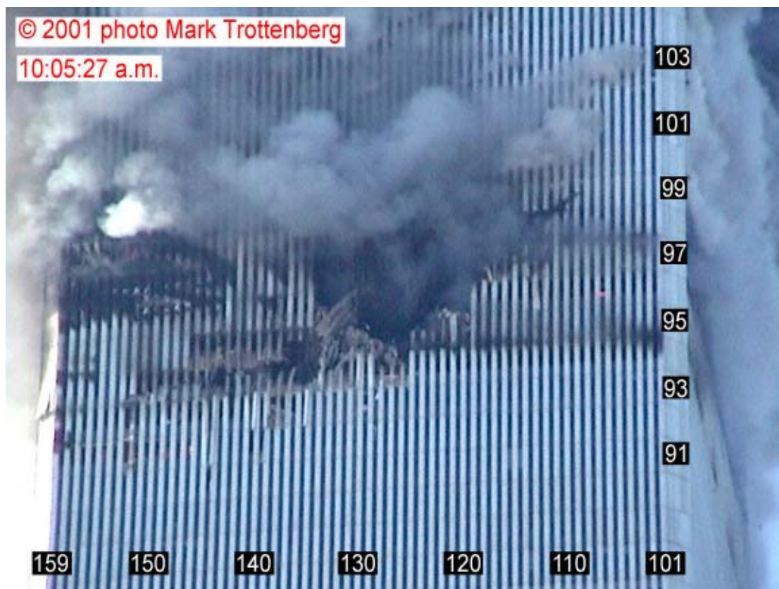
Figure 8-81. This view of the north face of WTC 1 was captured from a video recorded at 10:05:27 a.m. The image has been enhanced by adjusting the intensity levels. Column and floor numbers have been added.
