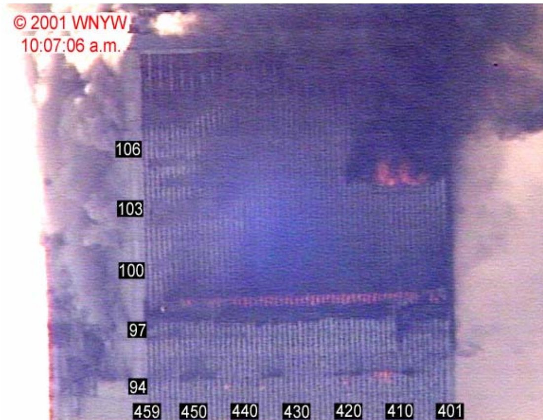
Figure 8-90. This image of the north and west faces of WTC 1 is a frame captured from a video recorded by a news helicopter at 10:07:06 a.m. The image has been enhanced by adjusting the intensity range, and some areas are saturated. Column and floor numbers have been added.
