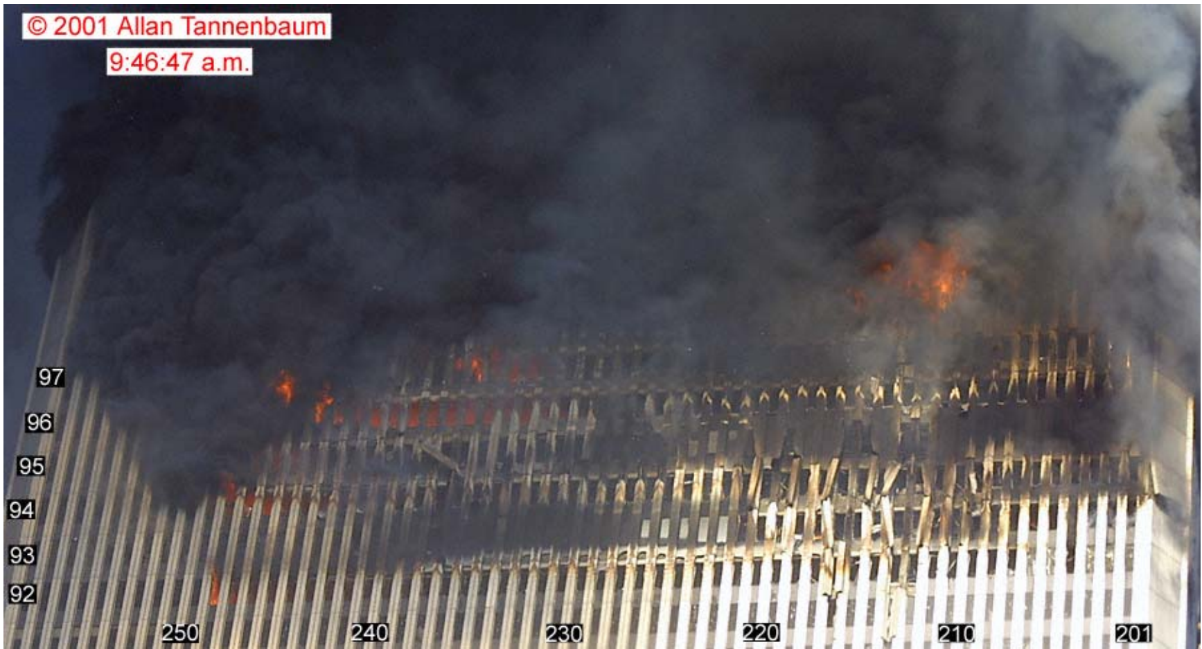
Figure 8-58. This image shows the east face of WTC 1 at 9:46:47 a.m. The original image has been cropped, rotated, and enhanced. Column and floor numbers have been added.
