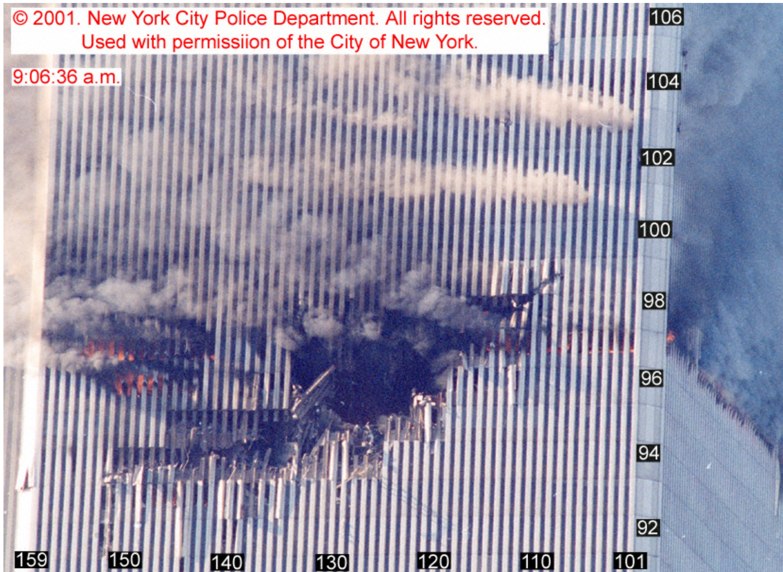
Figure 8-17. A photograph of the north face of WTC 1 recorded at 9:06:36 a.m. is shown. The image has been cropped, rotated, and enhanced. Column and floor numbers have been added.
