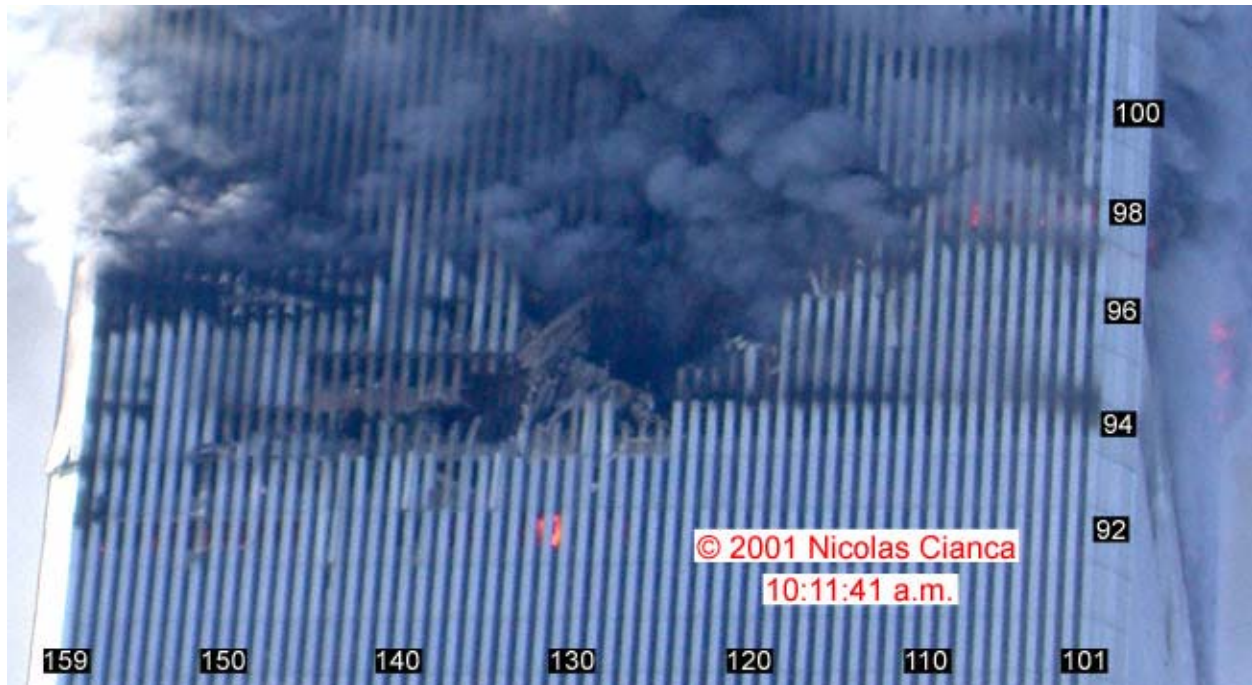
Figure 8-83. This photograph shows the north face of WTC 1 at 10:11:41 a.m. The original image has been cropped, rotated, and adjusted for intensity levels. Column and floor numbers have been added
