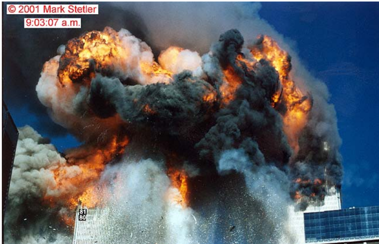
Figure 7-7. An image of WTC 2 recorded from just north of due east is shown. The photograph was taken 7.9 s after the aircraft impact on the tower. The locations of the 80th and 81st floors are identified
