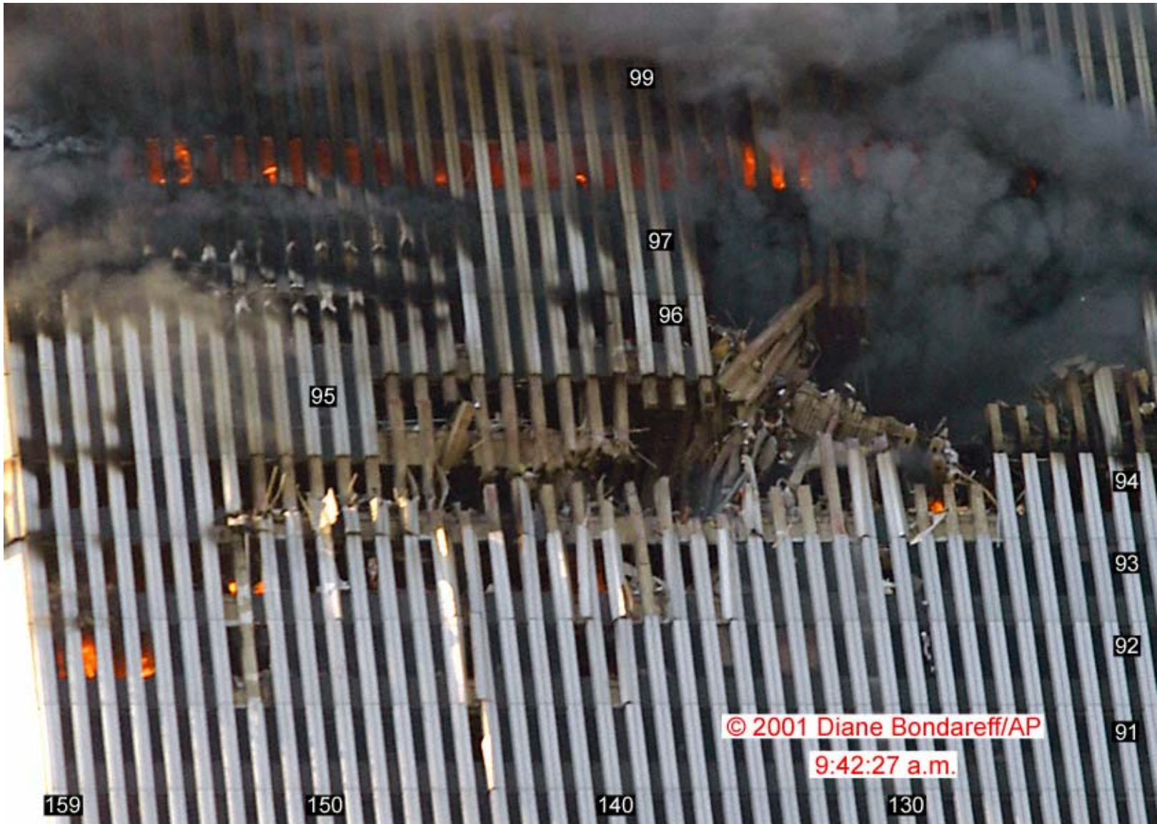
Figure 8-53. This sharp photograph shows the eastern portion of the north face of WTC 1 at 9:42:27 a.m. The original version has been cropped and enhanced. Column and floor numbers have been added.
