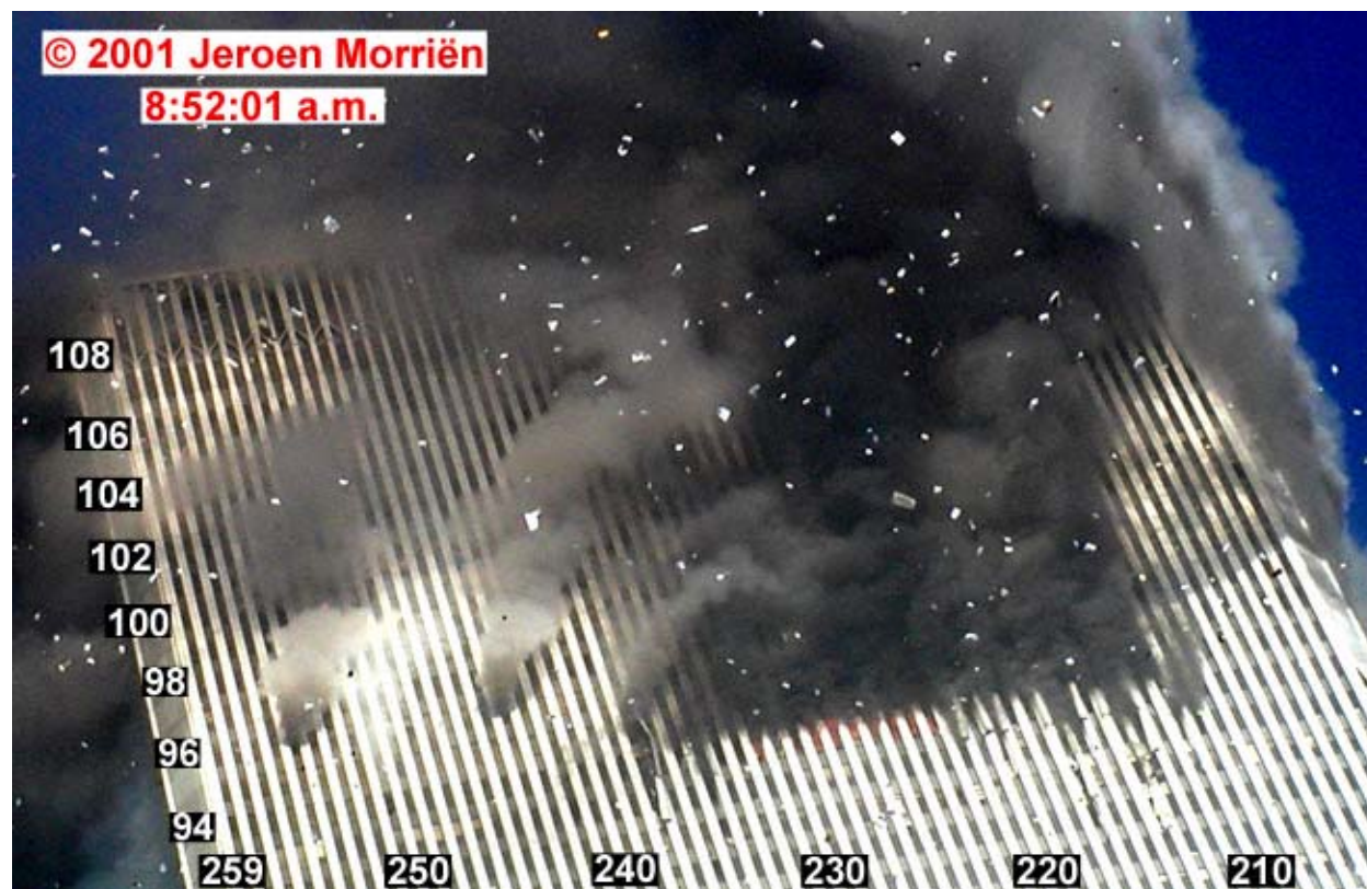
Figure 6-11. Photograph of the east face of WTC 1 taken at 8:52:01 a.m. The photograph has been enhanced and cropped. Floor numbers are indicated along the left edge of the building and column numbers along the bottom of the photo.
