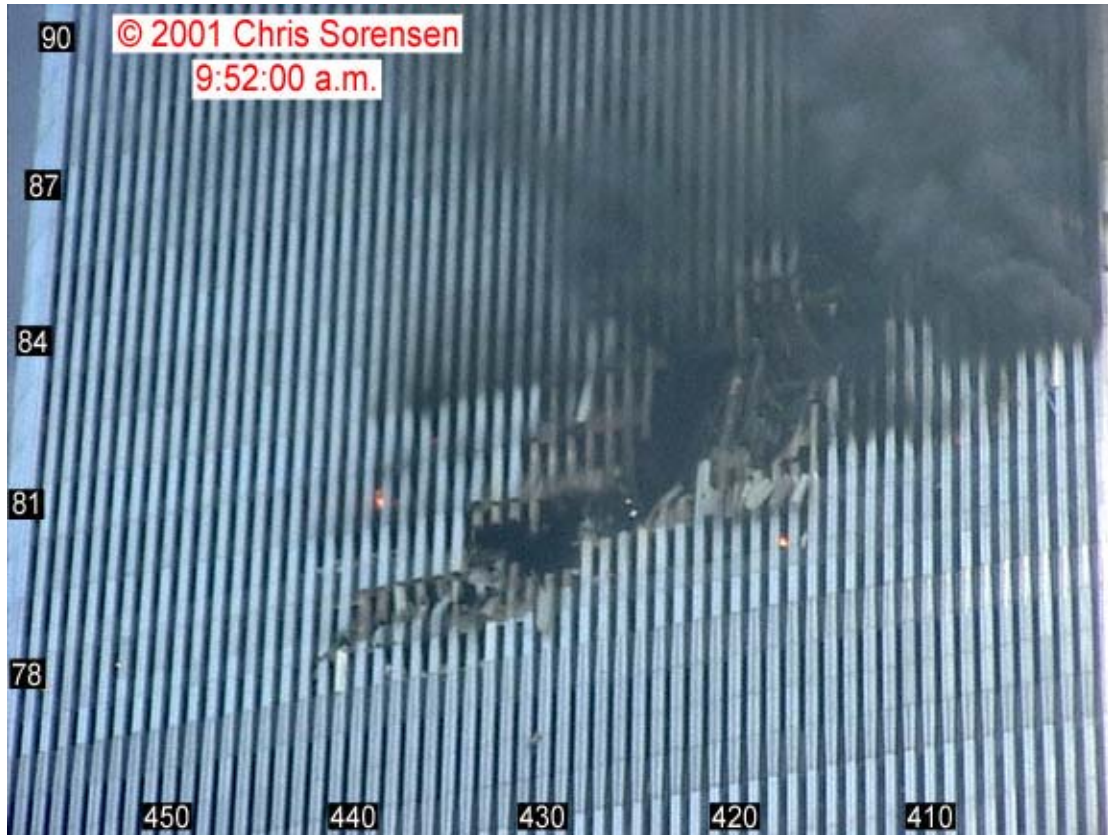
Figure 9-68. This view of the south face of WTC 2 was taken from a video recorded at 9:52:00 a.m. The intensity levels have been adjusted, and column and floor numbers have been added.
