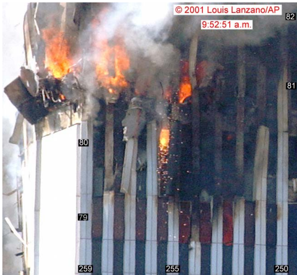
Figure 9-72. This image is a blow-up of a portion of Figure 9-71 showing the north face of WTC 2 around window 80-255 at 9:52:51 a.m. Column and floor numbers have been added.
