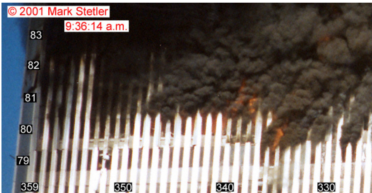
Figure 9-44. These two images show blow-ups of the north and south sides of the east face of WTC 2 taken from the photograph included in Figure 9-43, which was shot at 9:36:14 a.m. Column and floor numbers have been added
