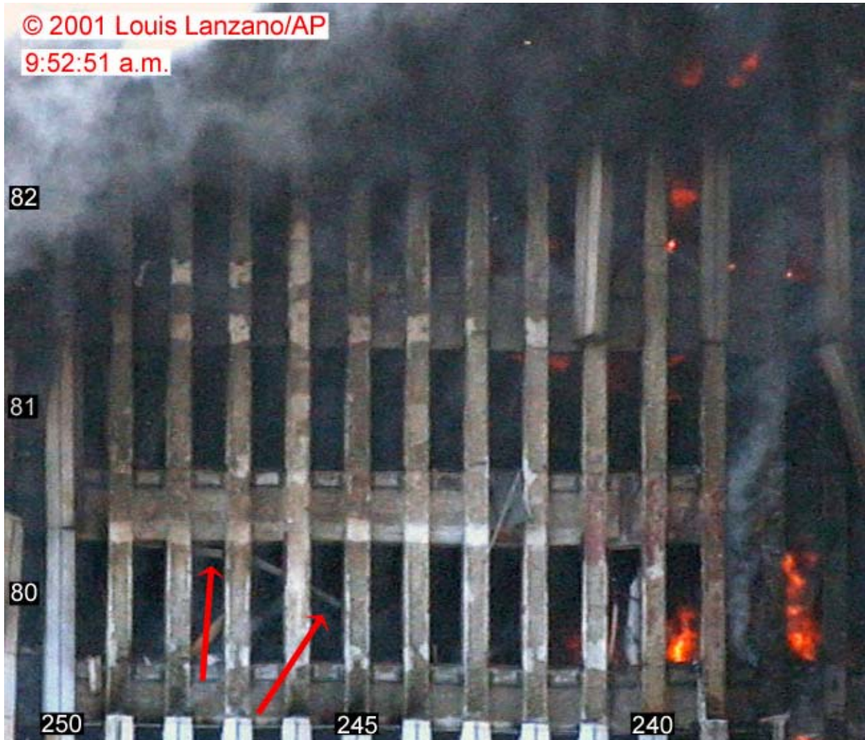
Figure 9-73. This image is a blowup of a portion of Figure 9–71 showing the cold spot on the north face of WTC 2 at 9:52:51 a.m. Column and floor numbers have been added. The arrows highlight a hanging object visible through open windows on the 80th floor.
