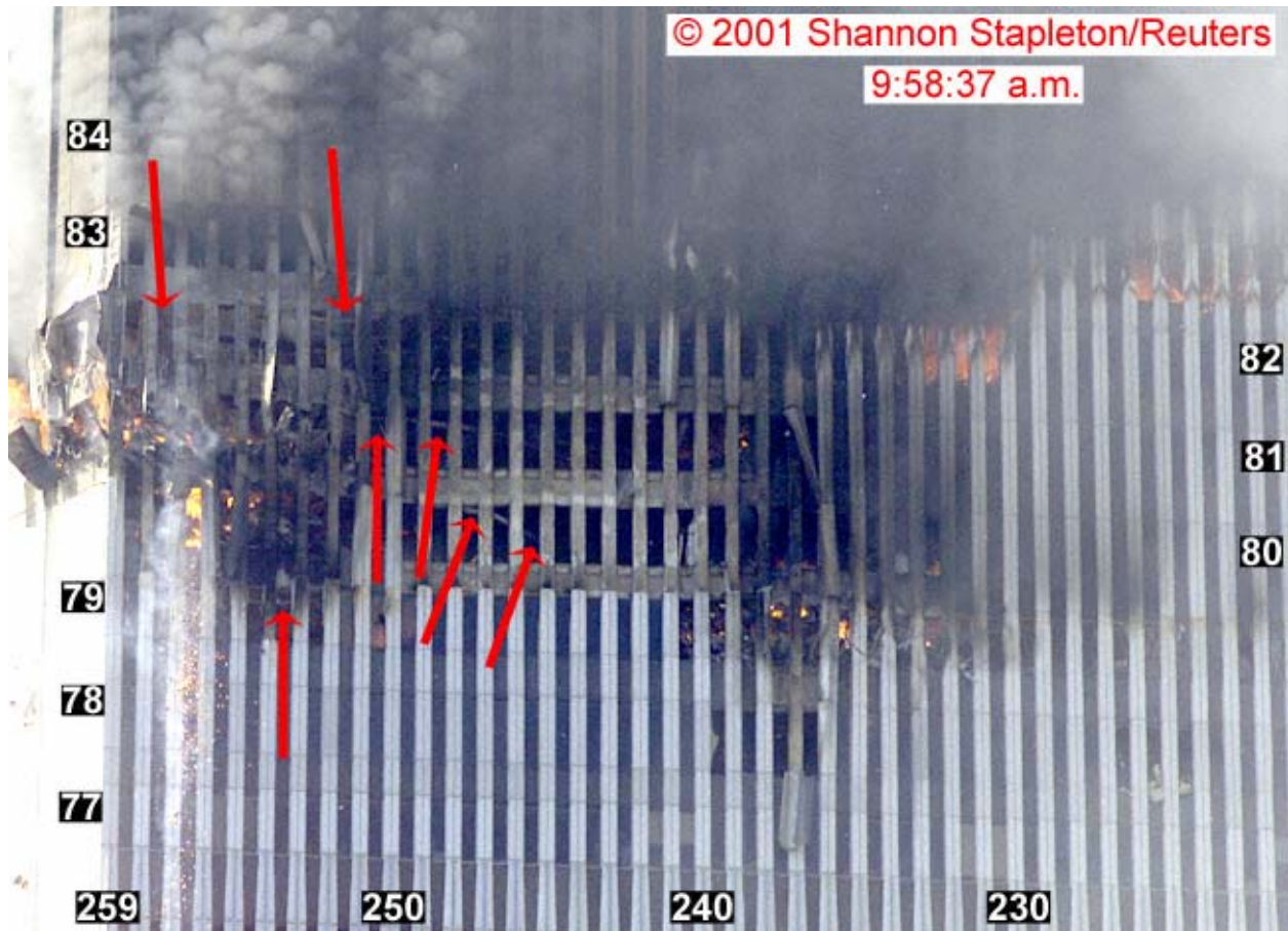
Figure 9-78. This cropped photograph shows the north face of WTC 2 at 9:58:37 a.m. The intensity levels have been adjusted, and column and floor numbers have been added. Arrows highlight hanging objects visible through open windows on the 79th, 80th, 81st, and 82nd floors.
