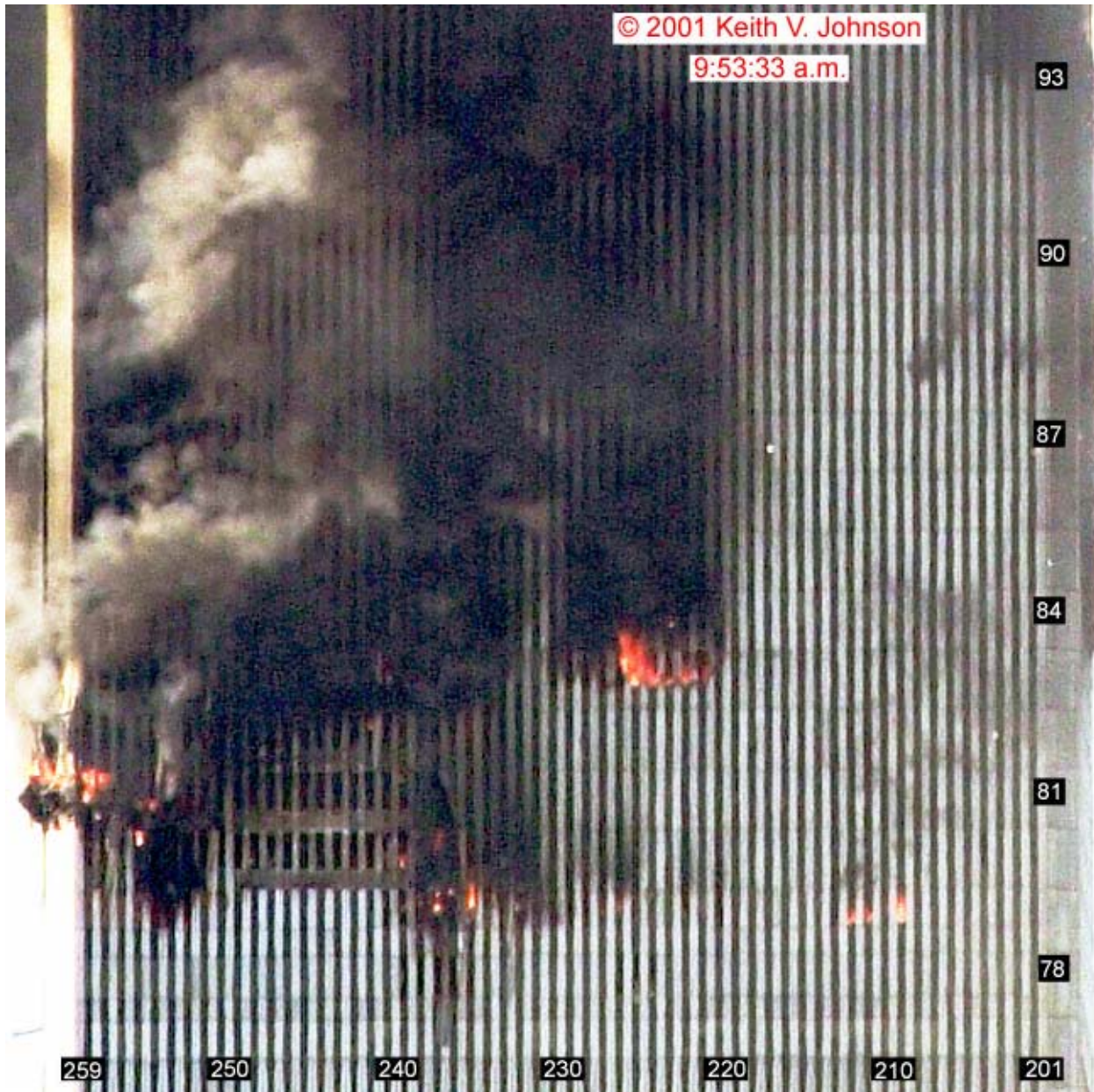
Figure 9-74. This cropped photograph shows the north face of WTC 2 at 9:53:33 a.m. The intensity range has been adjusted, and column and floor numbers have been added.
