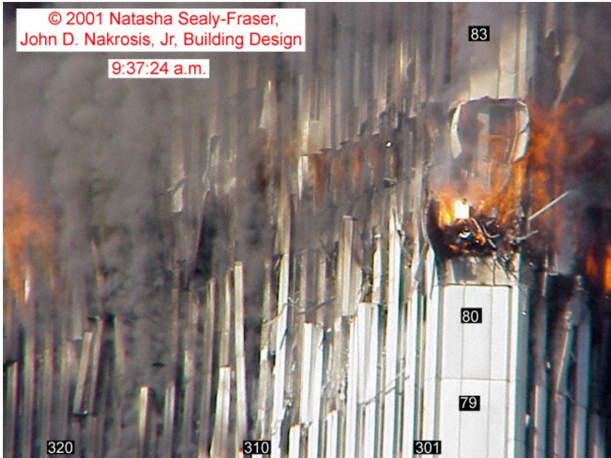
Figure 9-45. This photograph was taken from the northeast at 9:37:24 a.m. and shows portions of the north and east faces of WTC 2. The intensity levels have been adjusted, and column and floor numbers have been added.
