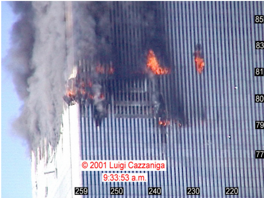
Figure 9-37. This frame taken from a video shows the north face of WTC 2 at 9:33:53 a.m. The intensity levels of the image have been adjusted, and column and floor numbers have been added.
