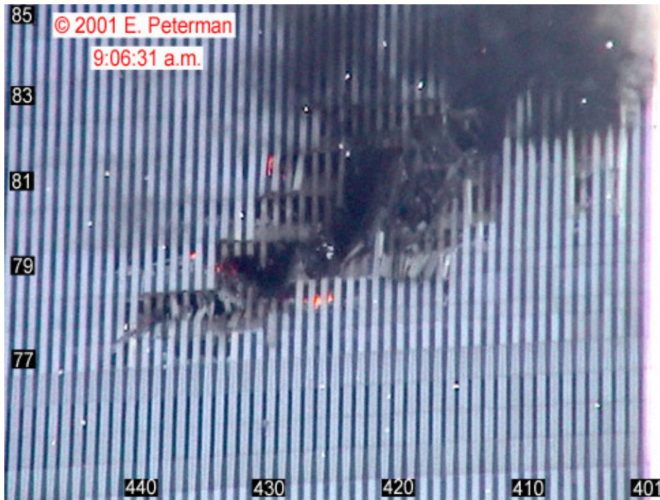
Figure 9-10. This image showing the south face of WTC 2 is a frame captured from a video recorded at 9:06:31 a.m. It has been enhanced by adjusting the intensity levels, and column and floor numbers have been added.
