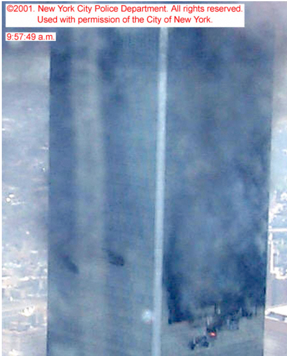
Figure 9-86. This cropped photograph showing the west and south faces of WTC 2 was shot from a helicopter at 9:57:49 a.m. The intensity levels have been adjusted.
