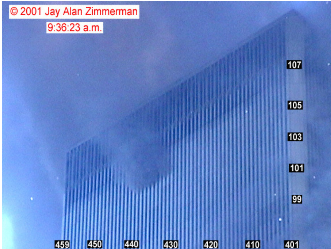
Figure 9-54. This image is taken from a video shot from the southeast and shows the upper portion of the south face of WTC 2 at 9:36:23 a.m. The intensity levels have been adjusted, and column and floor numbers have been added.
