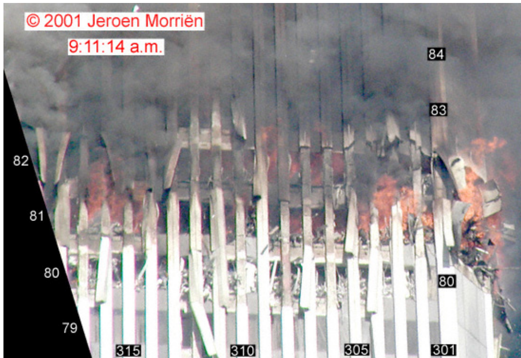
Figure 9-13. This photograph shows the northern portion of the east face of WTC 2 at 9:11:14 a.m. The image has been cropped and rotated, and the intensity levels have been adjusted. Column and floor number have been added.
