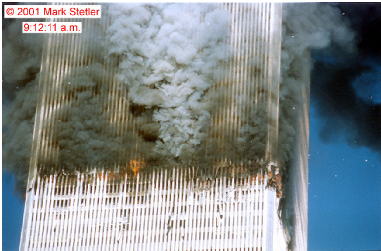
Figure 9-14. This photograph showing the east face of WTC 2 was recorded at 9:12:11 a.m.
