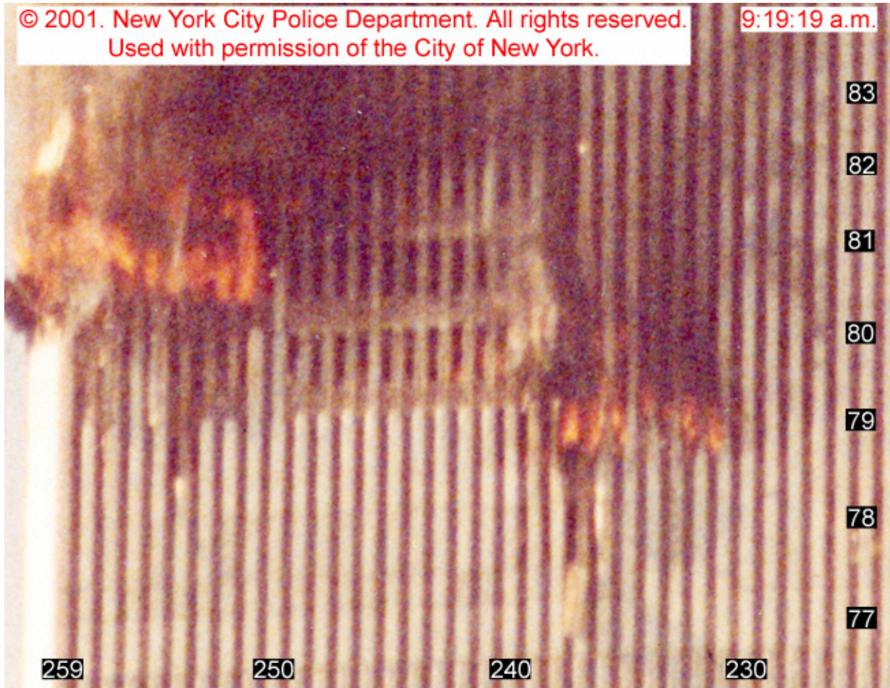
Figure 9-24. This cropped photograph shows the north face of WTC 2 at 9:19:19 a.m. The image has been enhanced by adjusting the intensity levels, and column and floor numbers have been added.
