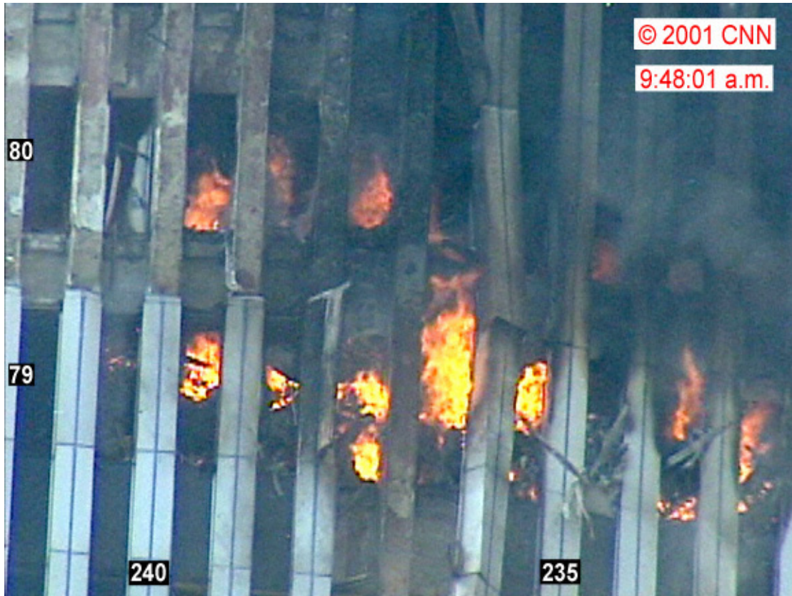
Figure 9-64. This close-up image of the north face of WTC 2 was captured from a video recorded at 9:48:01 a.m. The intensity levels have been adjusted, and column and floor numbers have been added.
