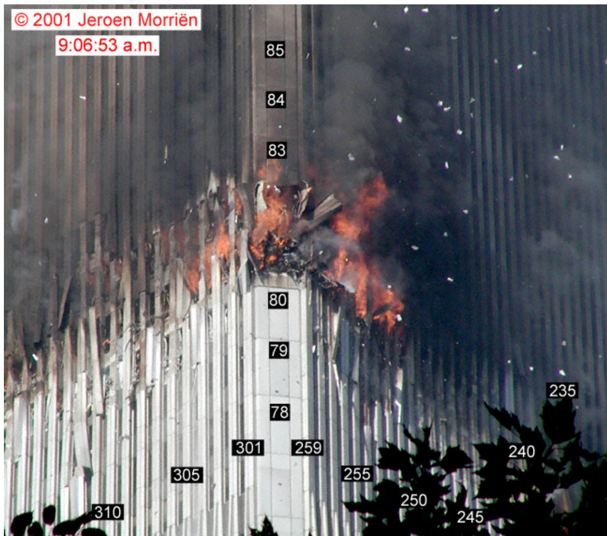
Figure 9-9. This cropped photograph showing the northeast corner of WTC 2 was taken at 9:06:53 a.m. The image has been enhanced by adjusting the intensity levels. Column and floor numbers have been added.
