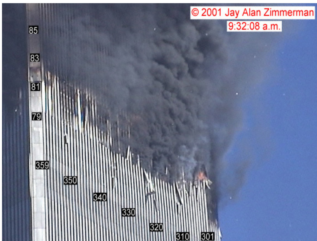
Figure 9-39. This view of the east face of WTC 2 is a frame from a video taken at 9:32:08 a.m. Column and floor numbers have been added. The northeast corner of WTC 1 is visible in the background.
