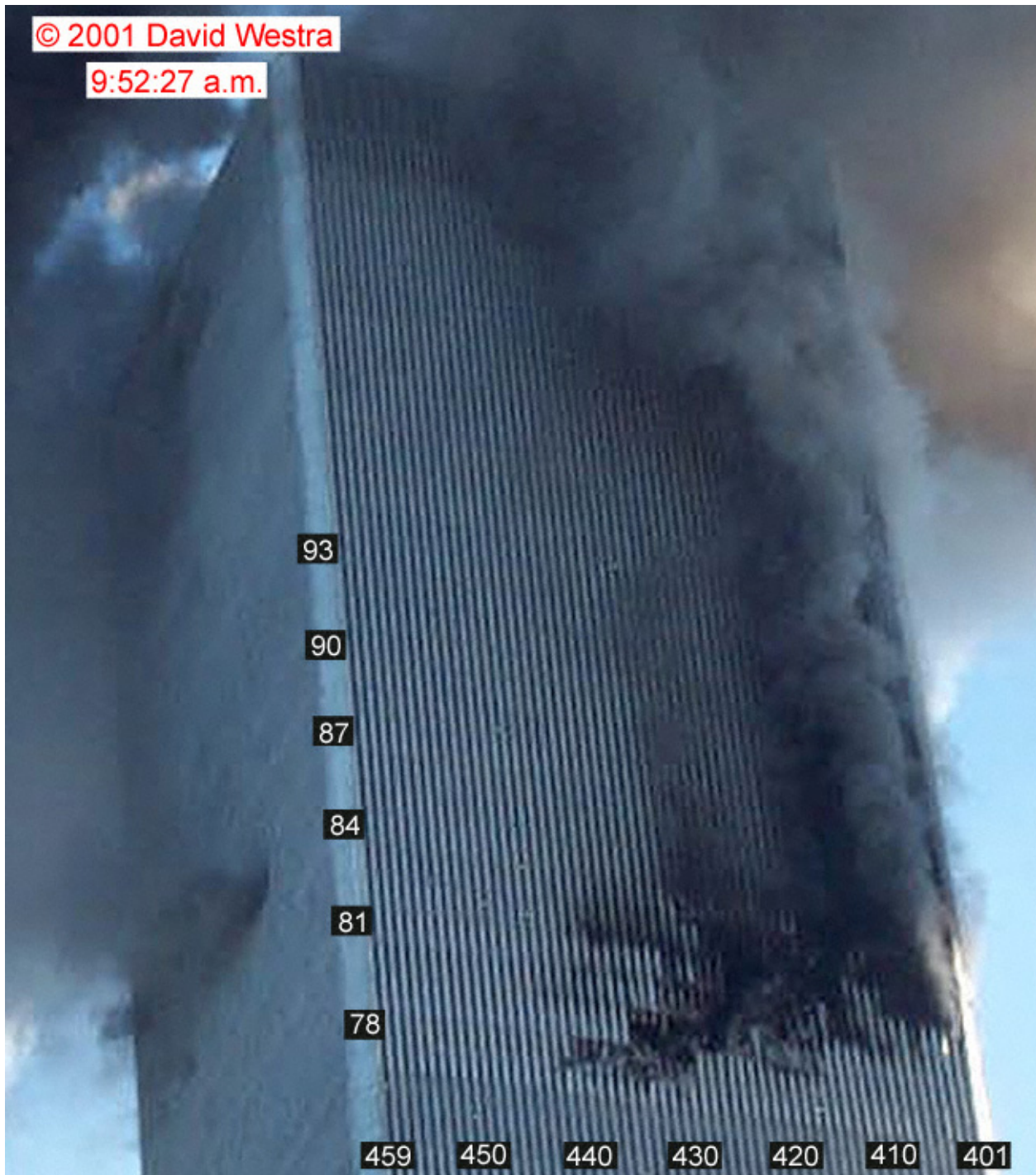
Figure 9-84. This cropped photograph shows the south and west faces of WTC 2 at 9:52:27 a.m. The intensity levels have been adjusted, and floor numbers have been added.
