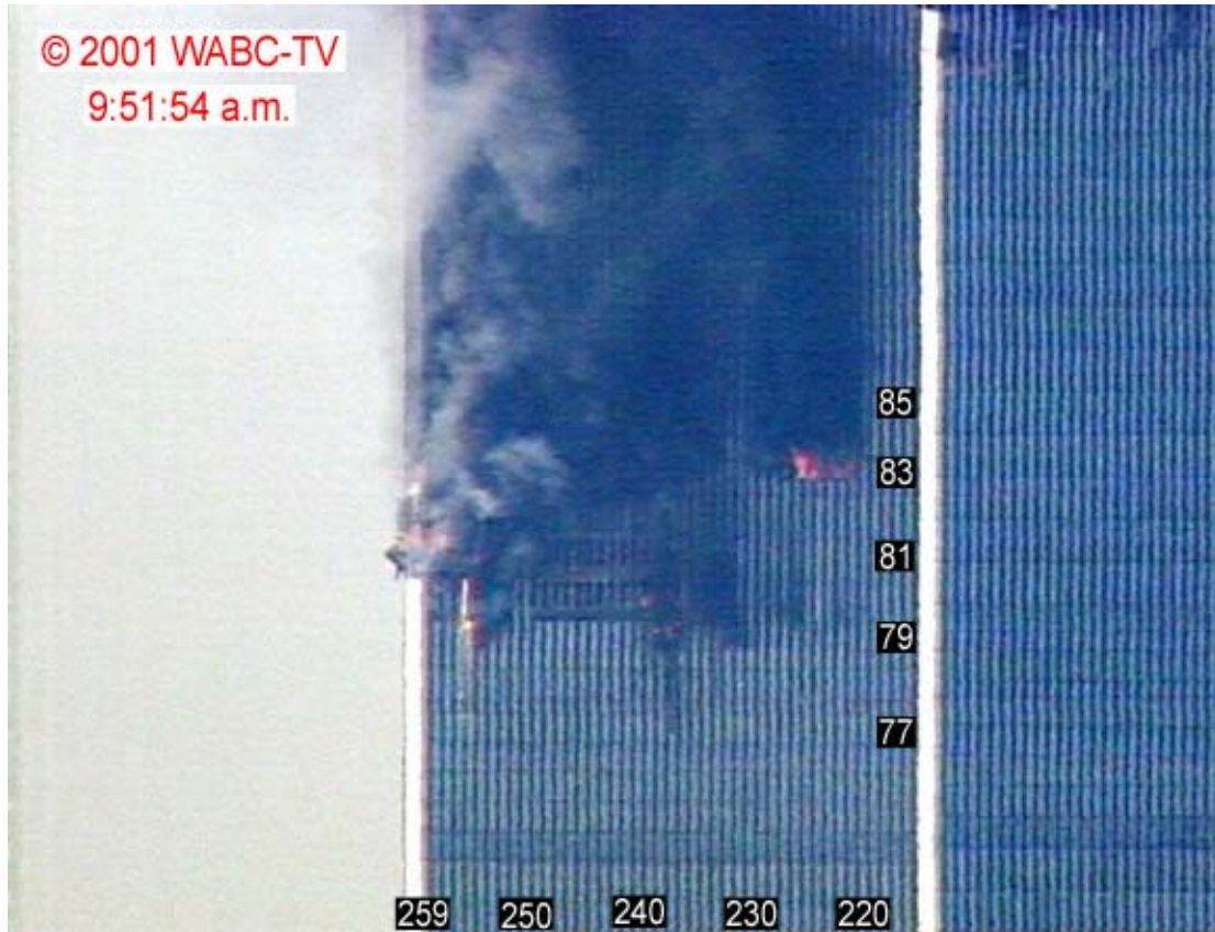
Figure 9-70. This image of the north faces of WTC 1 and WTC 2 was captured from a video recorded at 9:51:54 a.m. The intensity levels have been adjusted, and column and floor numbers have been added to WTC 2.
