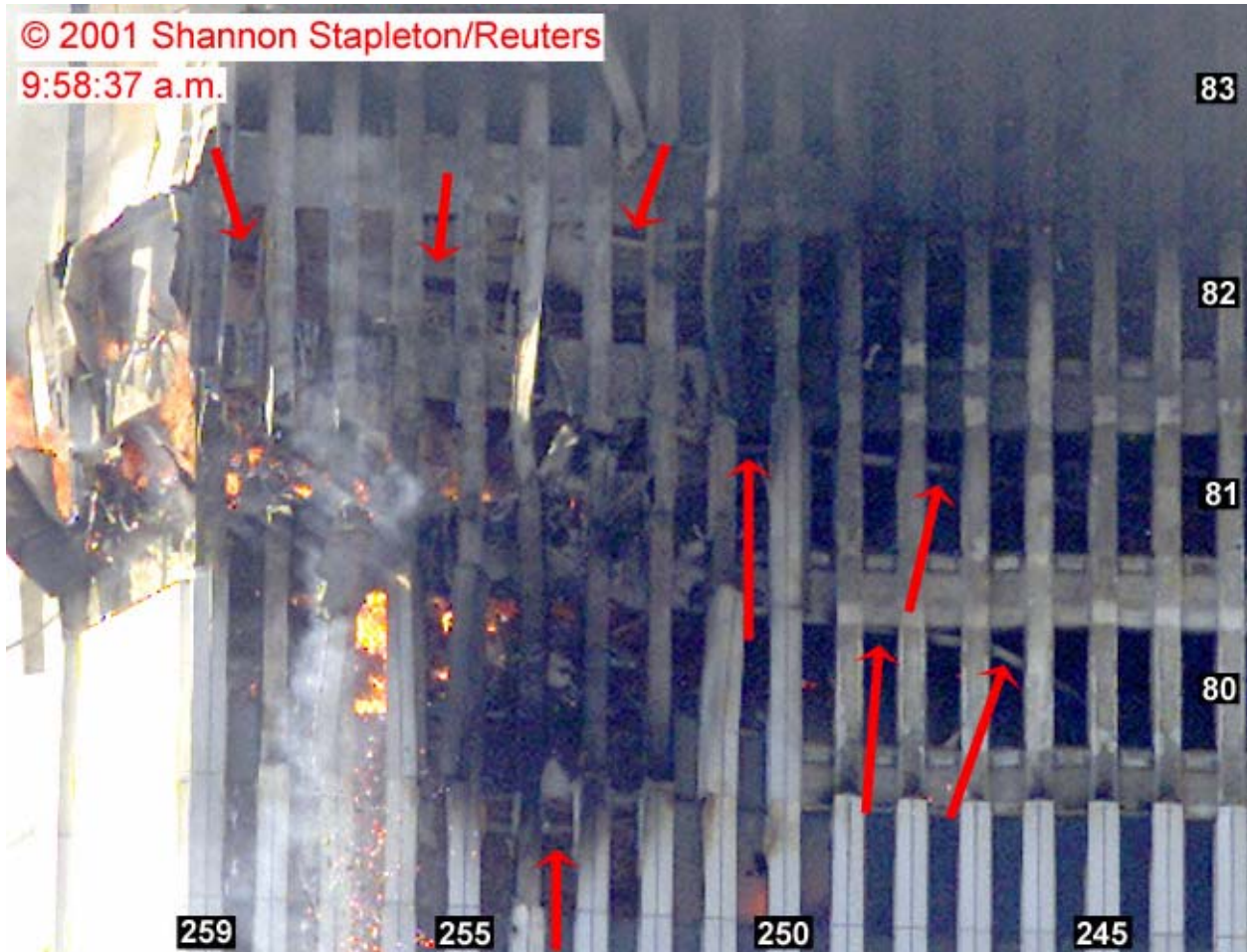
Figure 9-79. This photograph is a blow-up of a portion of the photograph shown in Figure 9–78. It shows the north face of WTC 2 and includes window 80-256 and part of the cold spot. The intensity levels of the original have been adjusted, and column and floor numbers have been added. Arrows highlight hanging objects visible through open windows on the 79th, 80th, 81st, and 82nd floors.
