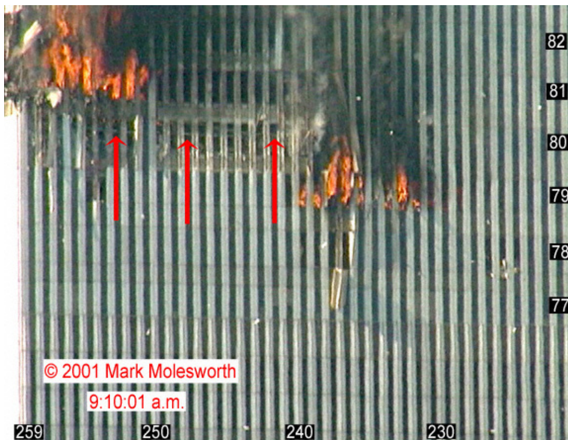
Figure 9-12. An image of the north face of WTC 2 captured from a video recording at 9:10:01 a.m. is shown. The intensity levels of the image have been adjusted, and column and floor numbers have been added. The arrows highlight hanging objects observed through open windows on the 80th floor.
