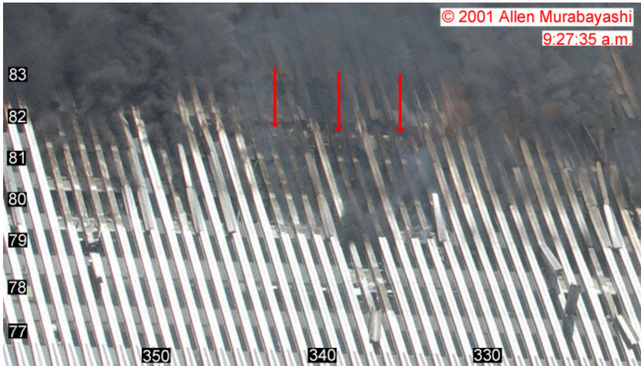
Figure 9-28. This cropped photograph shows the east face of WTC 2 at 9:27:35 a.m. The original image has been rotated, and column and floor numbers have been added. The arrows highlight a hanging object observed through open windows on the 82nd floor.
