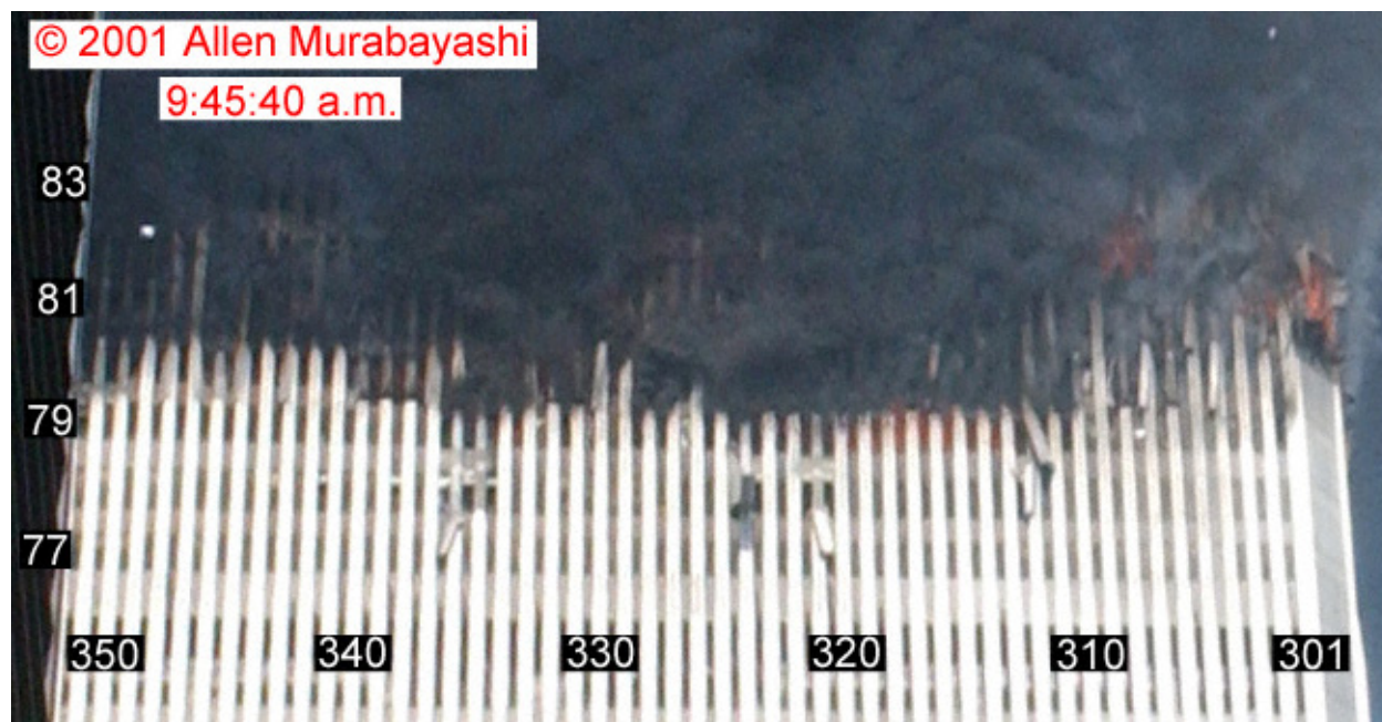
Figure 9-66. This cropped photograph shows the east face of WTC 2 at 9:45:40 a.m. The image has been rotated, and the intensity range has been adjusted. Column and floor numbers have been added.
