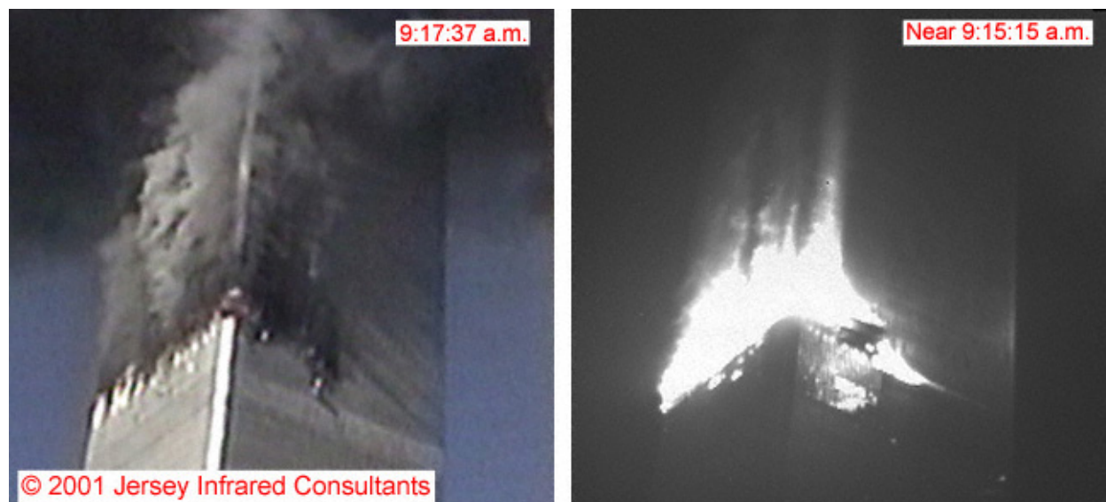
Figure 9-22. This figure compares an infrared photograph (on the right) and an image of WTC 2 captured from a video that was shot from the same vantage point and scaled and oriented to match the infrared shot. The north and east faces of the tower are visible. The video frame was shot at 9:17:37 a.m., and the infrared image was taken around 9:15:15 a.m. (an uncertainty of 15 s has been assigned).
