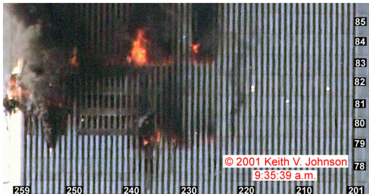
Figure 9-49. This cropped photograph shows the north face of WTC 2 at 9:35:39 a.m. The intensity levels have been adjusted, and column and floor numbers have been added.
