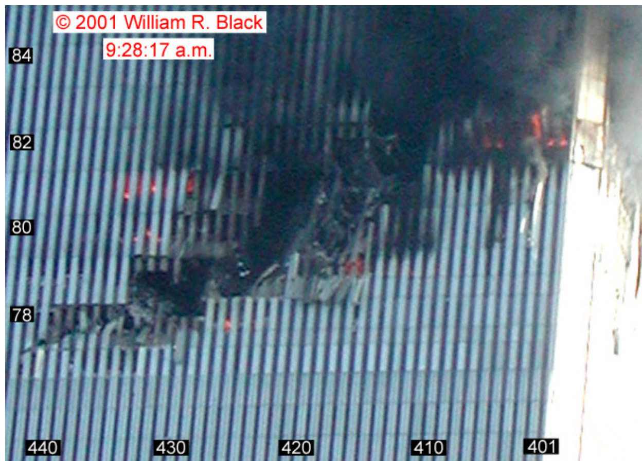
Figure 9-33. This cropped photograph showing the south face of WTC 2 was shot at 9:28:17 a.m. The image has been rotated, and the intensity levels have been adjusted. Column and floor numbers have been added.
