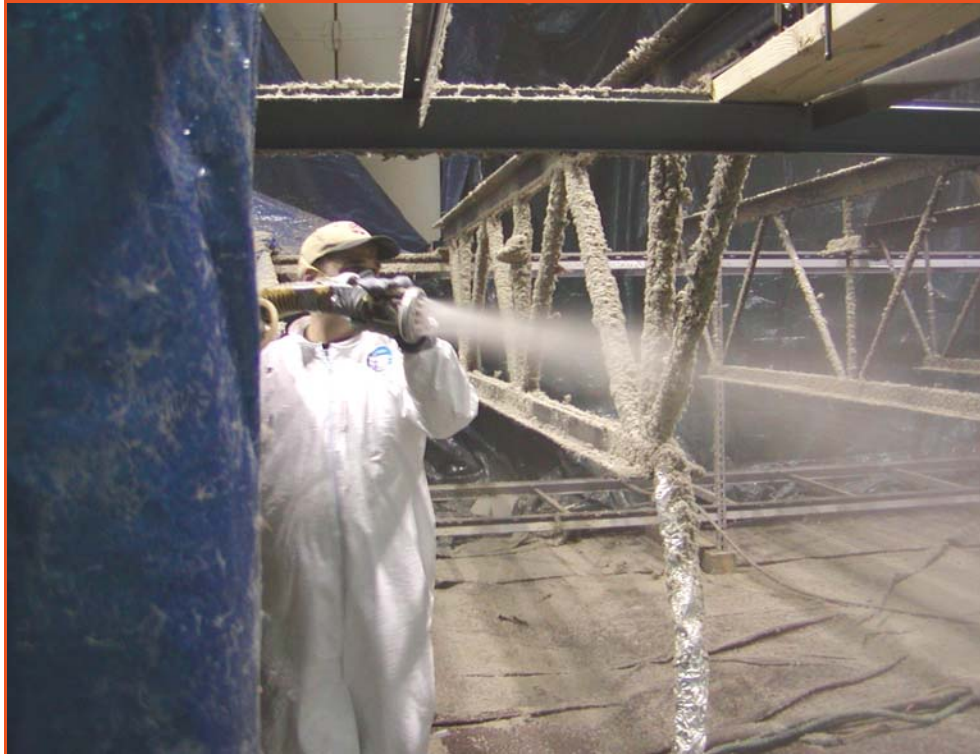
Figure 9–6d. Application of SFRM product to a truss.
