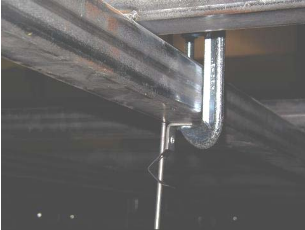
Figure 2–16. C-clamp and top CADDY fastener in suspension system 1.
