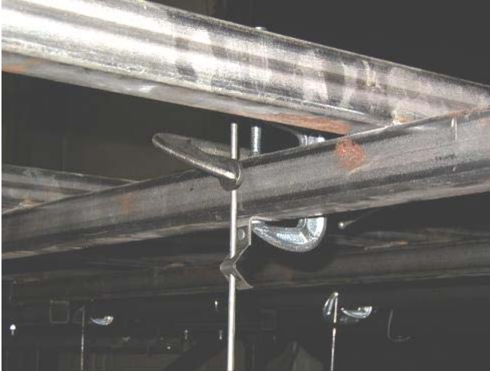
Figure 2–23. C-clamps and top CADDY clip in suspension system 2.
