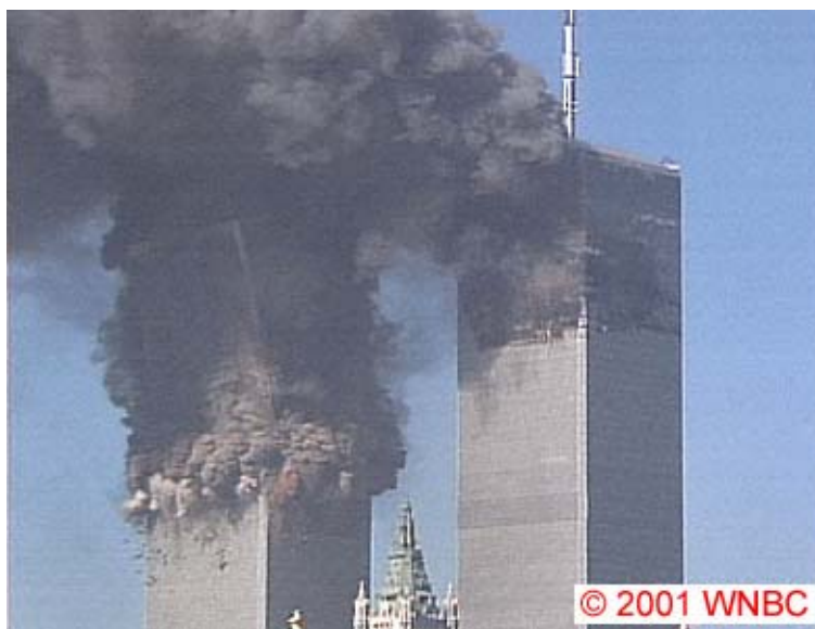
Figure E–8. View of upper building section of WTC 2 tilting to the east.
