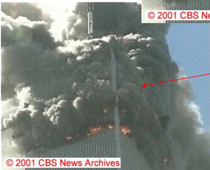
Figure 6–8. Smoke expulsion at Floor 98 from north and west faces as collapse initiates.
