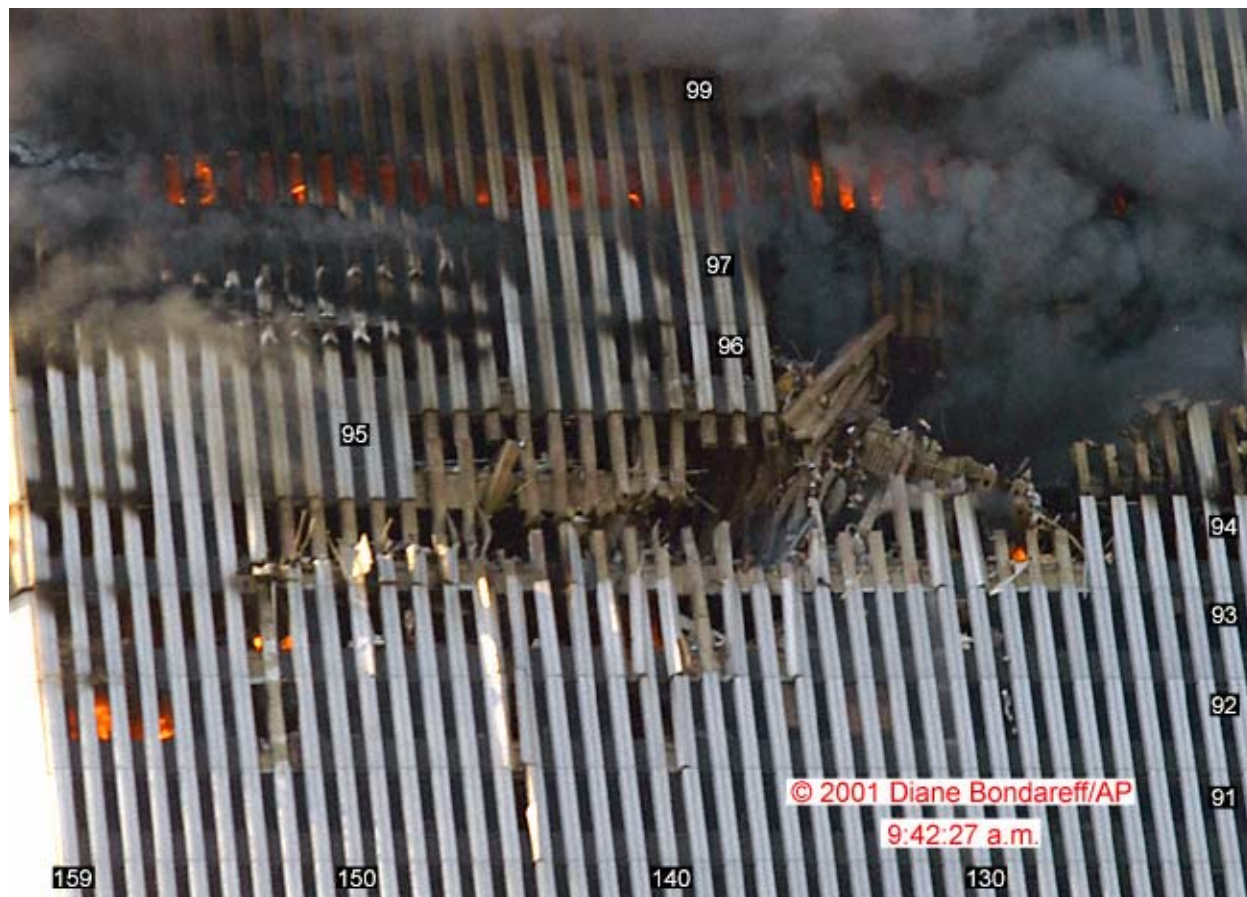
Figure 6–1. Initial aircraft impact damage on WTC 1 north face.
