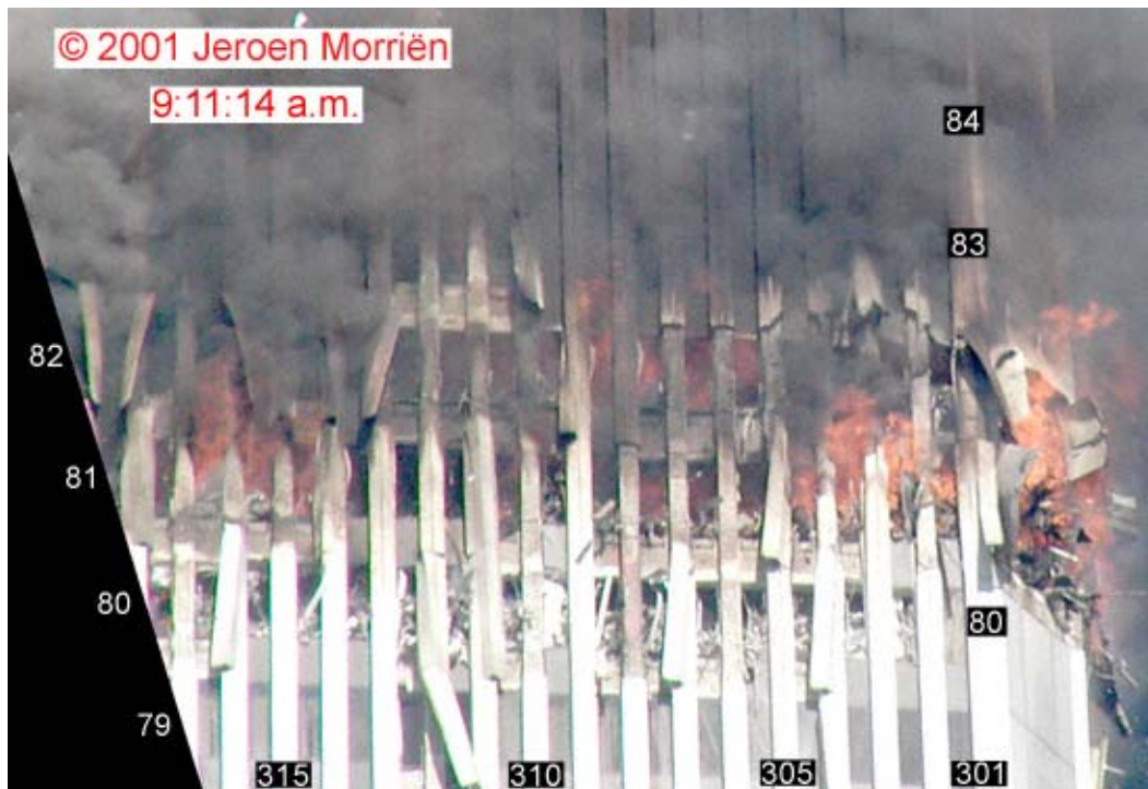
Figure 6–14. Debris piles at windows where fires are burning at the northeast corner.
