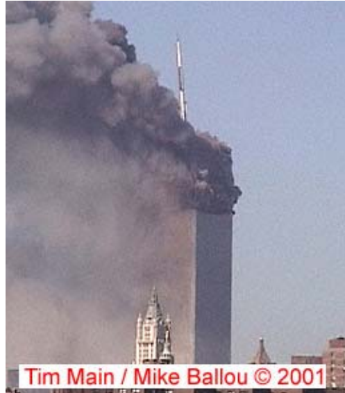
Figure E-6. WTC 1 building section above impact damage zone tilts to the south.
