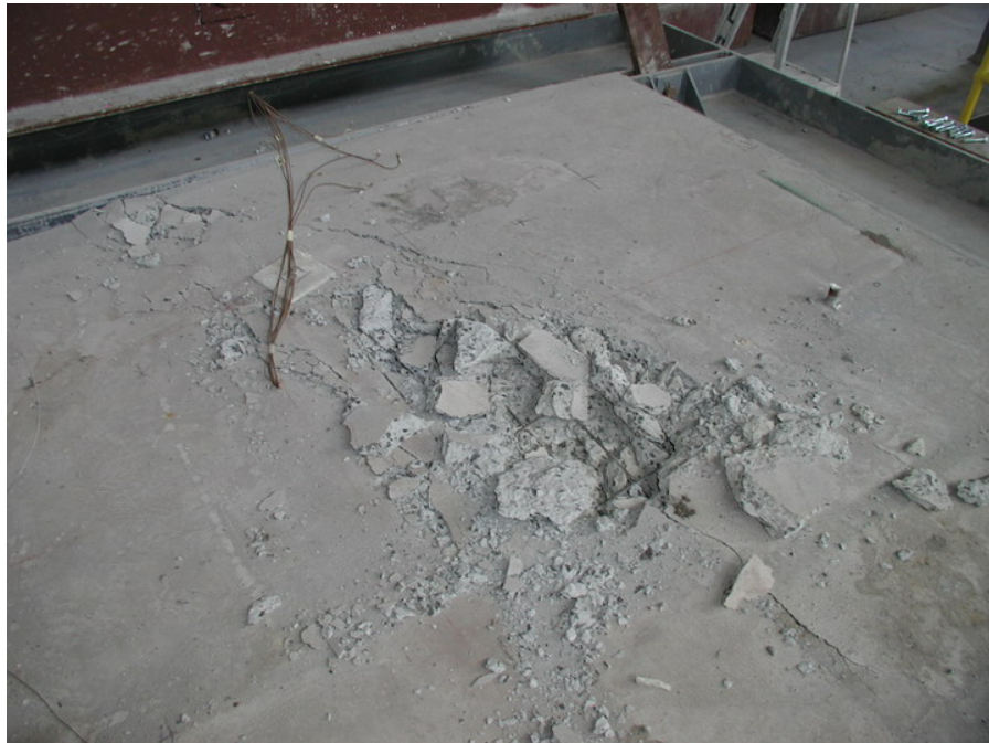
Figure 3–14. Detail of spalling concrete at east end of Assembly No. 1.
