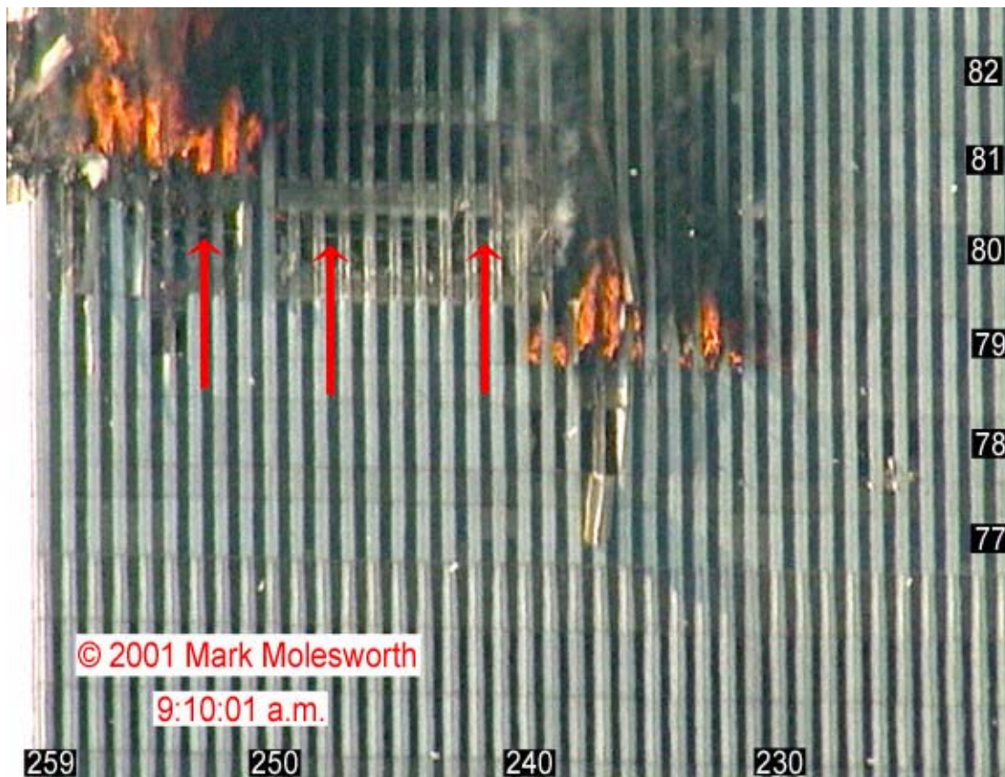
Figure 6–15. Hanging object (noted by arrows) in north windows of Floor 79 appears to be edge of Floor 80.
