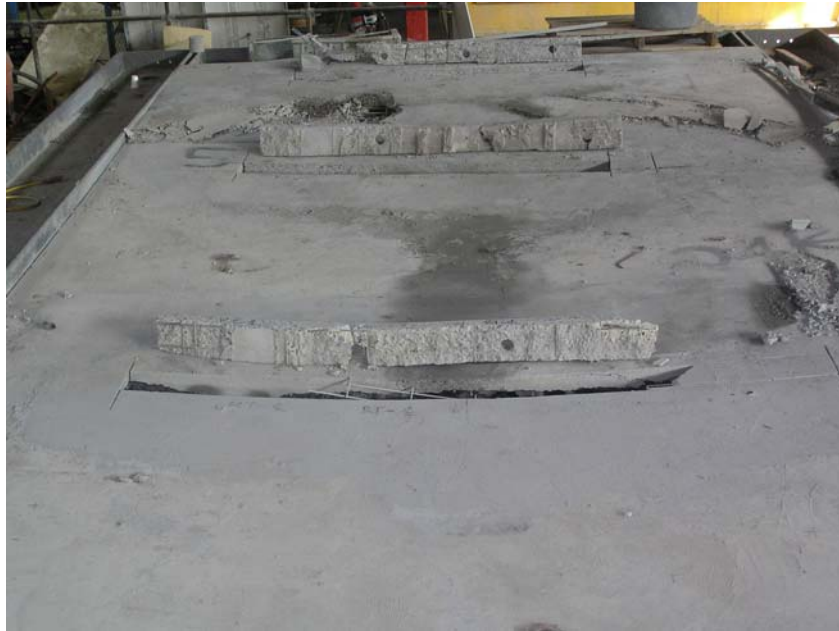
Figure 3–12. Sections cut through concrete slab to confirm extent and depth of spalling.
