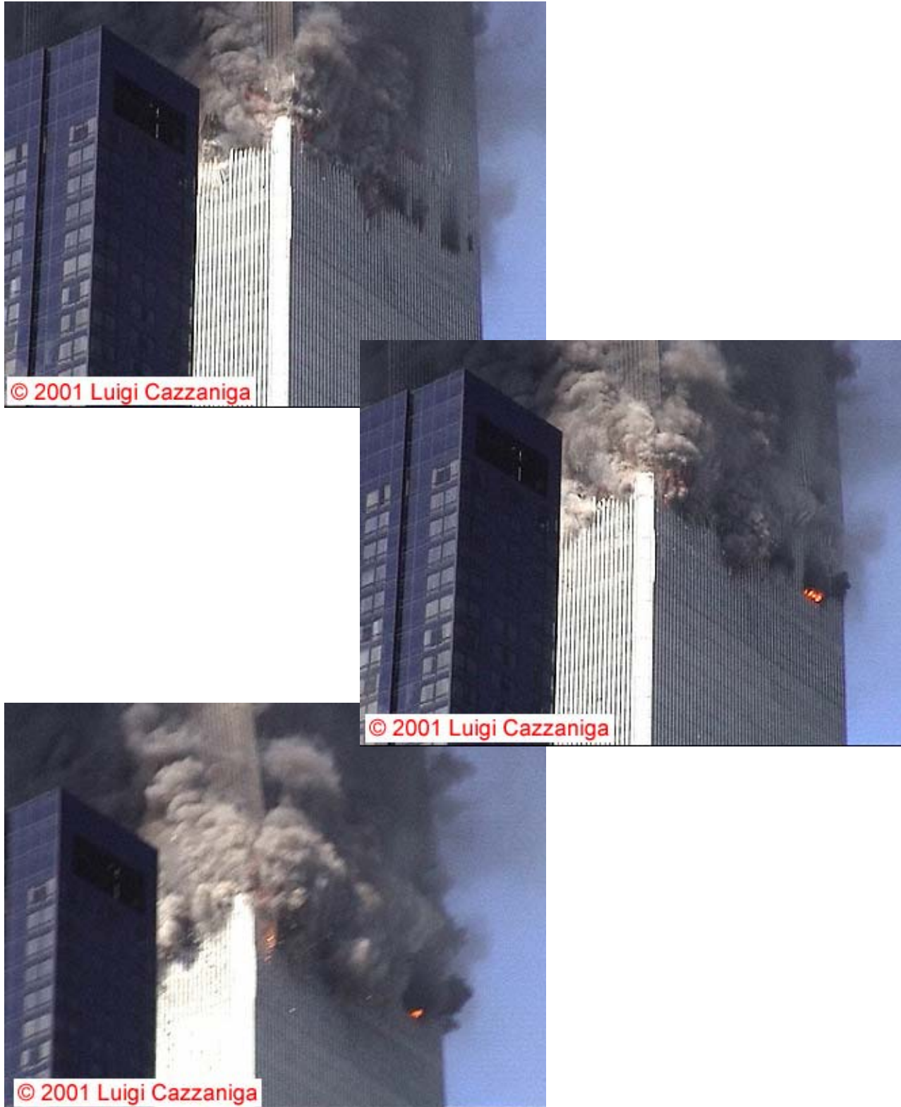
Figure 6–22. View of WTC 2 buckling of east wall near northeast corner as collapse initiates from northeast.
