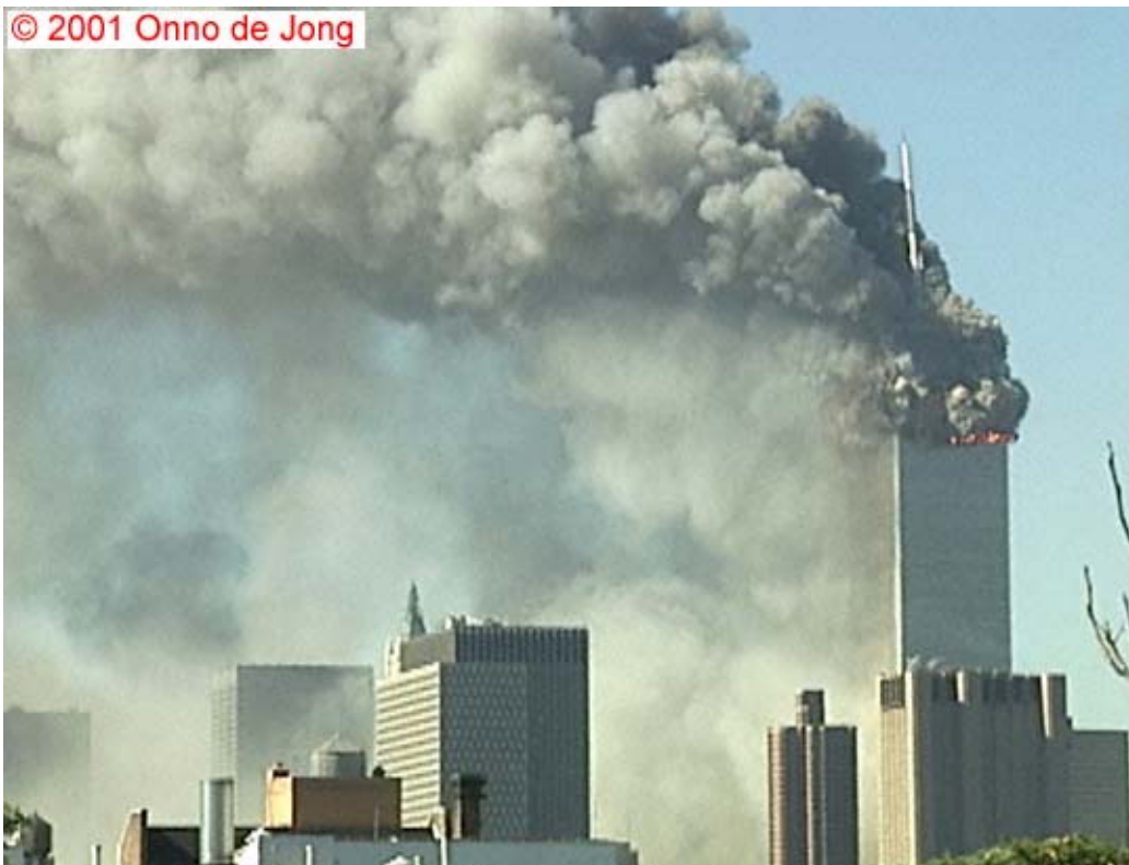
Figure 6–9. Smoke expulsion at Floor 98 from north and east faces at collapse initiation.
