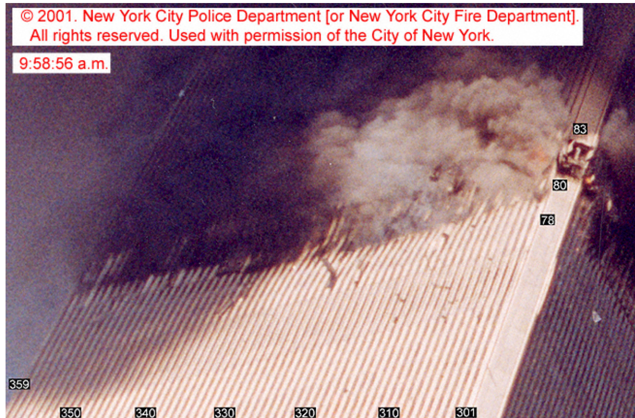
Figure 6–21. WTC 2 exterior columns bowing inward across the east face between Floors 77 and 83 at 9:58:55 a.m.
