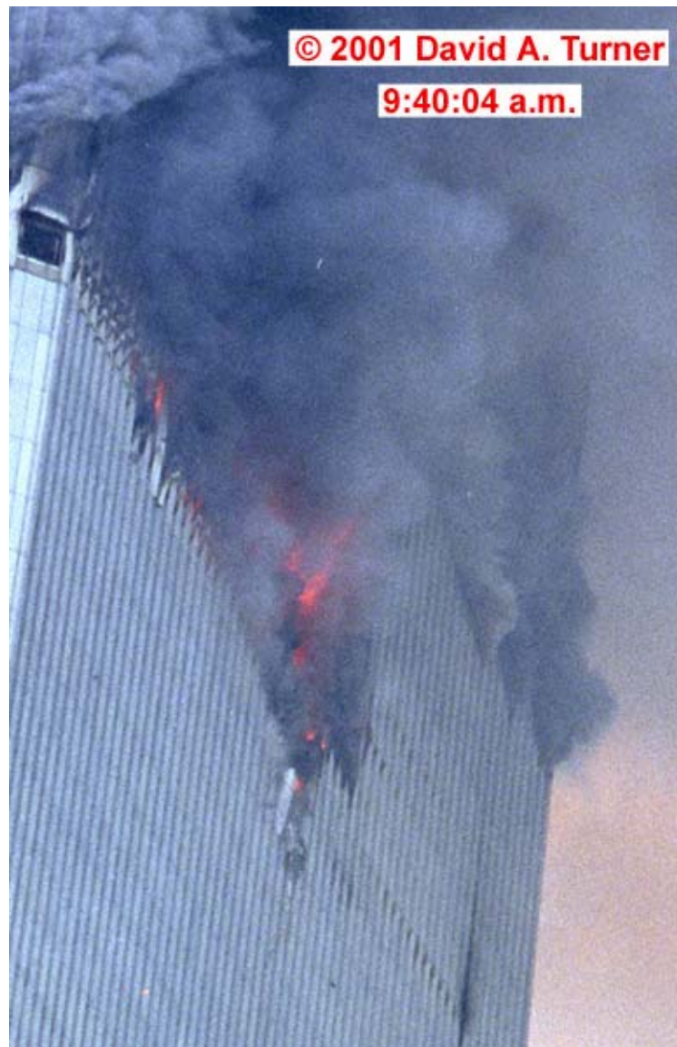
Figure 6–5. Fires on WTC 1 south face at 9:40 a.m. Note lack of inward bowing.
