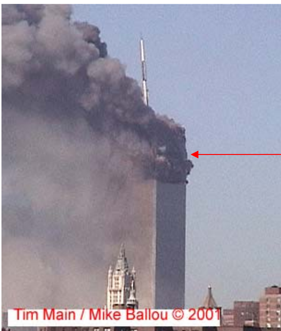
Figure 6–7. Expulsion of smoke and debris at WTC 1 Floor 98 on the east, north, and west faces.
