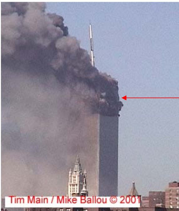
Figure 9–13. Expulsion of smoke and debris at WTC 1 Floor 98 on the east, north, and west faces.
