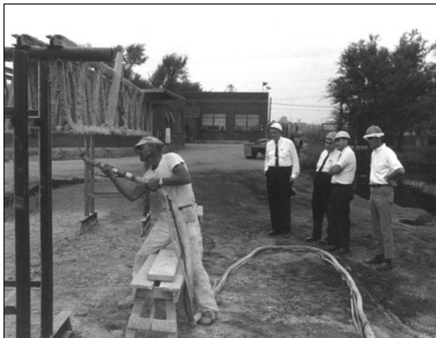
Figure 2–2. Demonstration of application of Monokote sprayed fire-resistive material to floor trusses.
