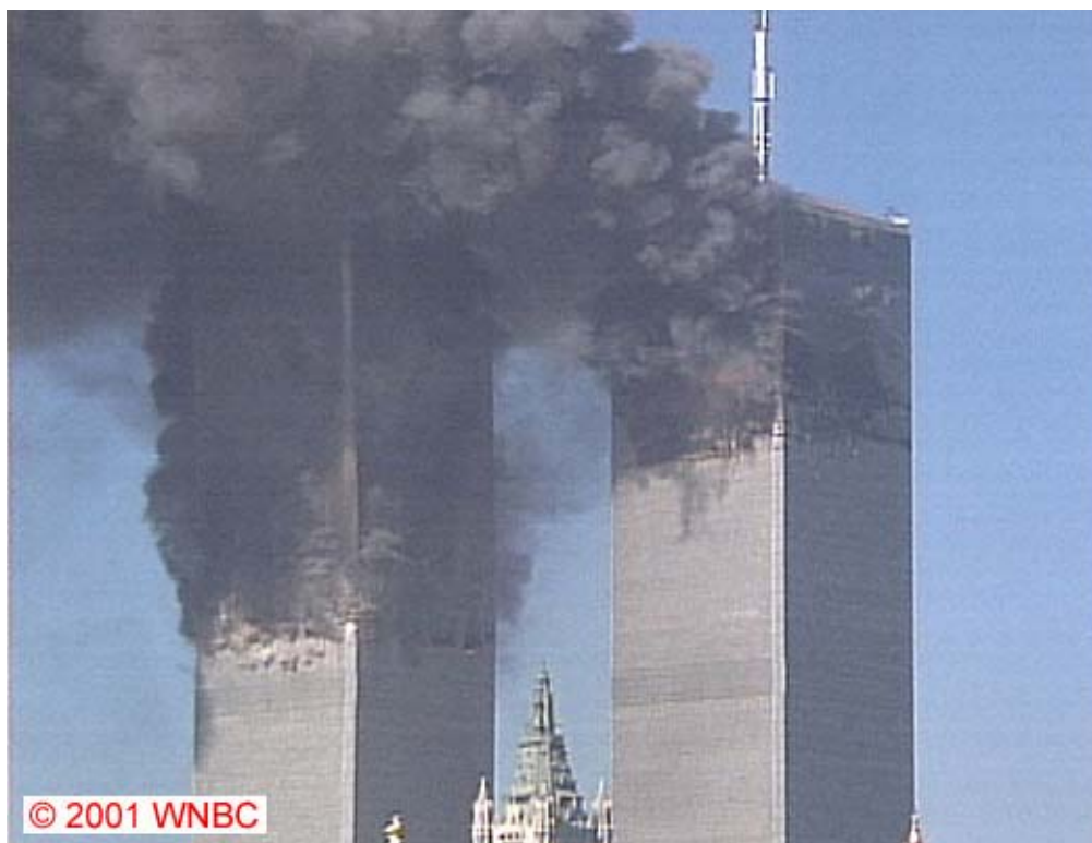
Figure 5–16. Initiation of Collapse of WTC 2. Note the tilt toward east and south.
