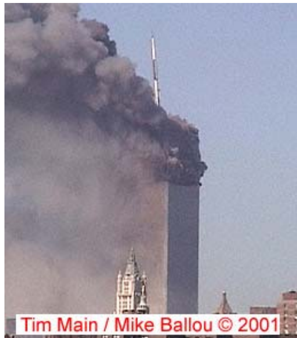
Figure 5–8. Collapse initiation and tilting of WTC 1 (view from the northeast).
