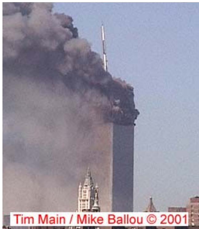
Figure E–11. Collapse initiation and tilting of WTC 1 (view from the northeast).
