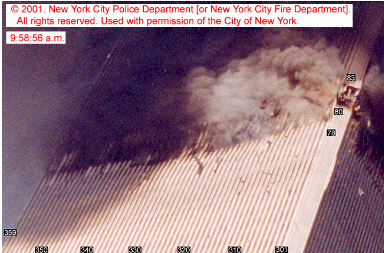
Figure E-14. Inward bowing of exterior columns of the west wall of WTC 2 just before collapse.
