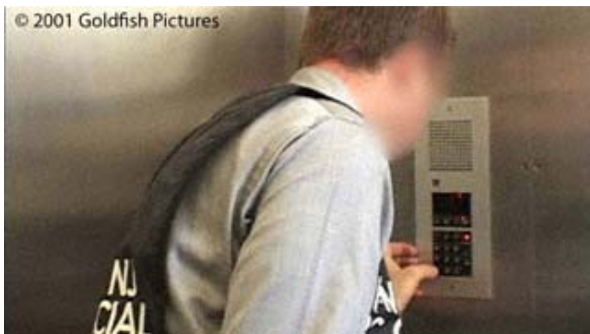
Figure 2–16. Elevator communication panel in the fire command station of WTC 1, as operated on September 11, 2001.
