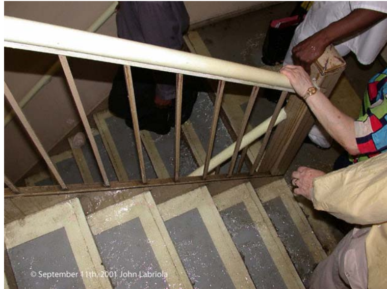
Figure 2–10. 44 in. stairwell in WTC 1 taken on September 11, 2001.
