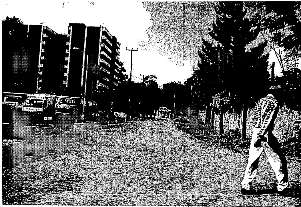
The approach to the Nairobi embassy as of December 1998 (author's photo)
