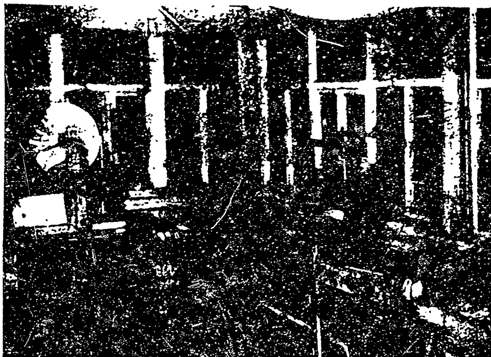
Corner of the workshop of K. E. Tsiolkovsky on the glassed in porch of the old house. In the center is a combined carpenter's work bench, serving in case of need and as a metal-working bench. On it there stands a small crimping machine; on the left on the small table is an electrical machine.
