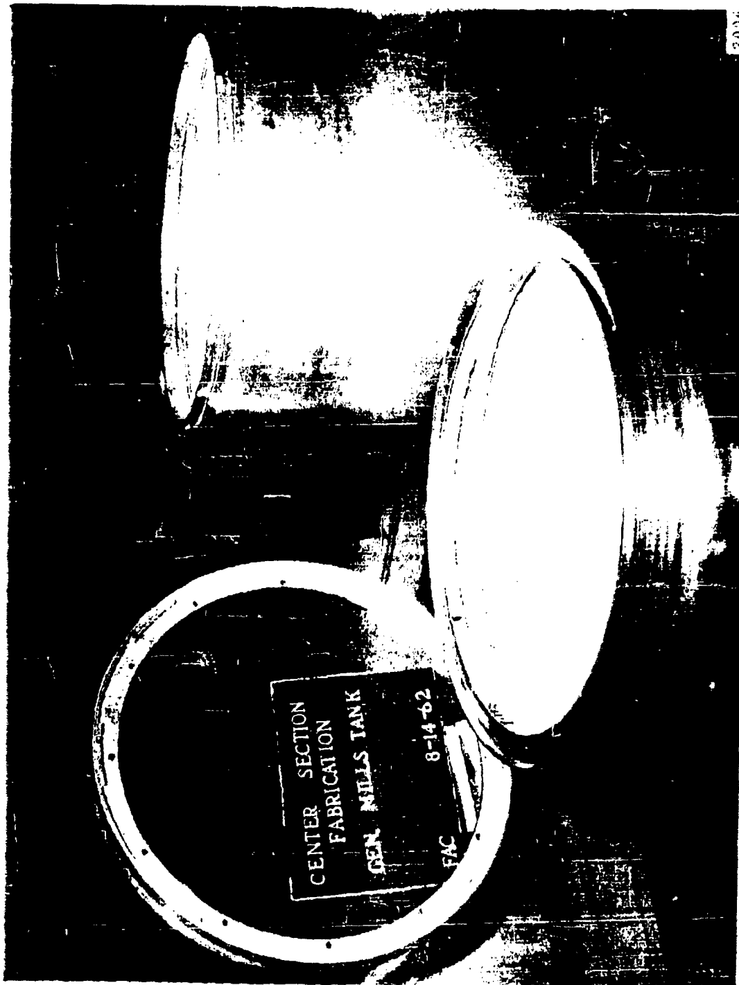
Figure 6.3 Bayonet Rings on Center and Tail Sections
