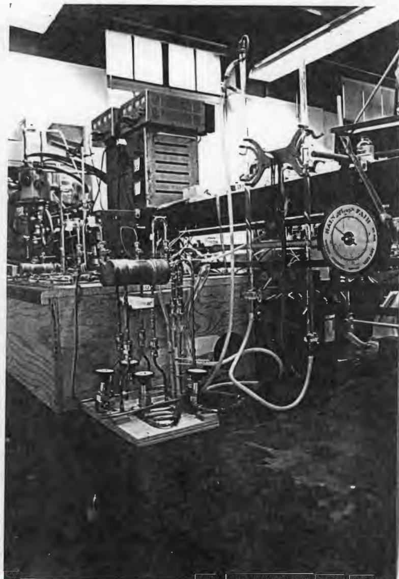
**LEFT:** View looking down on water bath, copper sample flasks and gas manifold valves in foreground, data acquisition system in background behind another sample flask.
