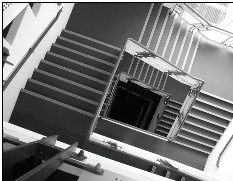
**Figure 7-42. Enclosed stairwell (large gap)**
