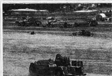
(U) 37 earth movers worked two shifts seven days per week for five months moving 3.2 Million cubic yards of earth
