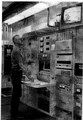
Figure 1. Weapons are tested at DOE's Pantex Plant in Amarillo, TX. Sandia-designed test systems provide physical and electrical stimuli to a weapon and record its response. In this case, a centrifuge provides acceleration environments a warhead would experience during missile flight (above). The test is controlled and response measured at the test system console (below).
