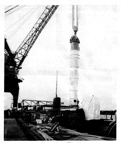
Figure 1. For as long as they are in the active stockpile, weapons are sampled periodically and returned to DOE facilities for extensive evaluation. Here, a development exercise shows a Trident II missile being removed from the USS Tennessee.
