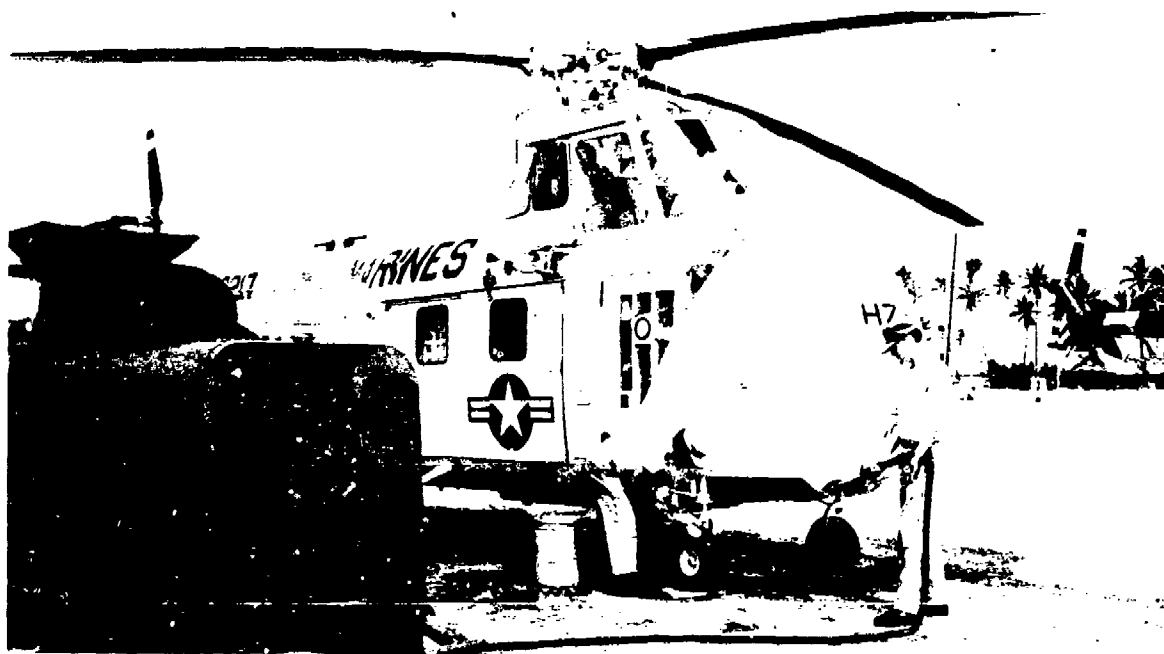
Figure 29. Scrubbing helicopter to remove contamination, REDWING.
