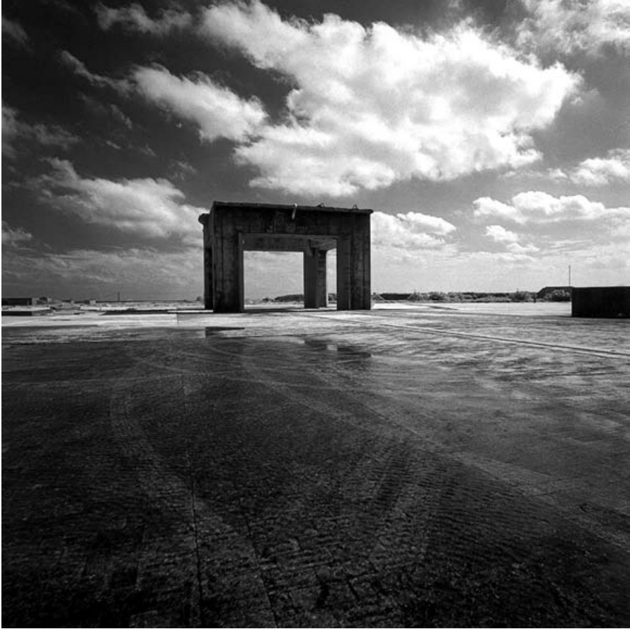
Saturn Apollo Launch Complex 34, Cape Canaveral Air Force Station: October 1999. (©Scott Andrews)
