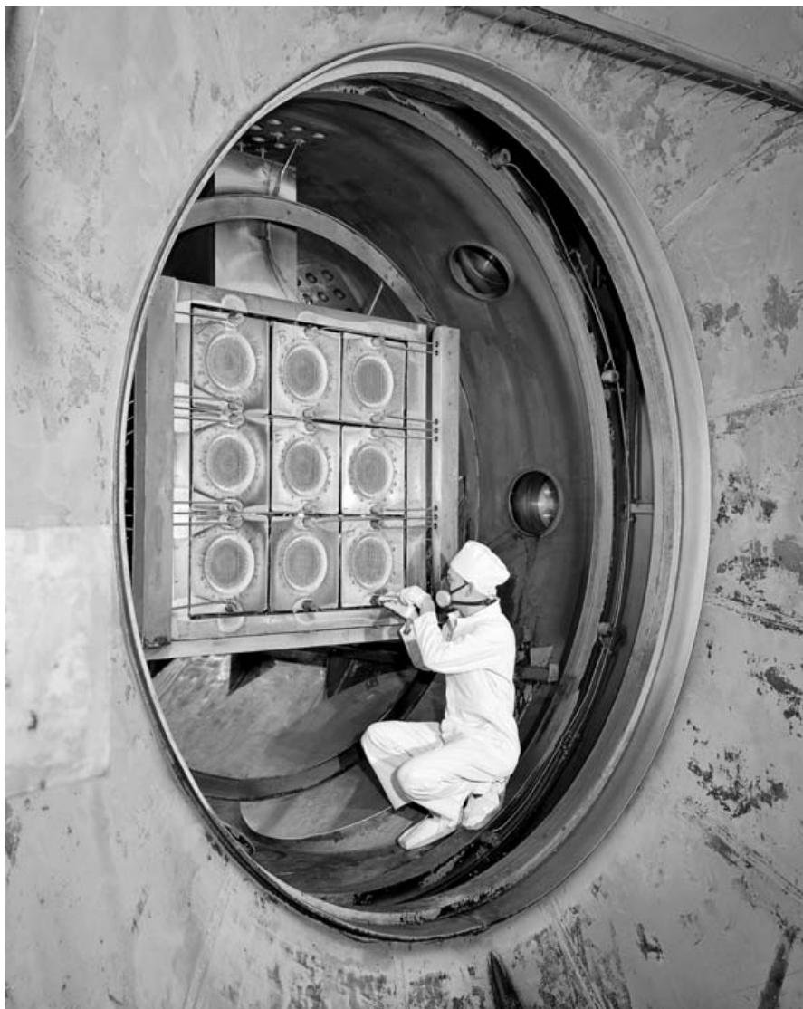
1964: Engineer at a 9 thruster ion engine array. (NASA)
