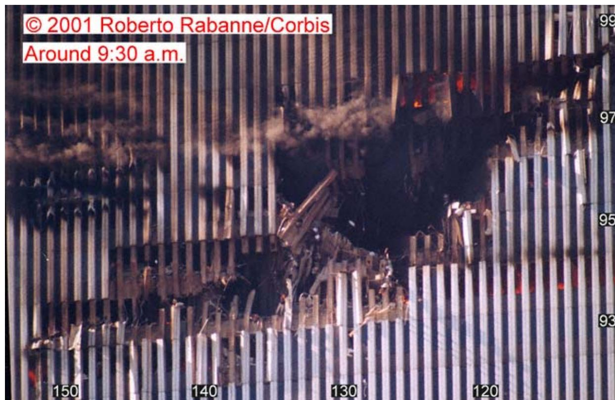
**Figure 2–2. Photograph of the north face of WTC 1 around 9:30 a.m. showing the area damaged by the aircraft strike.**
