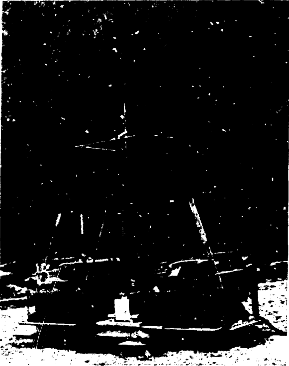
Fig. 4. Modular Subterrene field demonstration unit melting drain holes at Sandelier National Monument.
