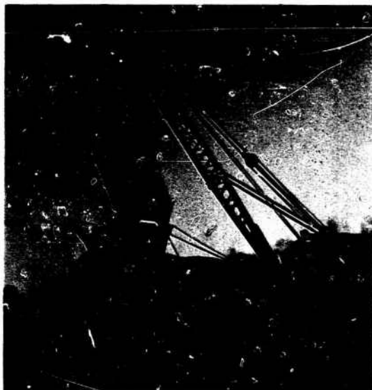
Snow being poured through a specially constructed metal chute into 25,000-gallon tank.
