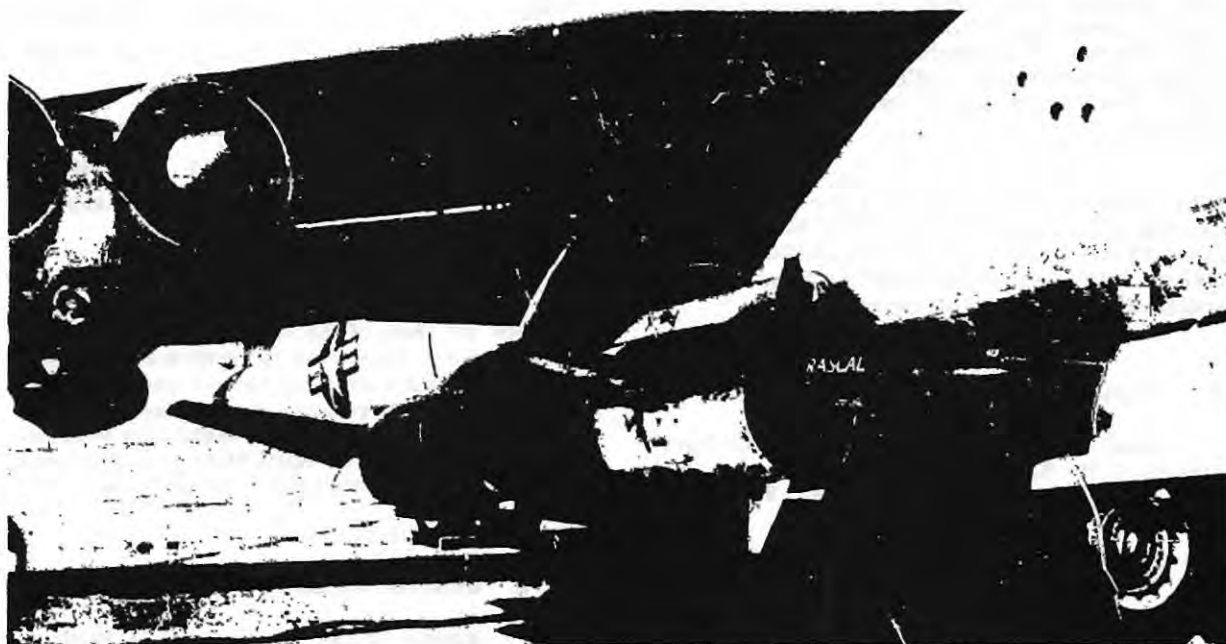
Figure 5. GAM-63A Mounted on the DB-47 Director Aircraft
