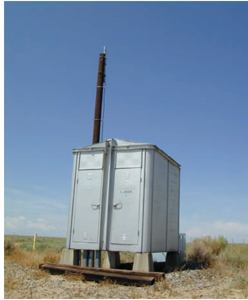
Figure 6-3. Typical Block Signal Control Equipment Enclosure
