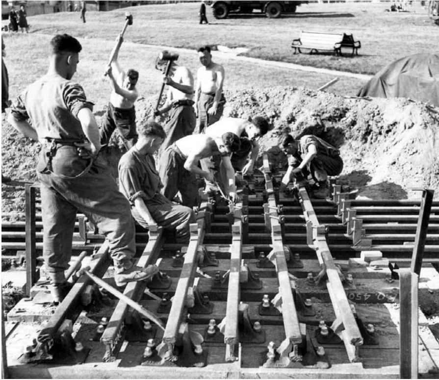
Figure 10: Pile mattress. The British emplaced their heavy (3.7 inch) guns on a solid base that became known as a “Pile mattress.” (Reprinted from Imperial War Museum.)
