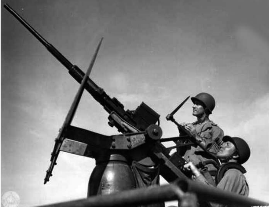
Figure 31. USN 20 mm gun. The Navy's 20 mm guns accounted for one-third of the Japanese aircraft claimed by ship guns prior to September 1944, and one-quarter of the claims after that date. (Reprinted from http://www.bcoy1cph.pacdat.net/20mm_Oerlikon_AA_USN..jpg .)
