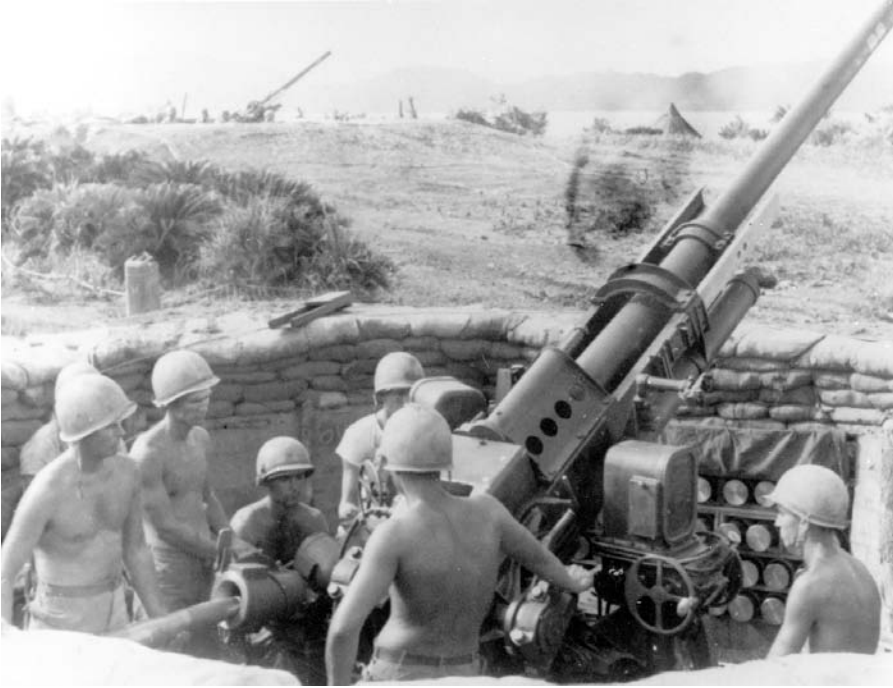
Figure 13. US 90 mm M-1 gun. The standard US heavy anti-aircraft gun during World War II was the 90 mm M-1. (Reprinted from US Army Air Defense Artillery Museum.)
